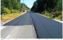
This photo of a repaving project shows the original road surface (lower left), the interlayer (upper left), and the new pavement surface (right).
