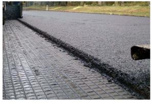
(c) Geocomposites (<u>www.ramalho1.com</u>) Figure A-3. Reinforcement of asphalt overlays.
