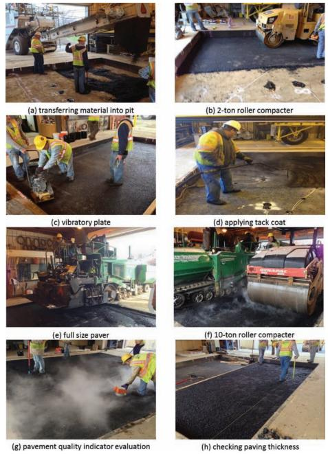
Figure 3.11 Asphalt concrete layer construction.
