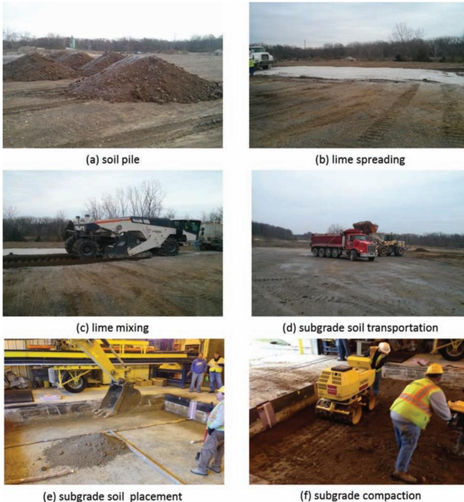
**Figure 3.8** Subgrade construction.
