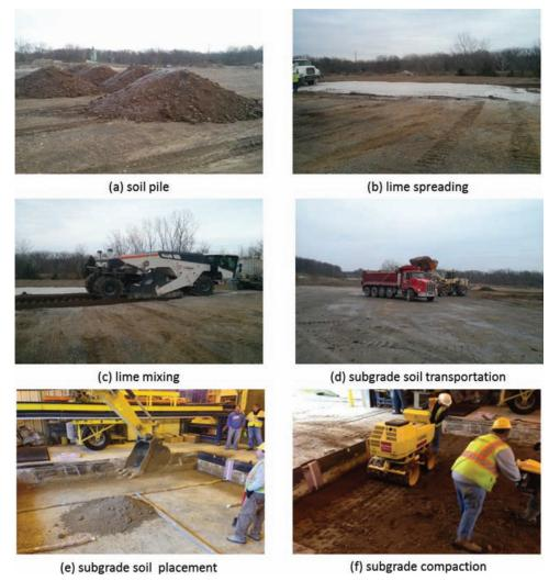
Figure 3.8 Subgrade construction.
