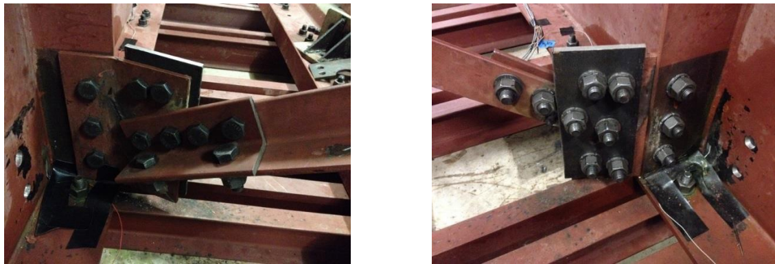
Figure 3-5: Crossframe after re-welding and repair
