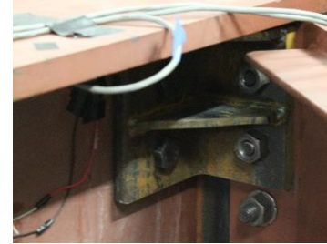
(c) Retrofit angle at top web-gap
