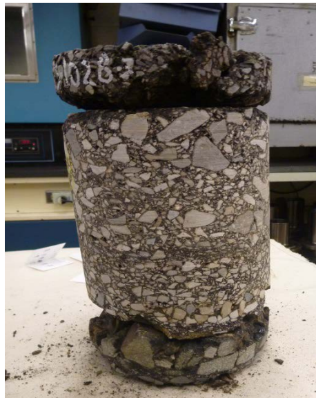
Figure 6. Cores Indicated Debonding and Stripping in Site Q (US 11 in Montgomery County)
