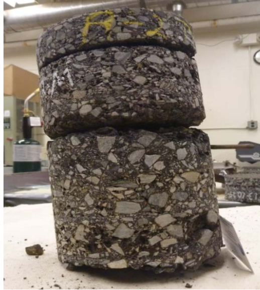
Figure 7. Delaminated Pavement Layers Found in Site R (US 221 in Floyd County)
