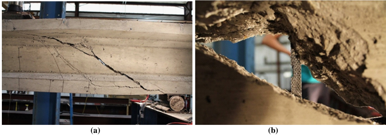
Figure 64. (a) Unloaded Shear Failure of Specimen 5 with Minimum NEFMAC Reinforcement, and (b) Frayed NEFMAC grid within the Shear Failure Crack
