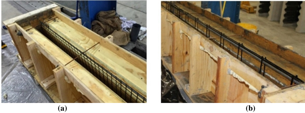
Figure 17. Completed Beam Formwork with (a) C-Grid and (b) NEFMAC Grid
