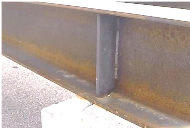
Figure 3.8 Visual Weld Inspection on the Small Bridge, E004
