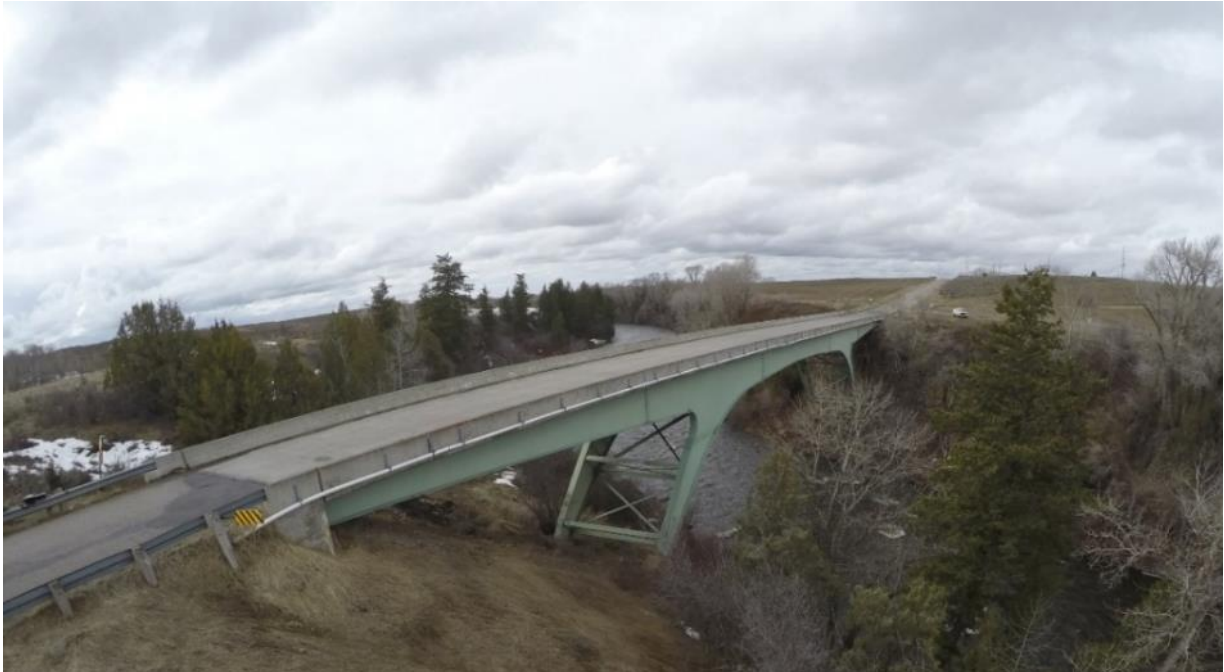
Figure 5.5 Northern Girder of the Fall River Bridge.
