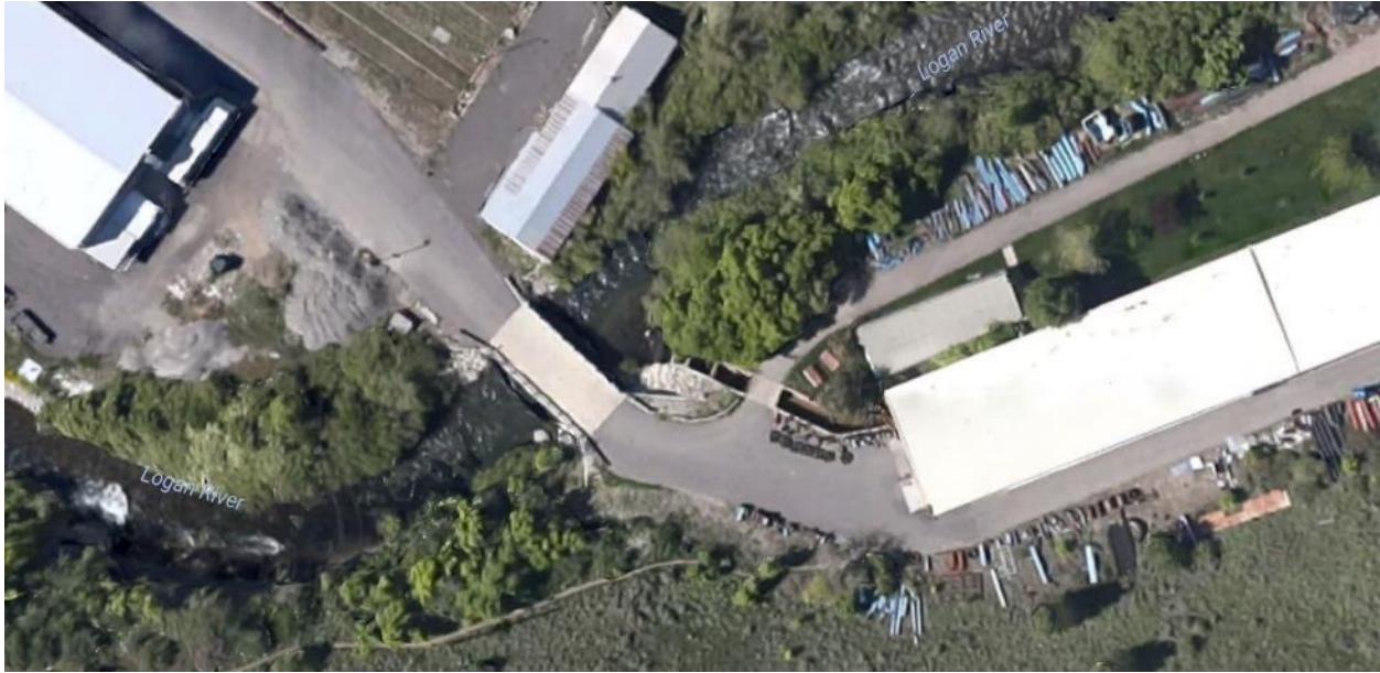
Figure 4.10 The UWRL Bridge
