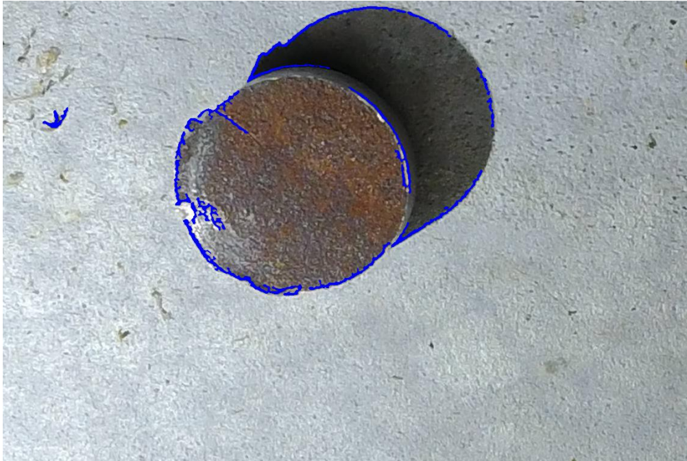
Figure 4.20 The Detected Crack Using Image Processing Techniques on the UWRL Image (Laplacian of Gaussian), E014
