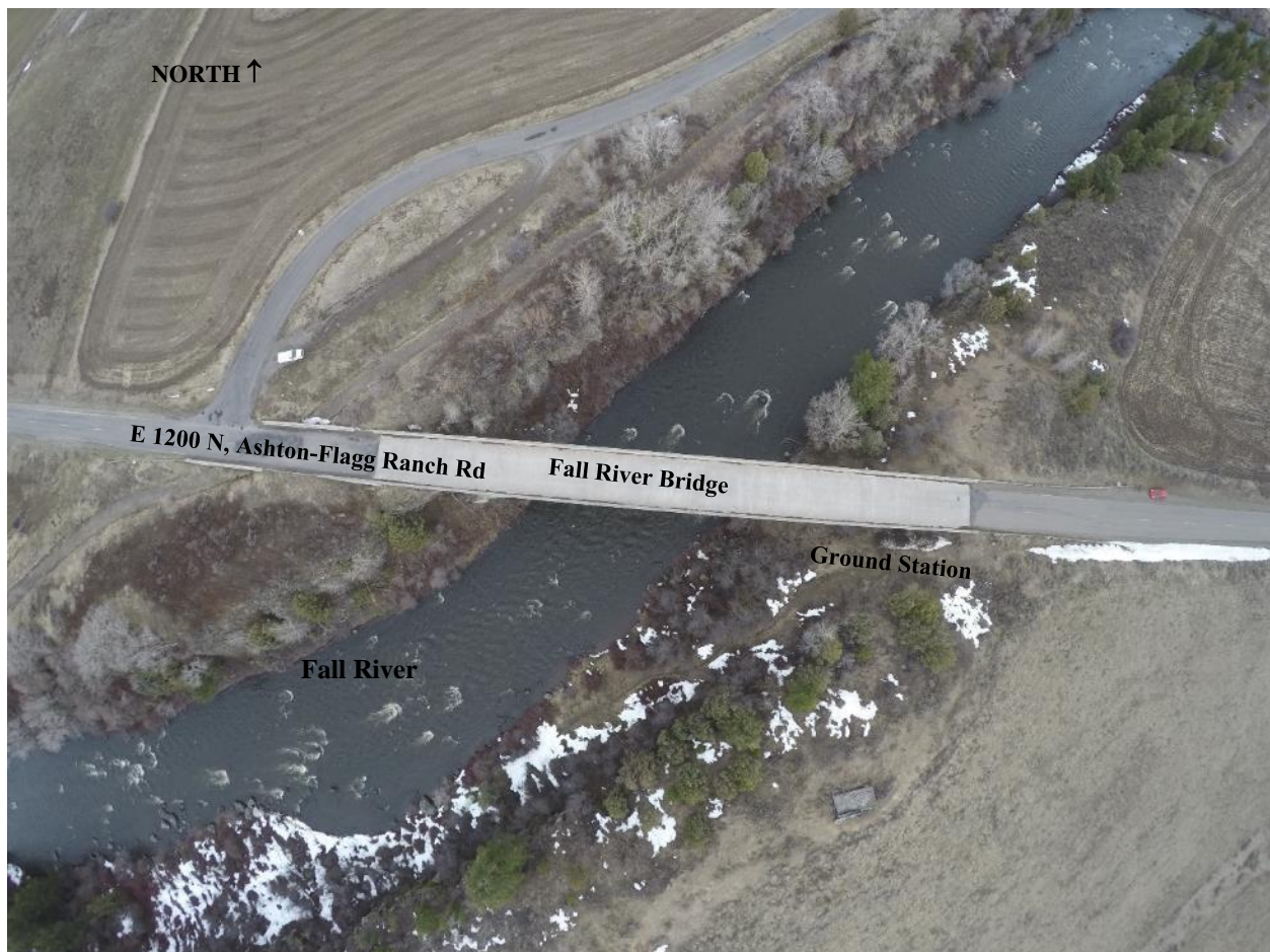
Figure 5.1 Aerial Image Captured by 3DR Solo (Courtesy of Dan Robinson)
