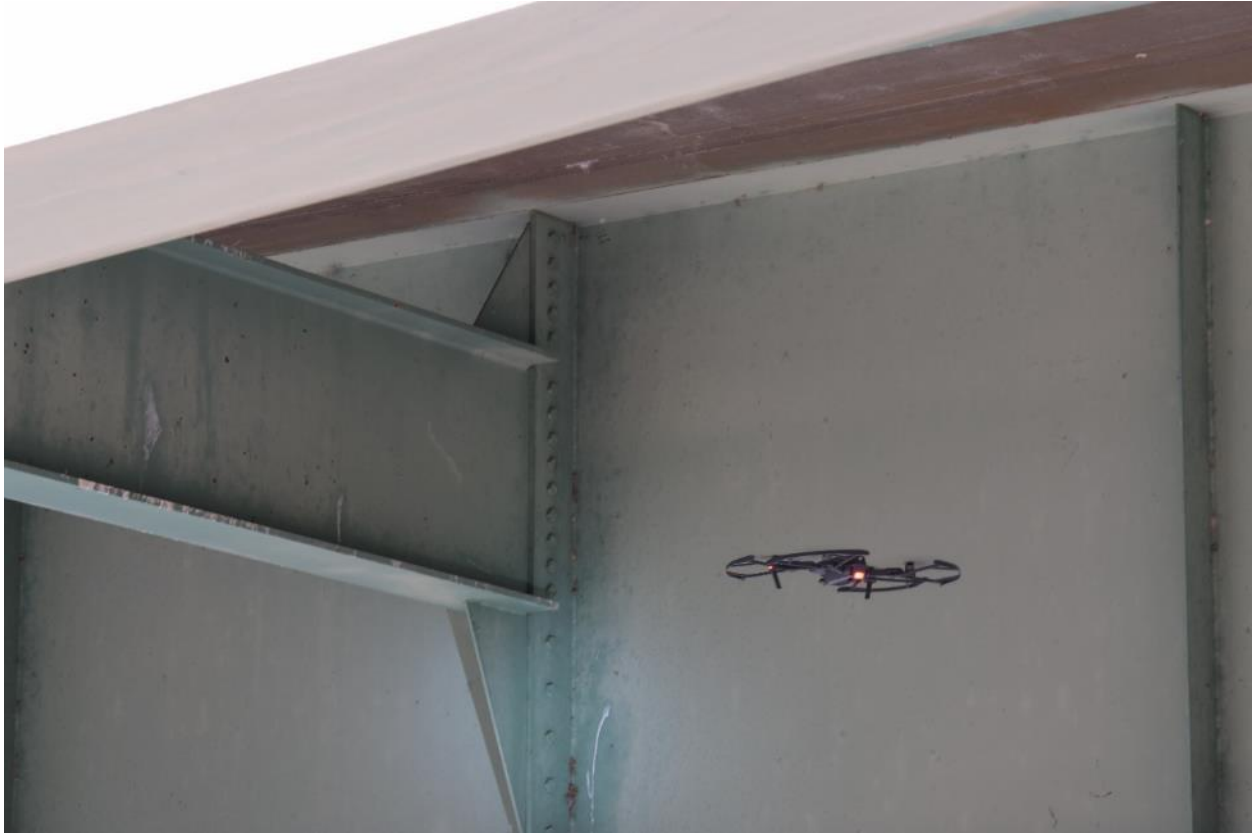
Figure 5.7 UAS Flying Under the Bridge.
