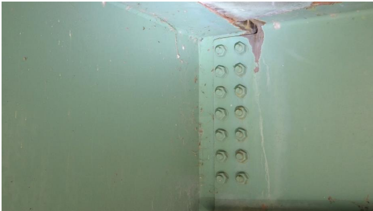
Figure 5.9 First Floor Beam on East, Northern Corner, No Noticeable Crack, E021
