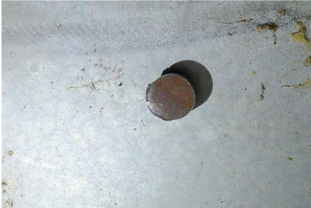
Figure 4.16 Photo of the Test-Piece Taken by DJI Mavic, UWRL Bridge, Bright Condition, Normal Camera Angle, E012
