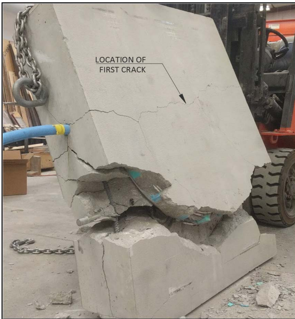
Figure 4.27 Third pad post failure
