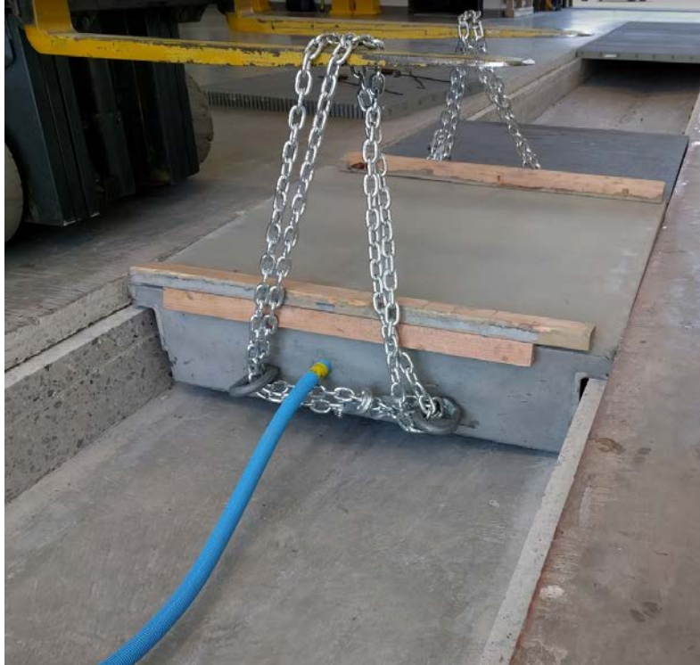
Figure 2.15 Installation of the first concrete embedded IPT coil
