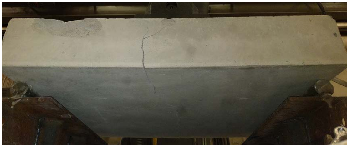
Figure 4.14 Crack 1/4 inch wide, load increased (32,000 cycles)
