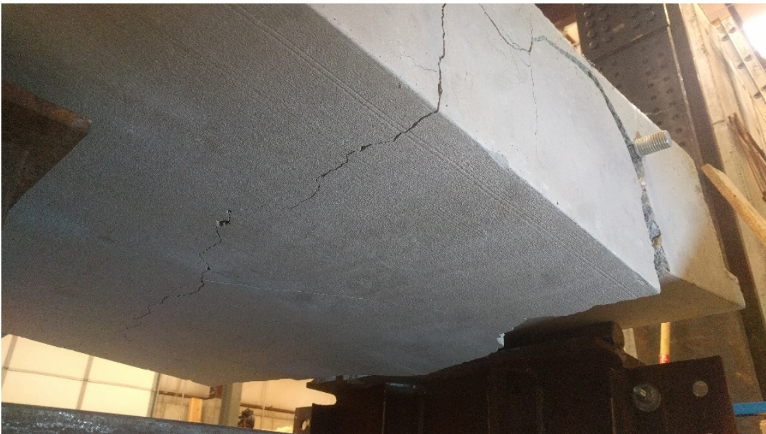
Figure 4.26 Pad after failure
