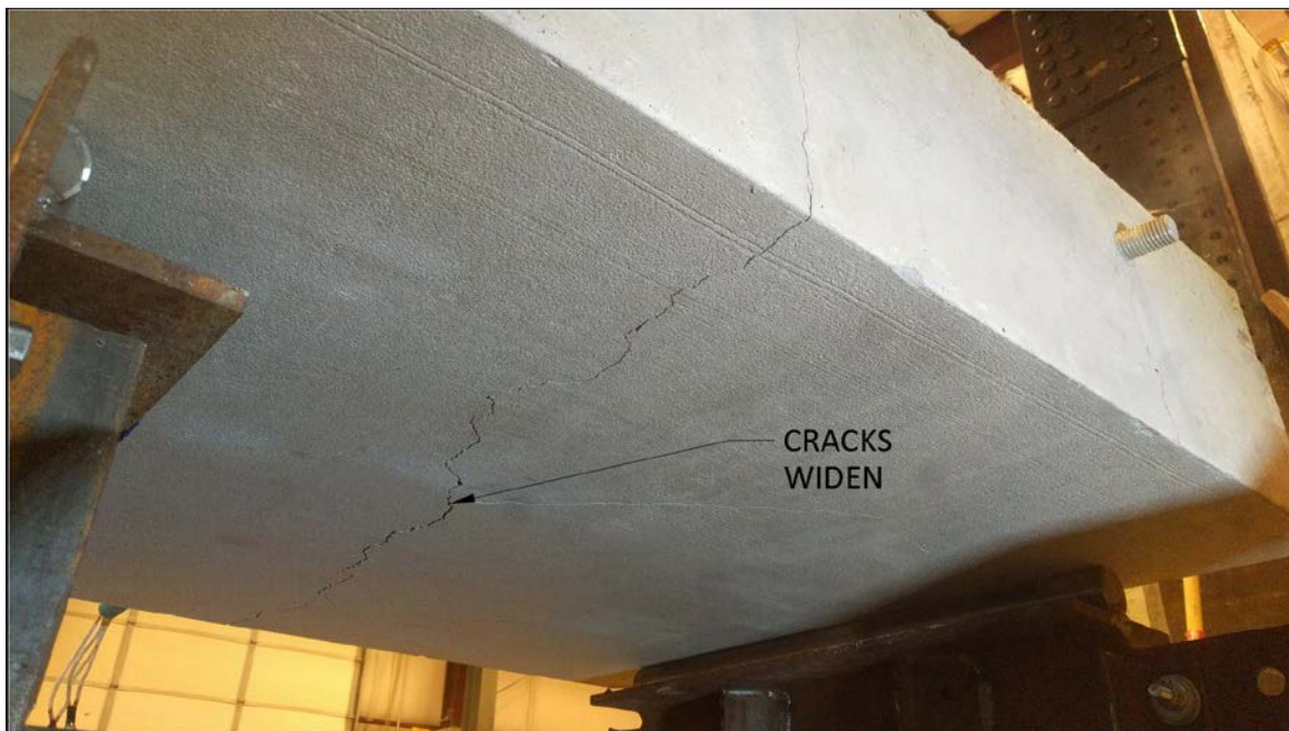
Figure 4.23 Crack 1/8 inch wide
