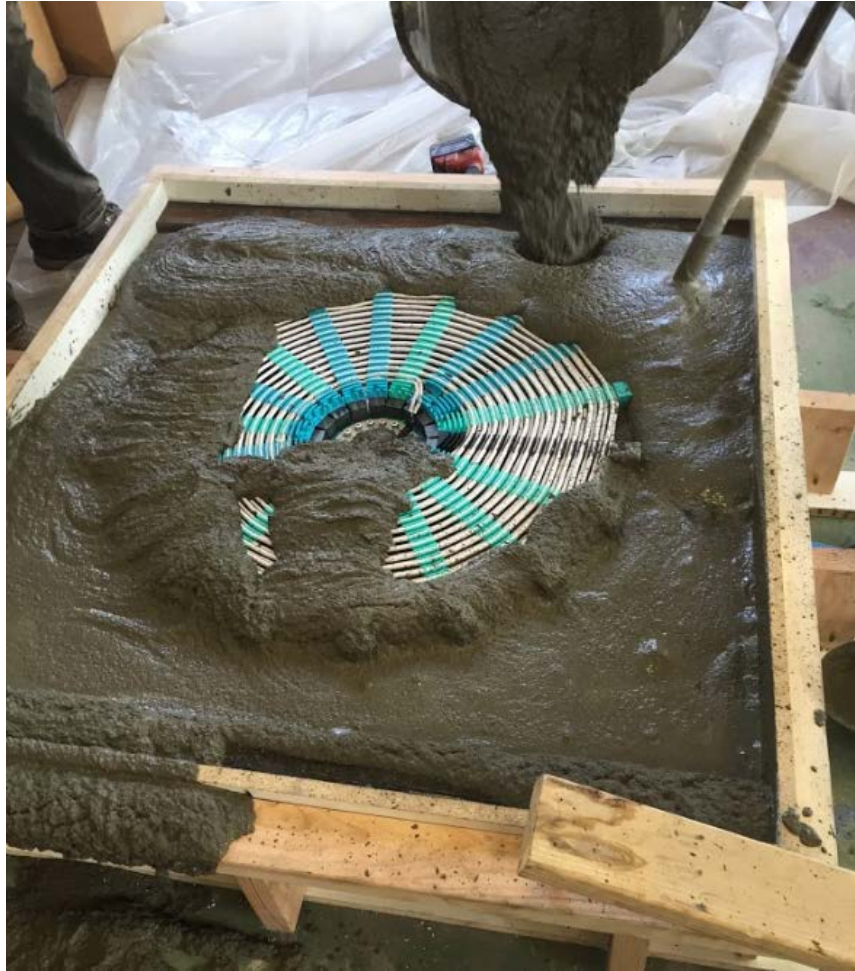
Figure 2.14 Pouring first inductor pad
