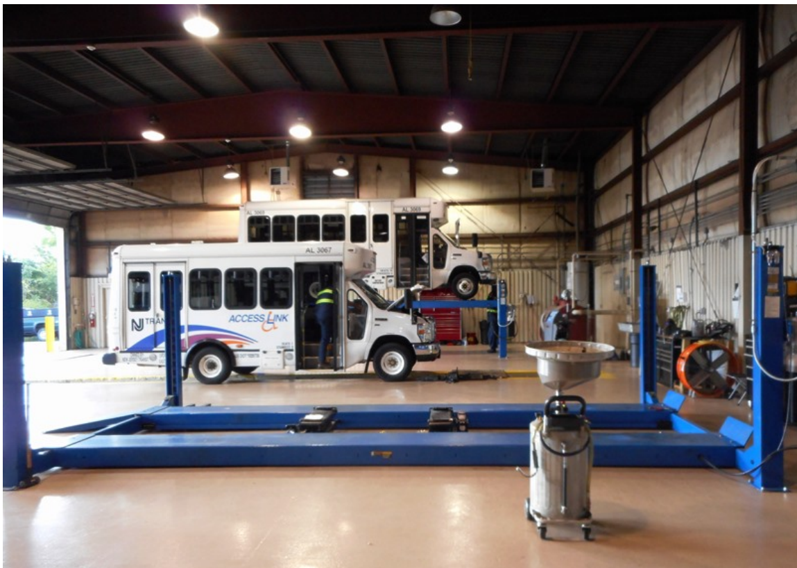
Figure 3. The maintenance area of an Access Link facility
