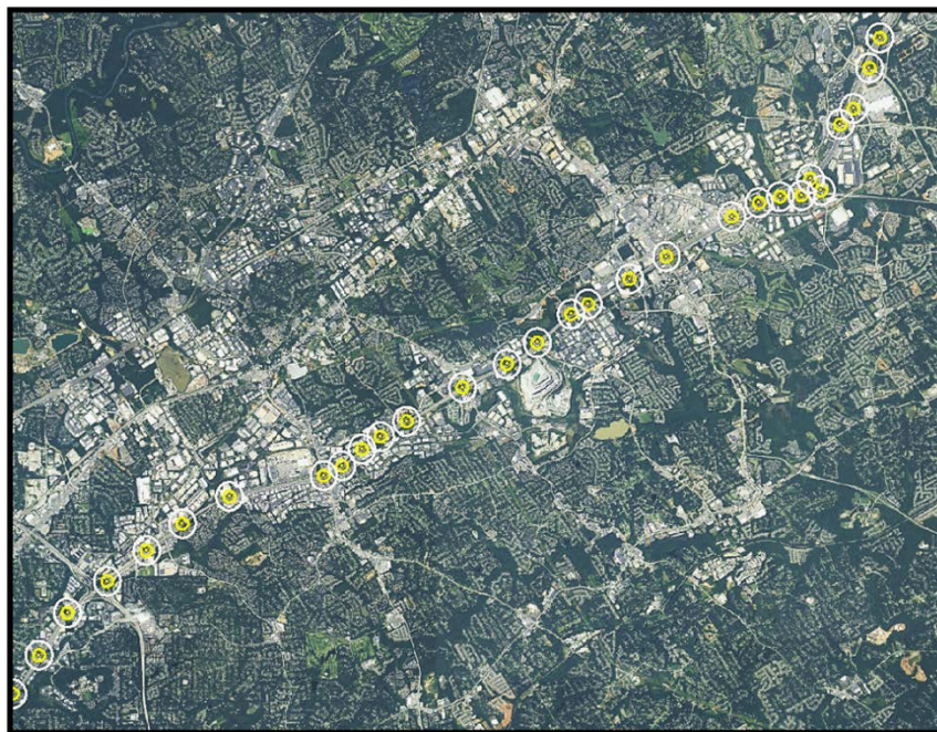
Figure 14: Locations of NaviGator PTZ Cameras on the HOT Corridor
