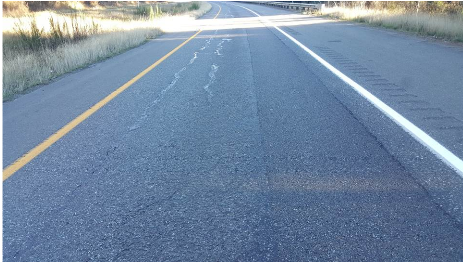
Figure 145. OR4 dig outs plus crack sealing on SR 3. (September 2016)
