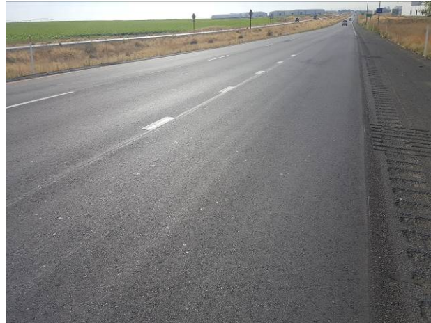
Figure 93. SC4, SR395, Good to Poor, age 26 months. HMA grind/inlay in 2017, C9052.
