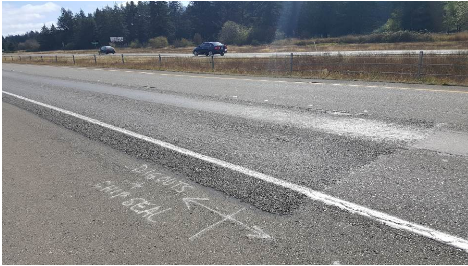
Figure 146. OR2a dig outs plus chip seal SR 8. (September 2016)
