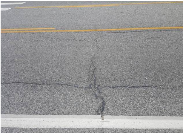
Figure 6. NC2, US2, Good, age 38 months. No spalling or potholes.
