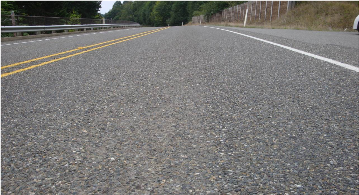
Figure 51. OR1a, SR101, one year after installation. Chip seal looks excellent.
