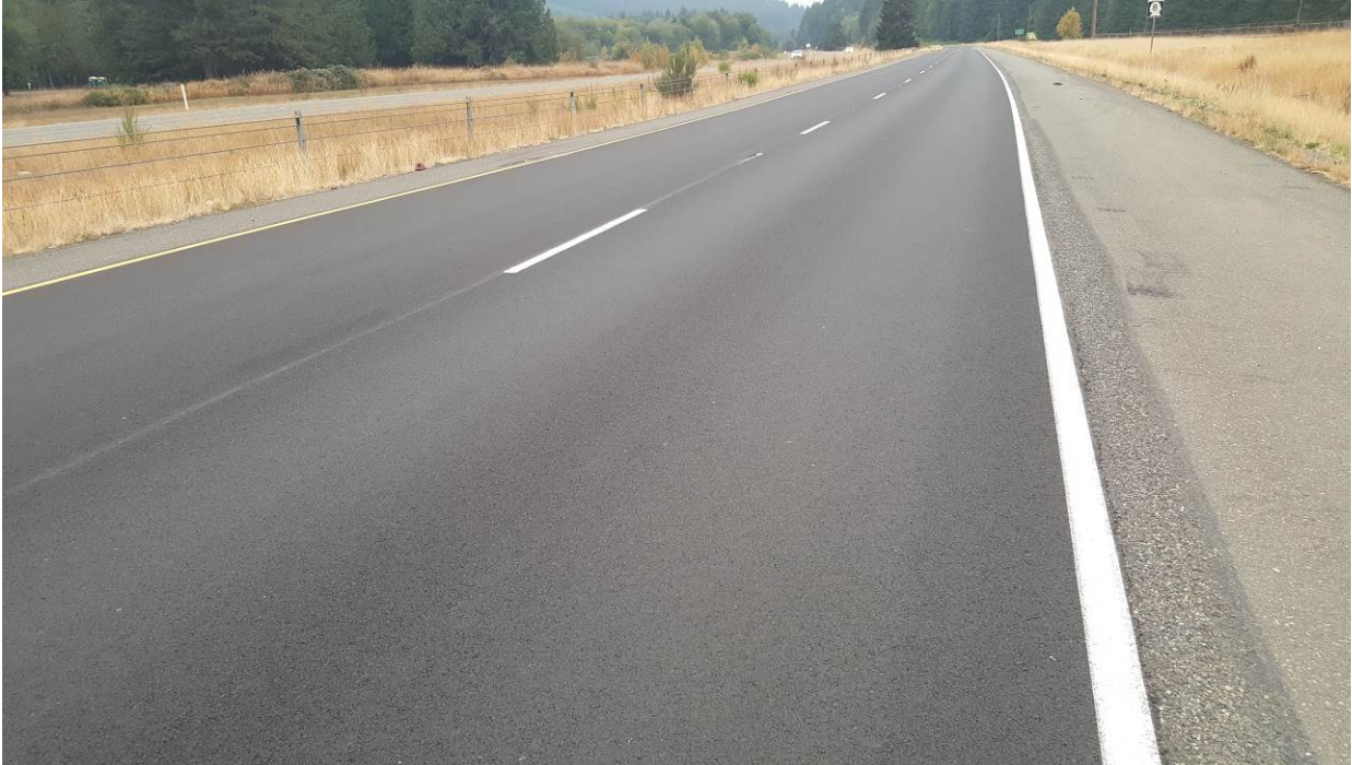
Figure 83. OR2, SR8 five years after installation. HMA grind/inlay in 2017 under Contract 9001.
