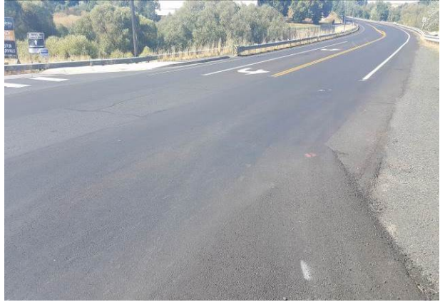
Figure 67. ER11, SR270, Fair, age 37 months. HMA grind/inlay in 2017, C9062.
