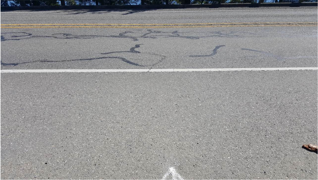
Figure 18. OR1, SR101, four years after installation. There has not been much change in the condition of the crack sealant since year one.
