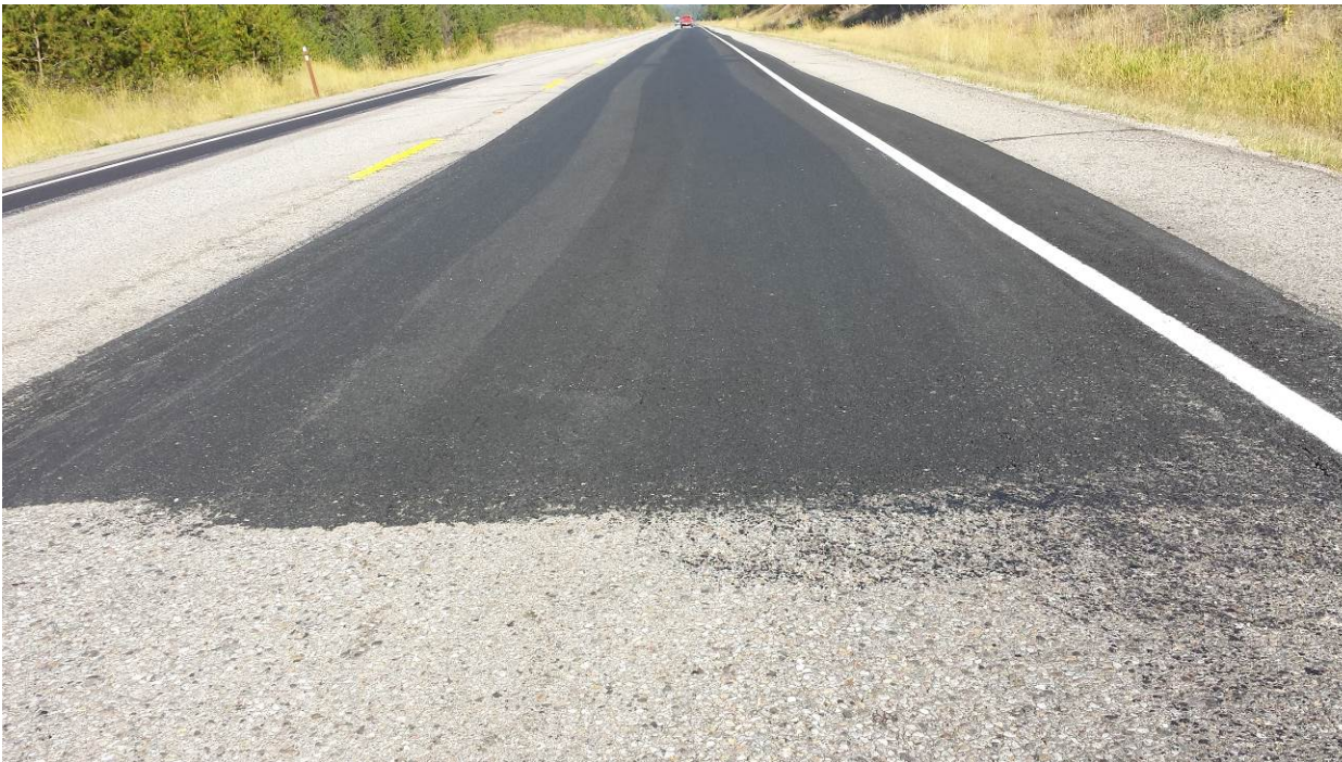
Figure 121. ER9a, SR395, a few months after installation. Blade patch looks excellent.
