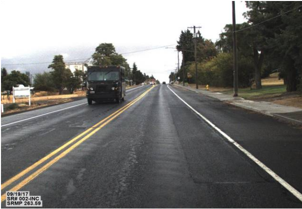
Figure 60. ER5, US2, Poor, age 49 months. Transverse reflection crack at the age of 10 months.
