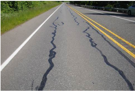
Crack Seal
