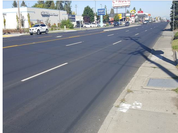
Figure 57. ER2, US2, Fair, age 62 months. HMA grind/inlay in 2017, C9063.
