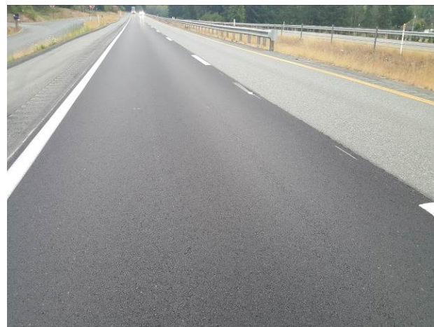
Figure 3. OR6, SR8, Good, age 50 months. HMA grind/inlay in 2017, C9001.
