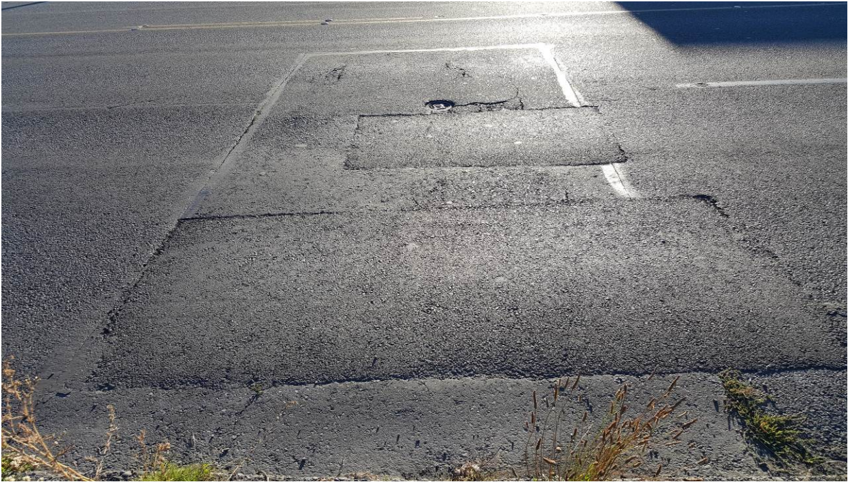
Figure 88. OR5, SR7, three years after installation. No change in the dig out patches.
