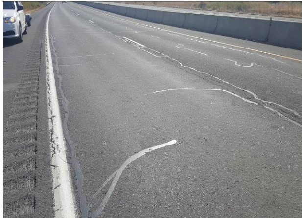
Figure 7. SC1, SR97, Good, age 25 months. No spalling or potholes.
