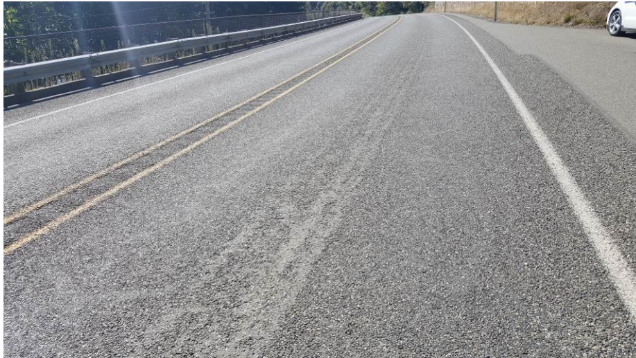
Figure 142. OR1a crack sealing plus chip sealing on SR 101. (September 2016)
