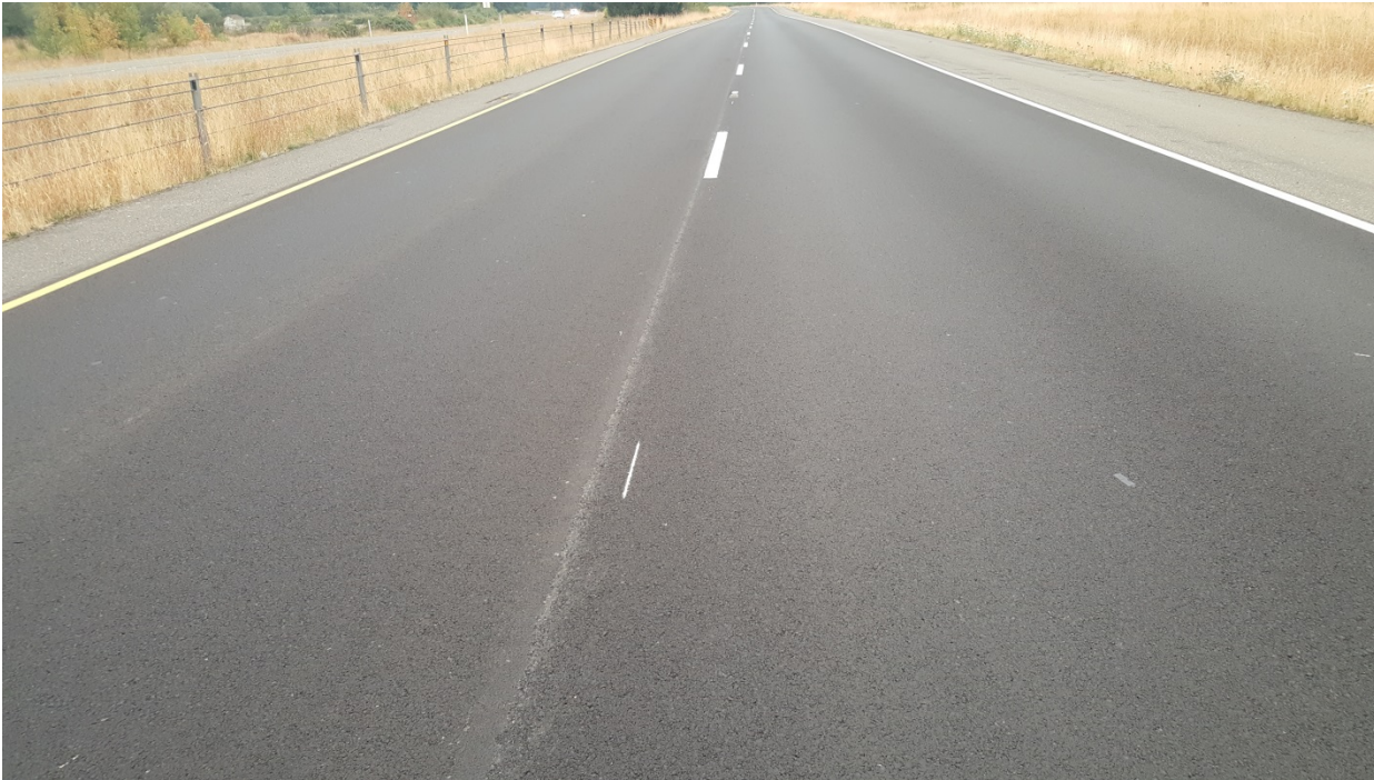
Figure 111. OR2a, SR8, the site received an HMA grind/inlay in 2017, C9001, five years after installation.
