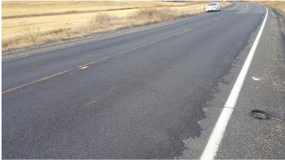
Figure 143. ER20 blade patch on SR 395. (September 2016)
