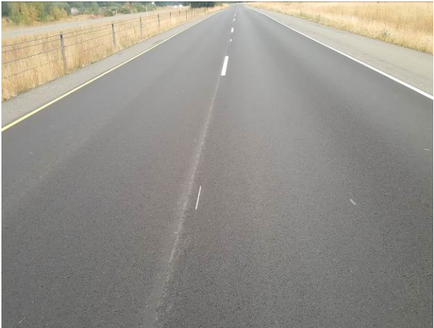
Figure 100. OR2a, SR8, Good, age 62 months. Flushing over the dig out patches. HMA grind/inlay in 2017, C9001.
