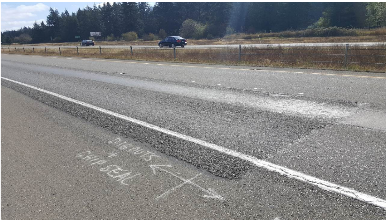
Figure 110. OR2a, SR8, four years after installation. Flushing has remained about the same as in 2015.
