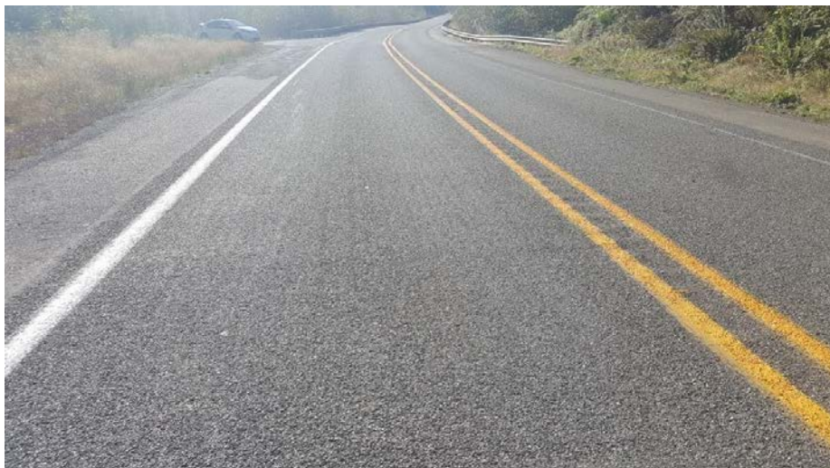
Figure 141. OR3b full lane chip seal on SR 101. (September 2016)
