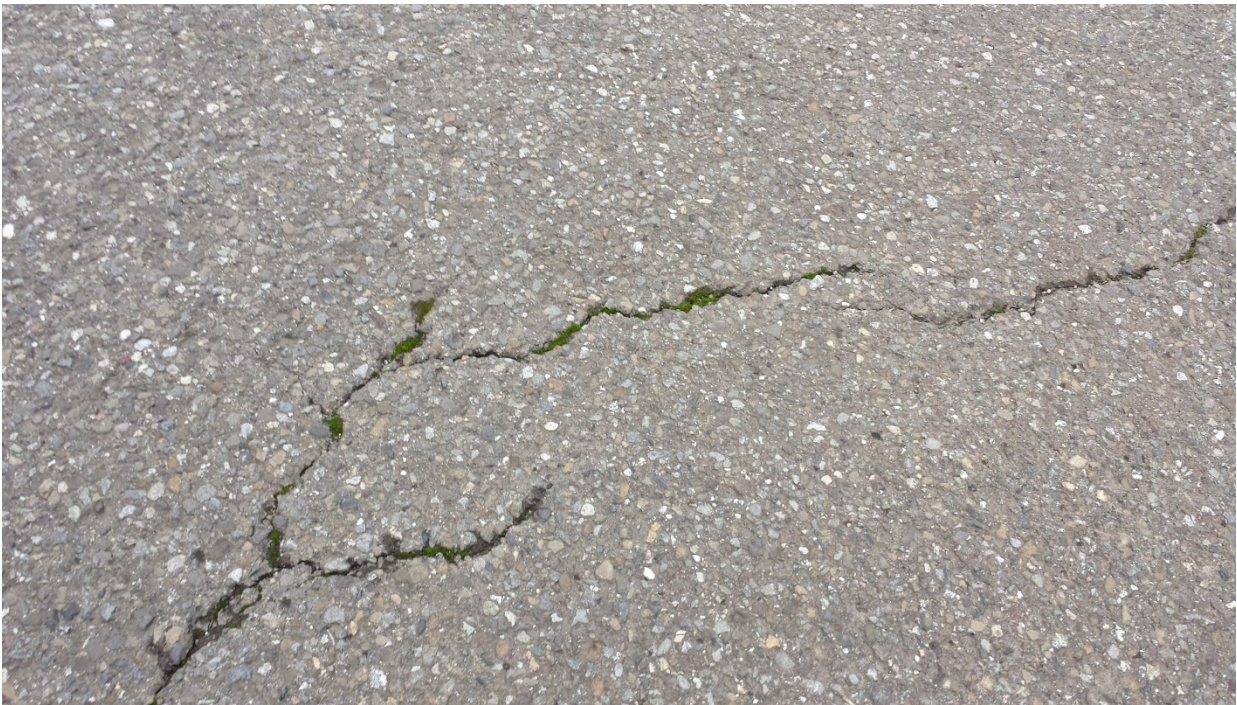
Figure 131. OR3a, SR101, two years after the other sections were treated. Vegetation growing in the wider cracks.
