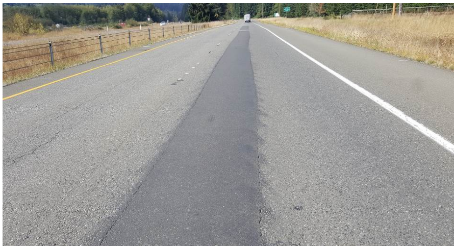
Figure 144. OR2 dig outs on SR 8. (September 2016)
