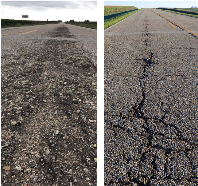
CR L-40 Otta seal project site prior to any surface treatment
