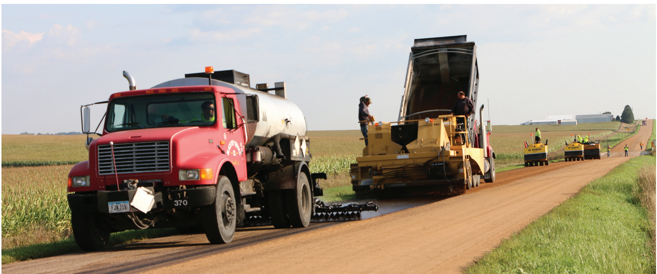
Otta seal construction process: binder spraying, aggregate application, and rolling compaction
