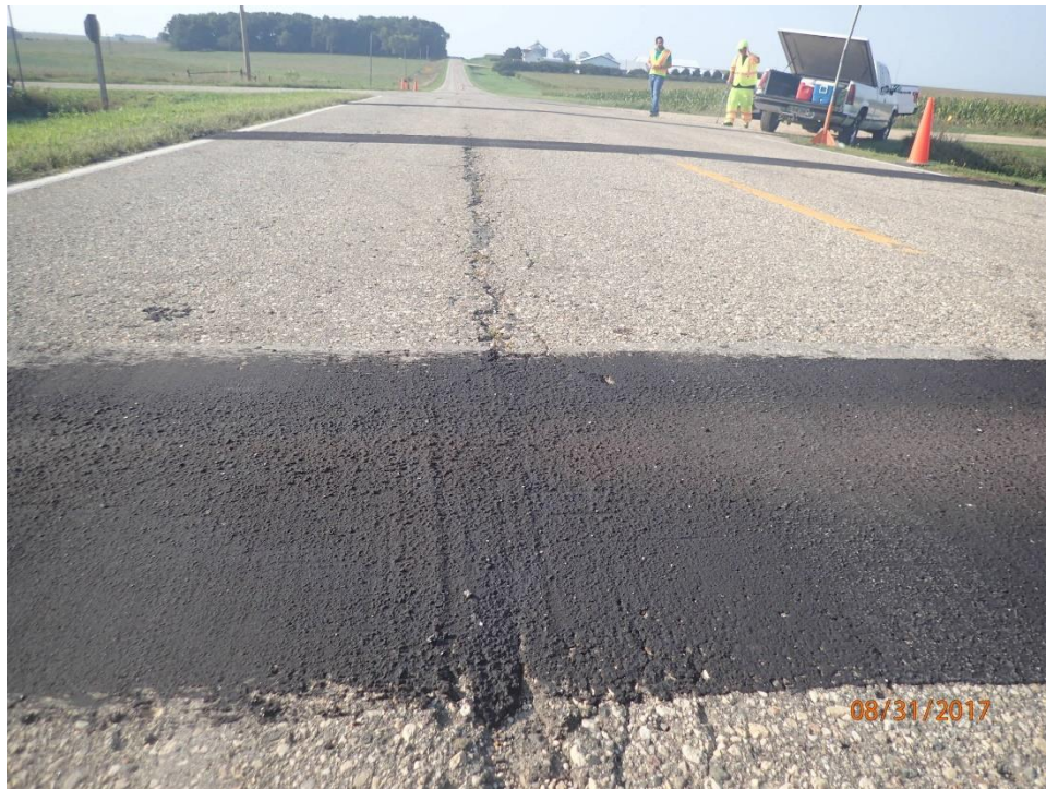
Figure 101. Slurry sealed cracking area
