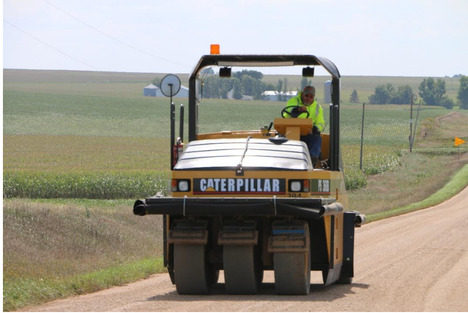
Figure 114. Compaction efforts during the first layer construction
