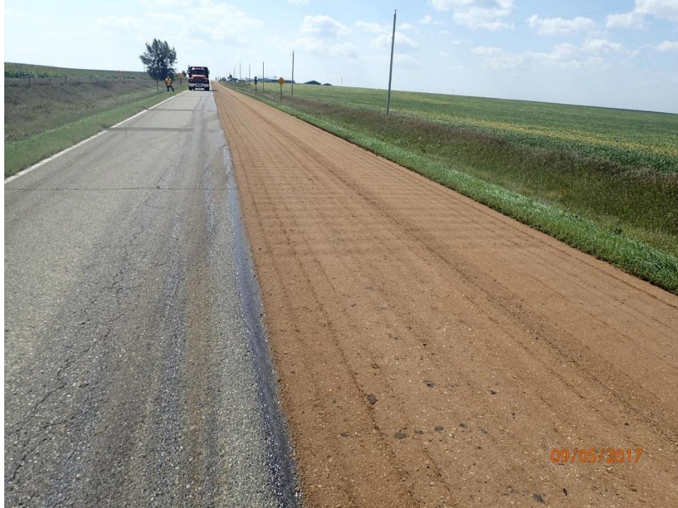
Figure 108. Otta seal first layer construction on CR L-40
