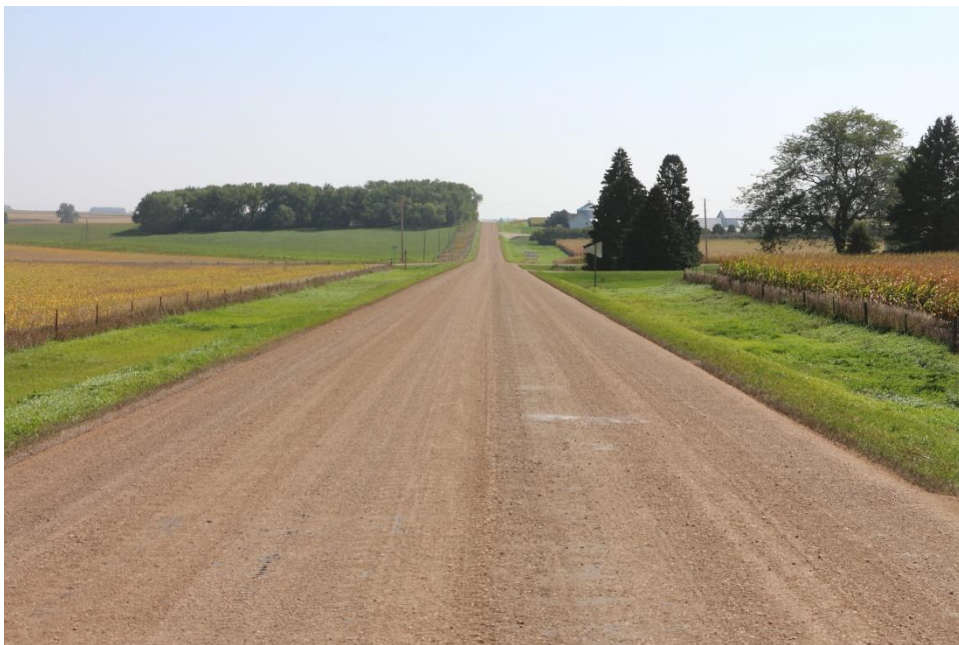
Figure 125. Appearance of Otta seal surface two days post construction
