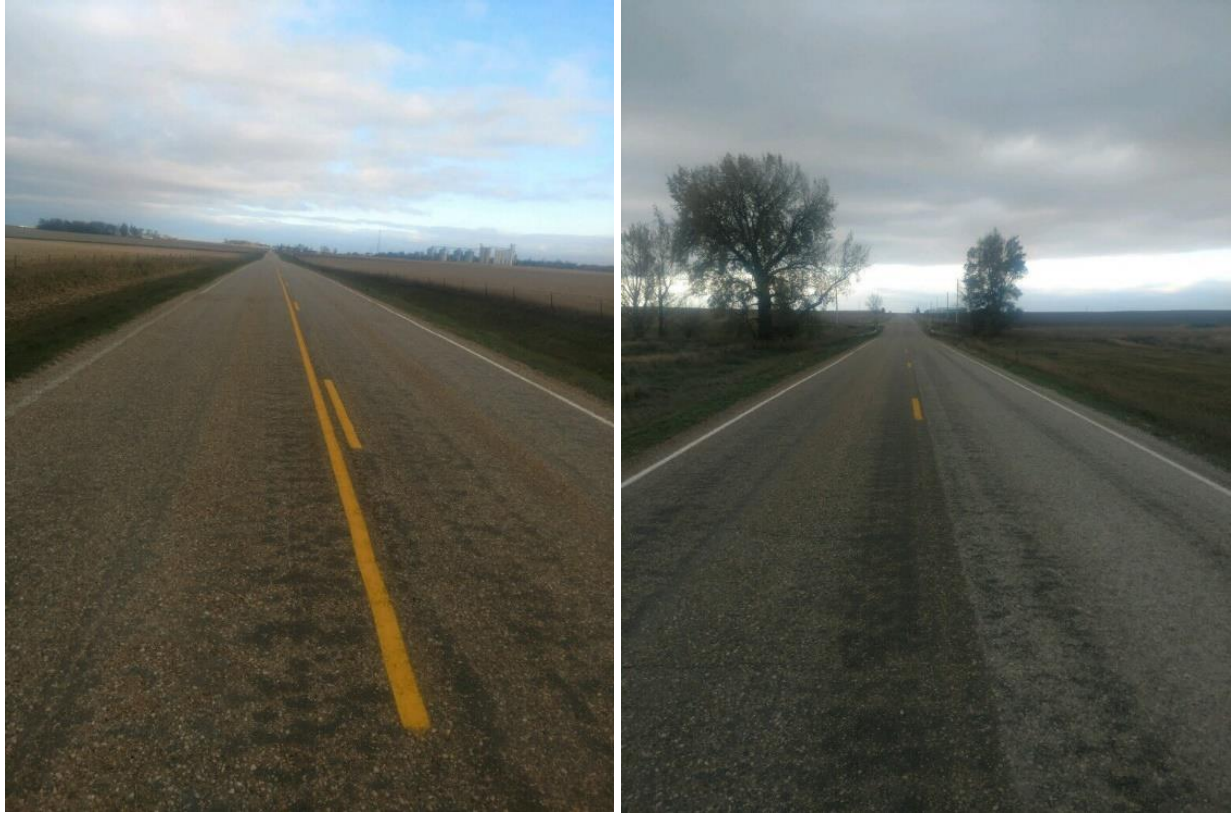
Figure 71. Three months after second layer construction
