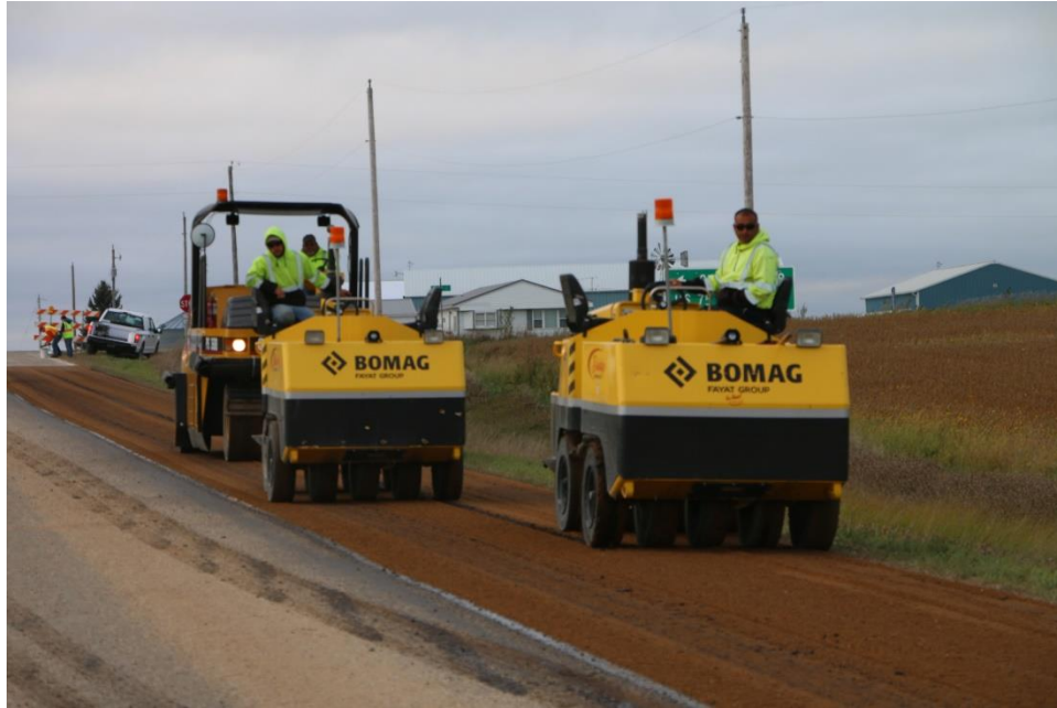
Figure 120. Compaction immediately after applying binder and aggregates
