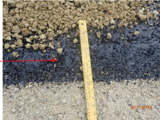
Figure 28. Completed sections showing a lack of rain-related damage
