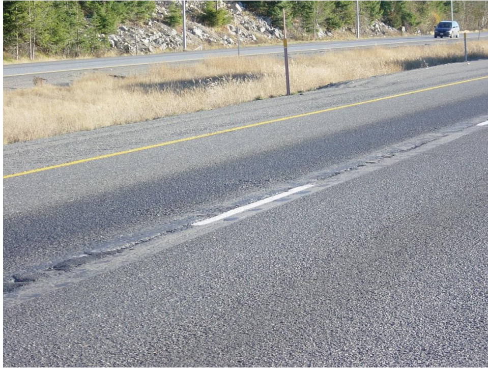
Figure 7. Maintenance patch on a longitudinal joint covered by a fog seal
