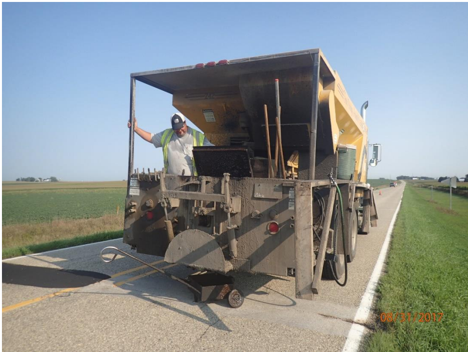
Figure 95. During the process of applying slurry seal
