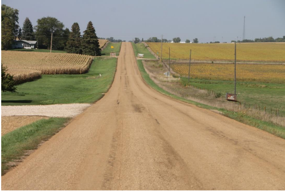
Figure 128. Appearance of Otta seal two days post construction showing color changes
