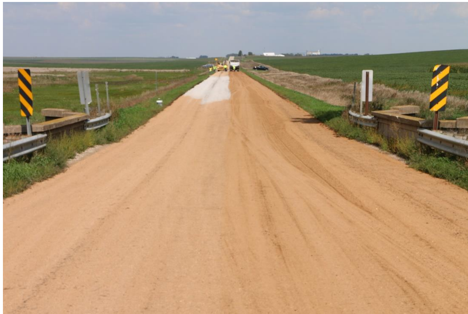
Figure 109. Otta seal first layer construction
