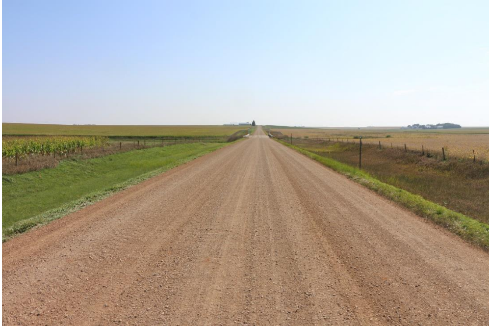
Figure 132. Appearance of Otta seal two days post construction with wheel paths
