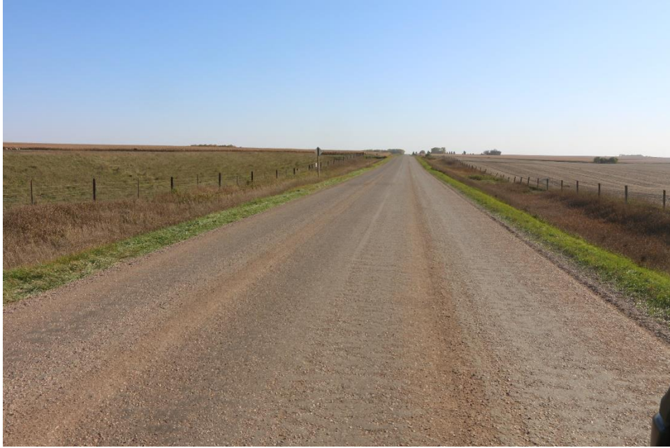
Figure 136. Appearance of Otta seal two weeks post construction showing surface color differences
