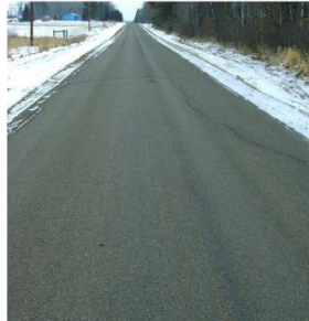
Otta Seal constructed 2001, Cass County CR171
