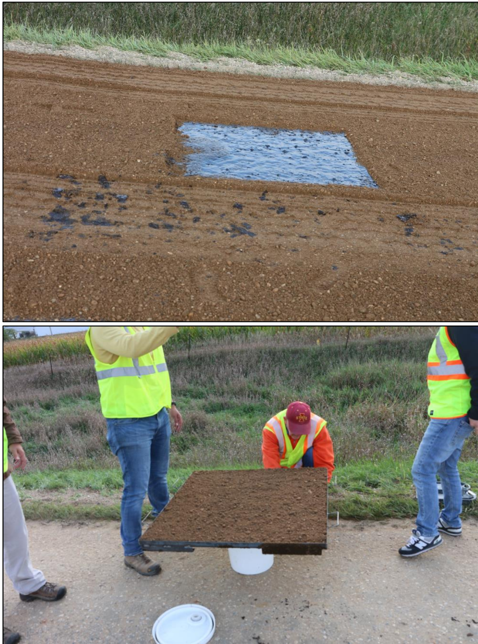
Figure 58. Measurement of the weight of aggregate per unit area
