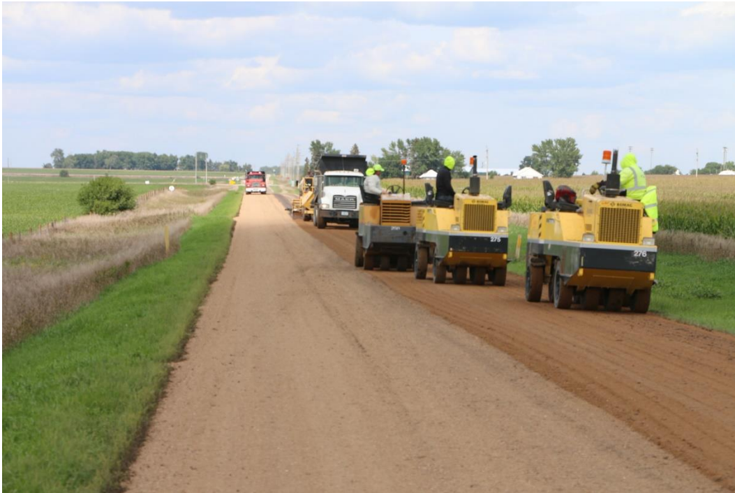
Figure 113. Compaction after applying binder and aggregates
