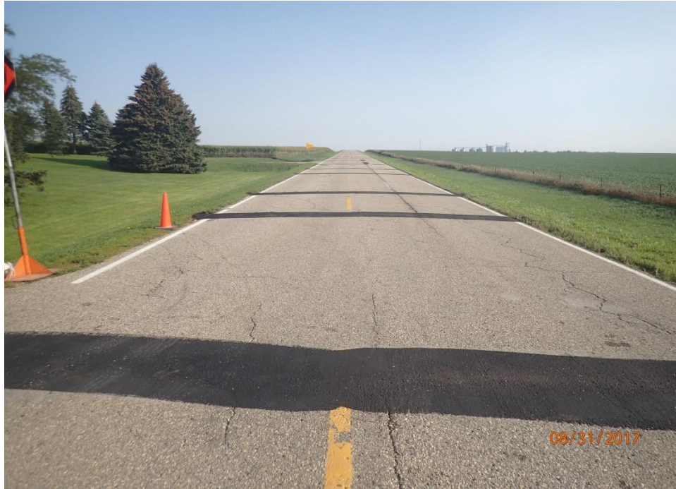
Figure 100. View of slurry sealed sections
