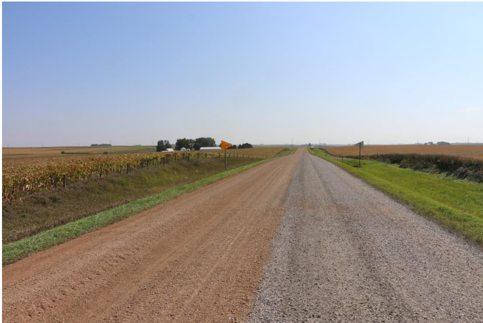
Figure 129. Appearance of Otta seal two days post construction comparing two test sections
