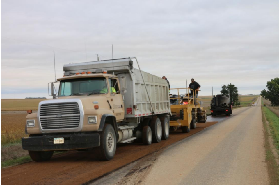
Figure 118. Binder, aggregate, and construction equipment for second layer construction
