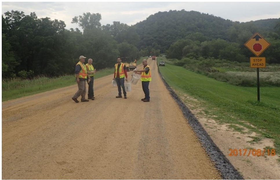
Figure 25. Newly placed Otta seal in Winona County, Minnesota
