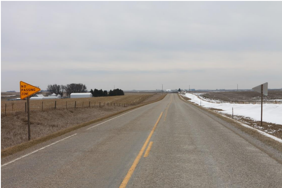
Figure 147. Appearance of Otta seal surface six months post construction
