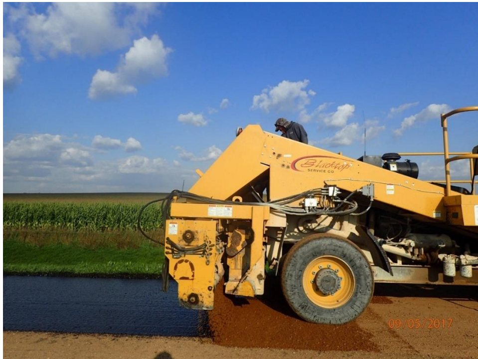
Figure 103. Aggregate application during the first layer construction
