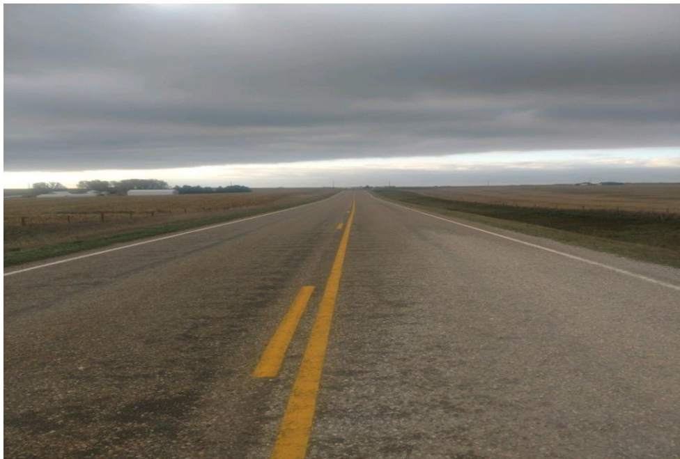
Figure 145. Appearance of Otta seal surface two months post construction, with one test section showing relatively lighter color
