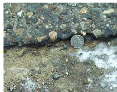
Otta Seal constructed 2003, NE of Cass County CR168
