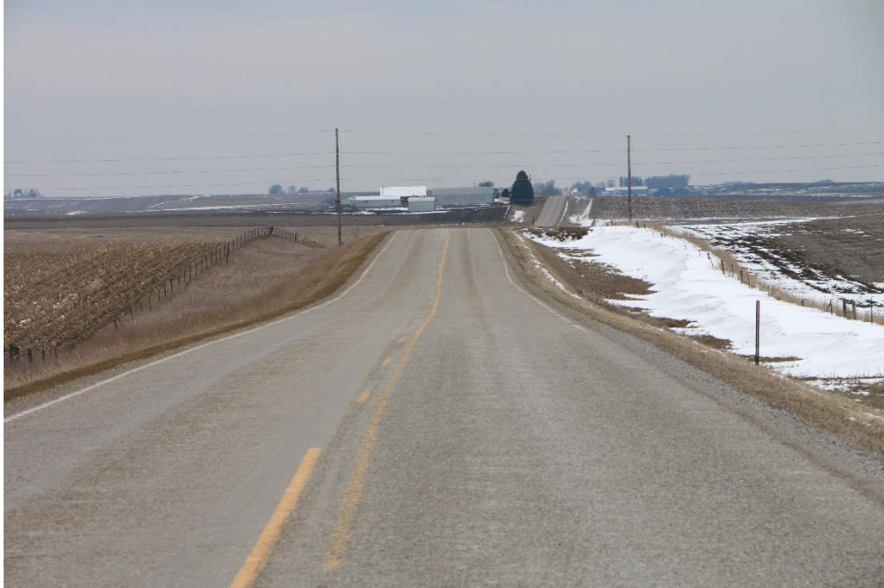
Figure 148. Appearance of Otta seal surface six months post construction – long view
