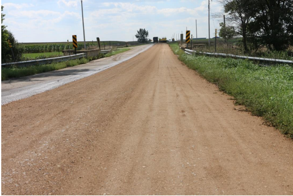
Figure 106. Otta seal first layer construction near 530th Street
