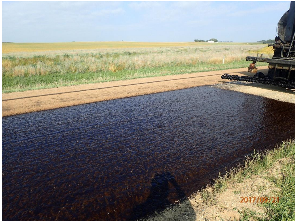
Figure 123. Binder spraying during second layer construction
