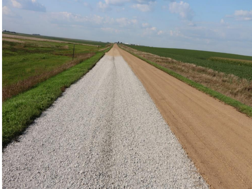
Figure 49. TS 1 using crushed limestone – asphalt aggregate
