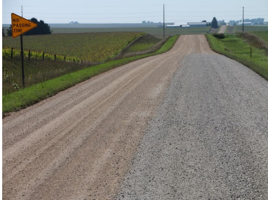
Figure 51. TS 3 using crushed limestone – Class A aggregate
