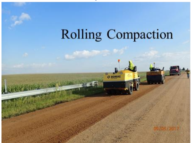
Figure 47. Three key steps during Otta seal construction
