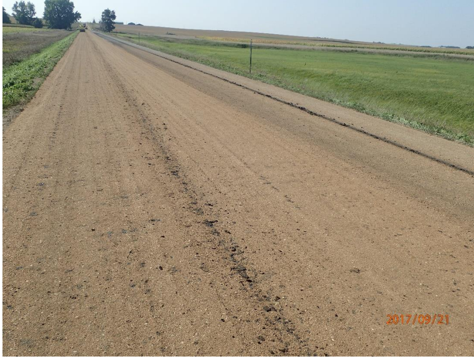
Figure 122. Appearance of Otta seal second layer immediately after construction
