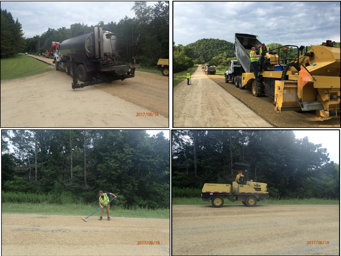
Figure 23. Equipment used for Otta seal on CR 116, Winona County, Minnesota
