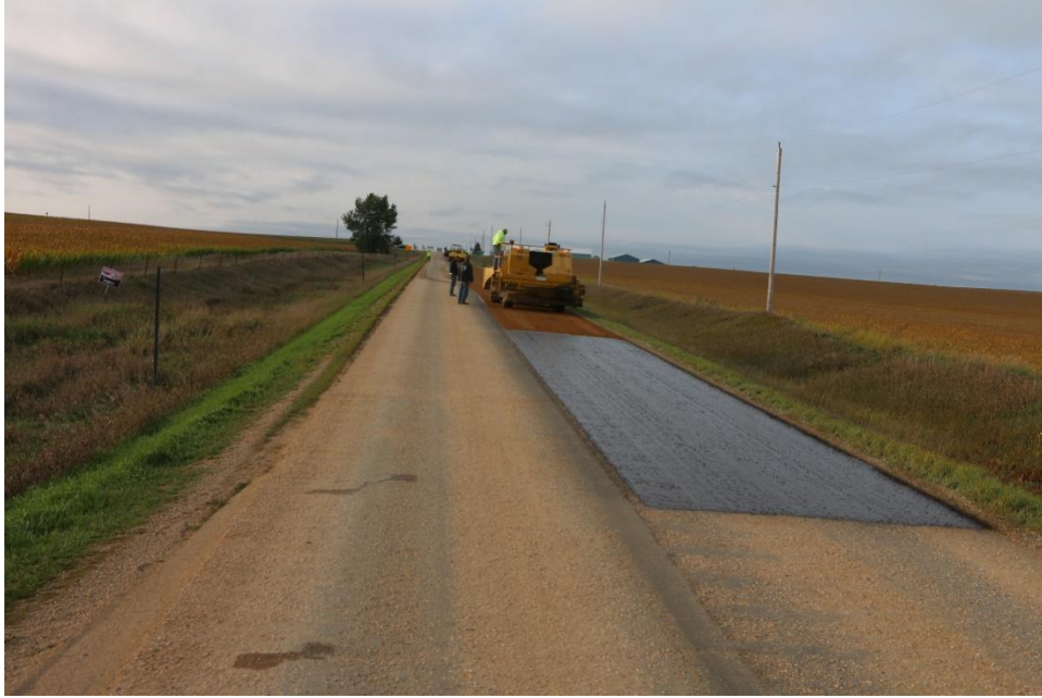
Figure 124. Aggregate application during second layer construction
