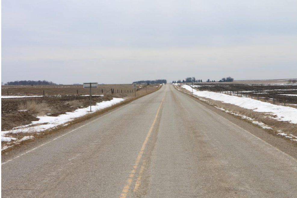
Figure 146. Appearance of Otta seal surface six months post construction, showing deteriorated pavement marking
