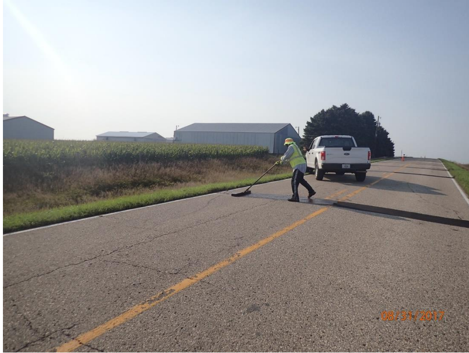
Figure 96. Applying slurry seal
