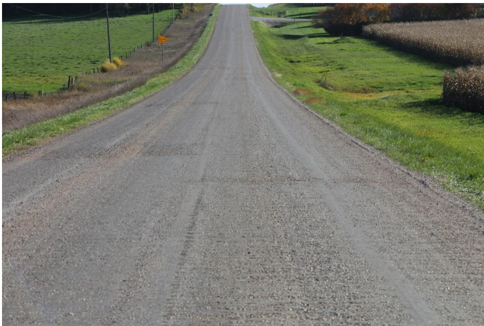
Figure 133. Appearance of Otta seal two weeks post construction showing color change
