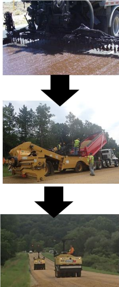
Figure 3. Surface treatment operation sequence
