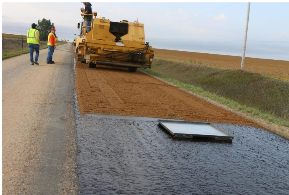
Figure 121. Quality control test to insure an accurate application rate of aggregate
