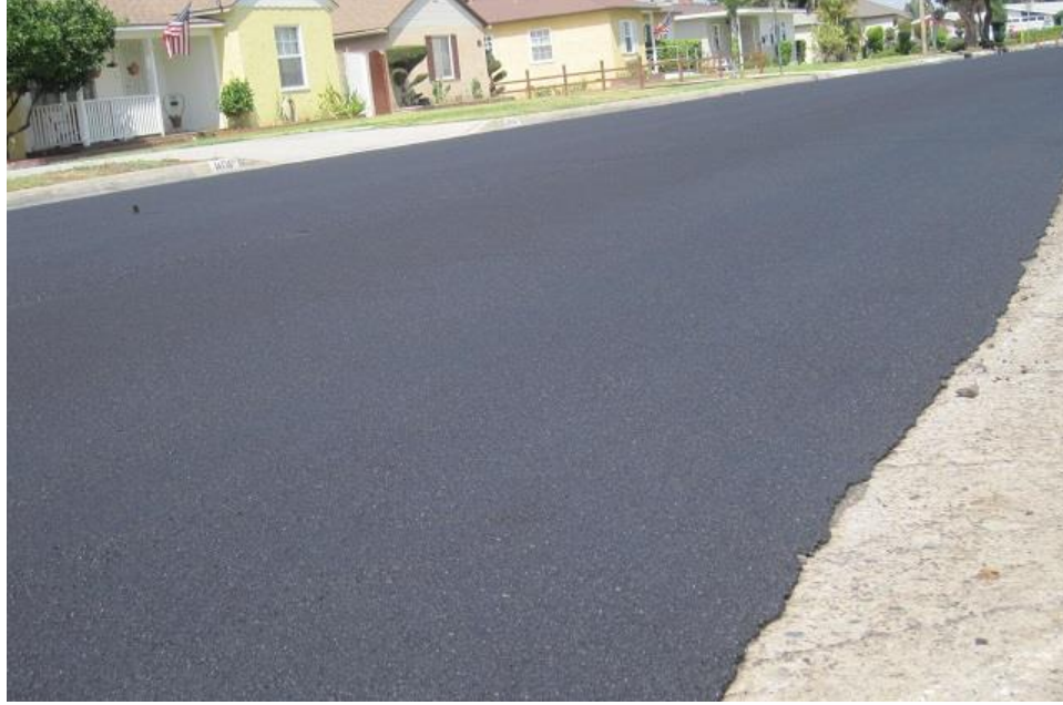
Figure 4. Slurry-sealed road one hour after application
