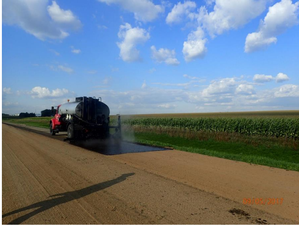
Figure 102. Binder application during the first layer construction
