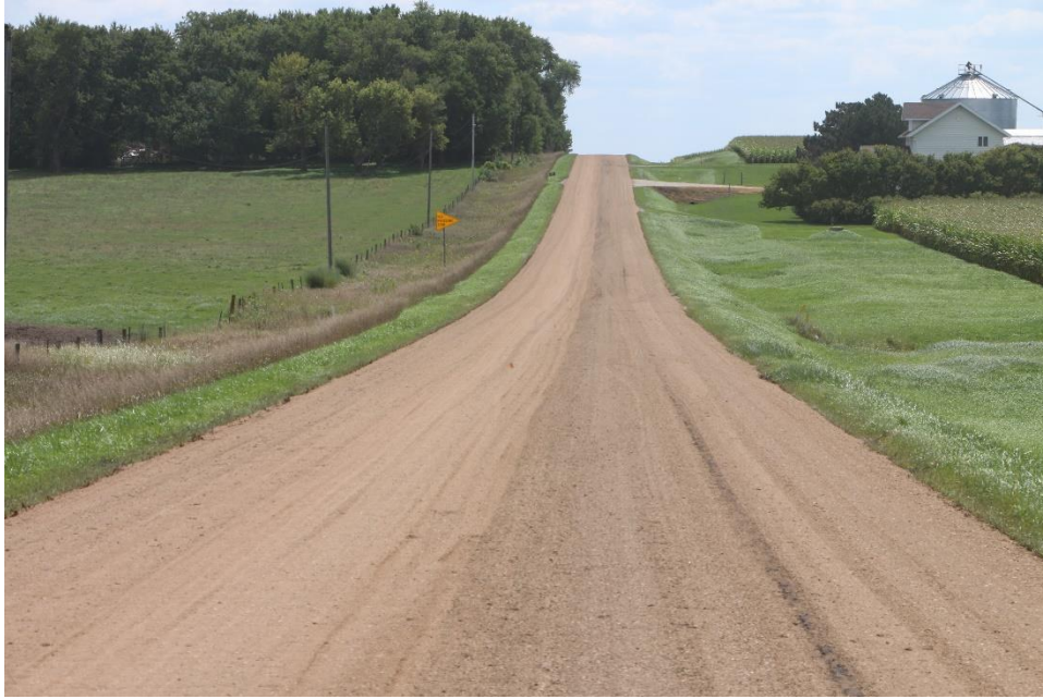
Figure 116. Appearance of Otta seal first layer comparing two lanes with different compaction efforts
