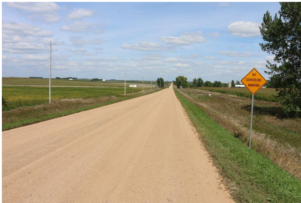
Figure 115. Appearance of Otta seal first layer immediately after construction
