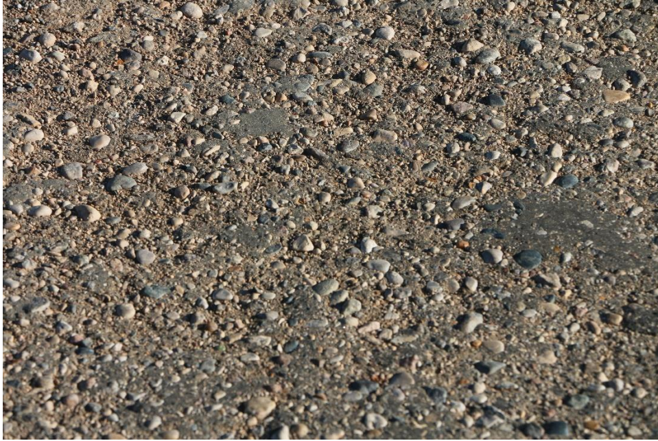
Figure 140. Appearance of Otta seal surface two weeks post construction, showing binder squeezed up to surface
