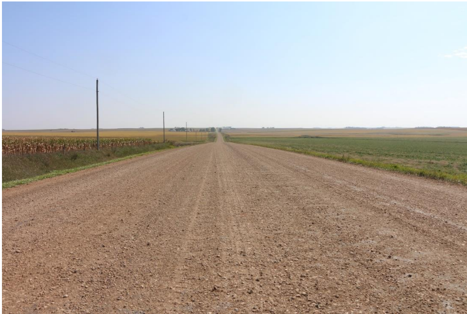
Figure 131. Appearance of Otta seal two days post construction – long view
