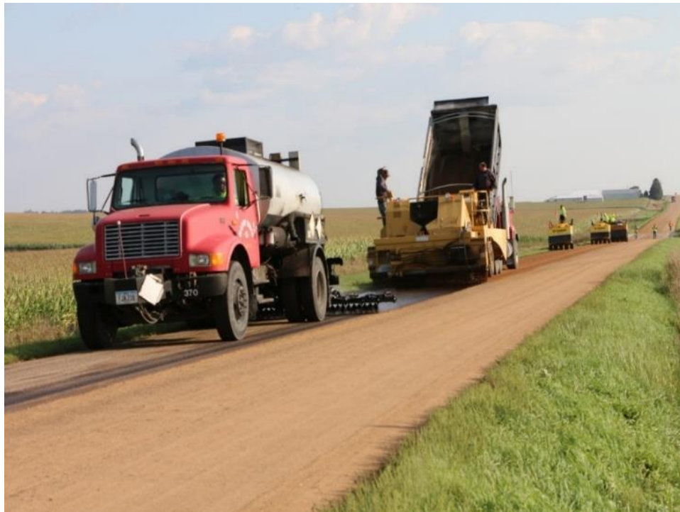
Figure 48. The entire Otta seal construction process
