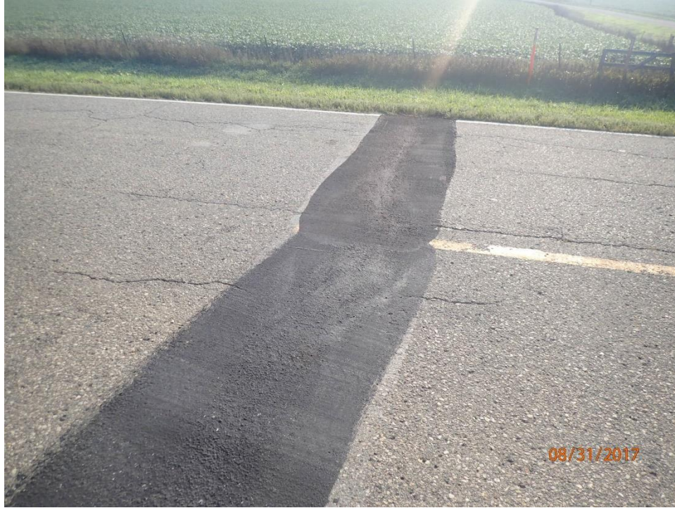
Figure 98. Slurry sealed area
