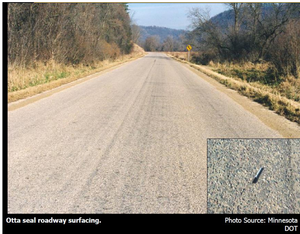
Figure 8. Otta seal surfacing
