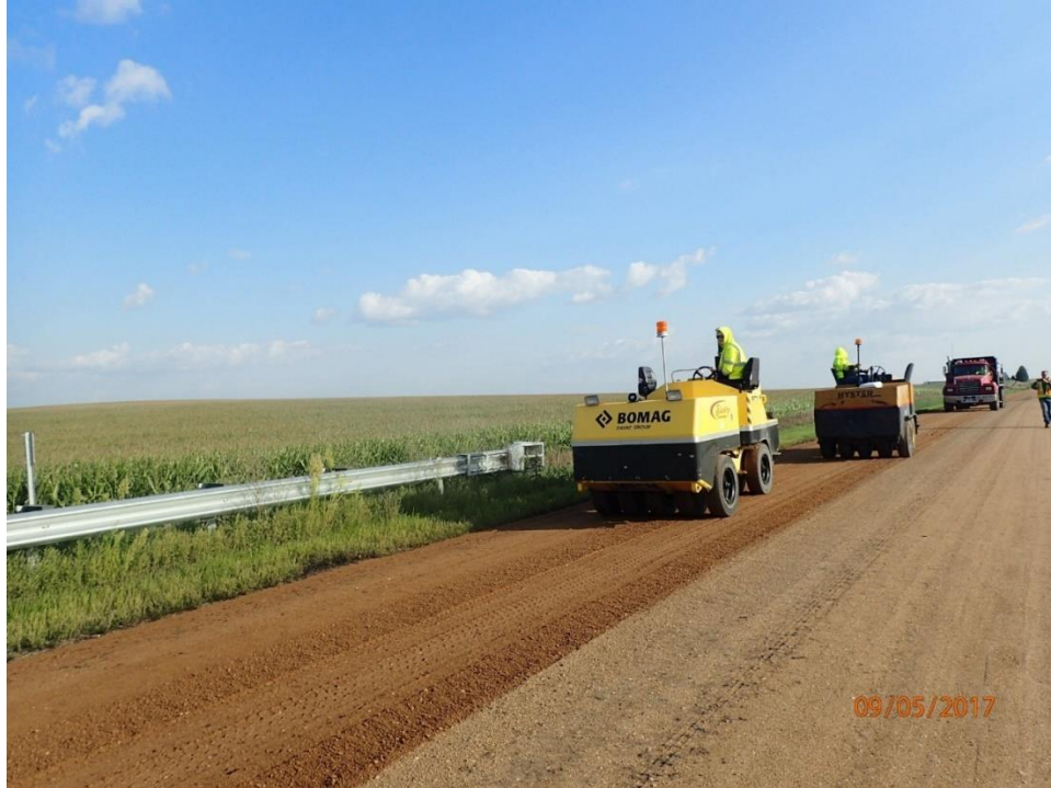
Figure 104. Compaction work during the first layer construction
