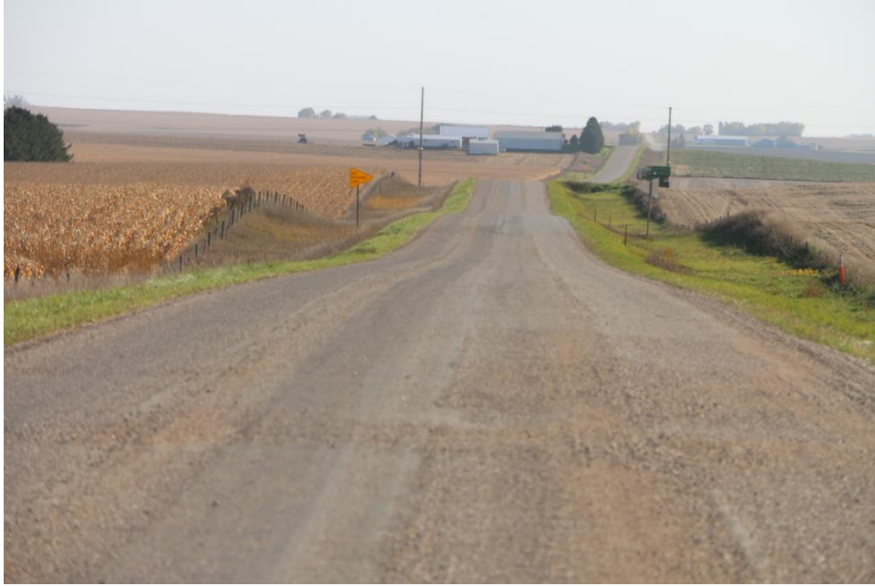
Figure 134. Appearance of Otta seal two weeks post construction – long view
