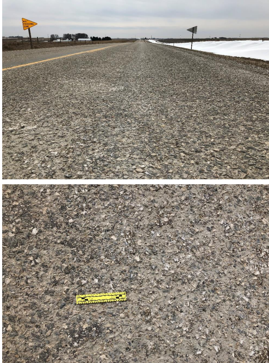
Figure 72. Six months after second layer construction
