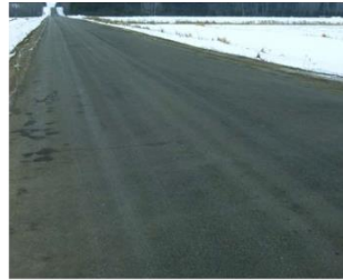
Otta Seal constructed 2001, Cass County CR25 – Dairy Farm.
