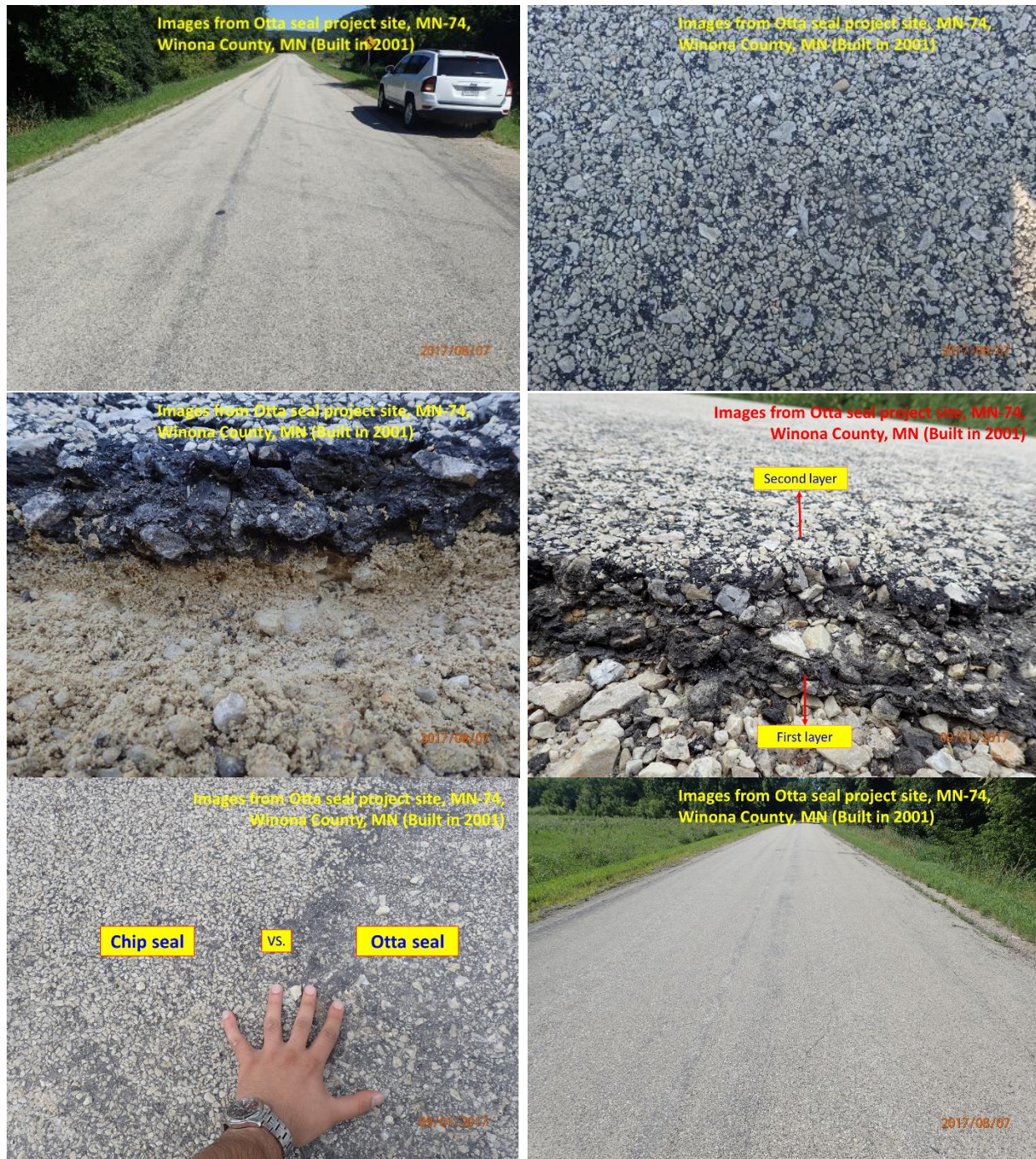
Figure 30. Performance of Otta seal on MN 74 Winona County, Minnesota
