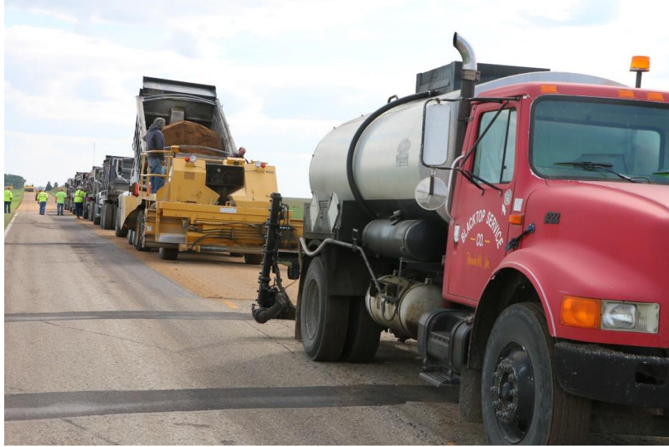
Figure 110. Binder, aggregate, and other construction equipment
