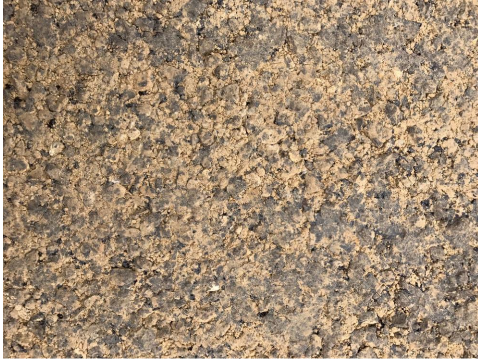
Figure 26. Otta seal surface texture immediately after constructing the first layer in Winona County, Minnesota
