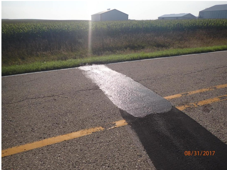
Figure 97. Slurry seal applied on the HMA cracking area
