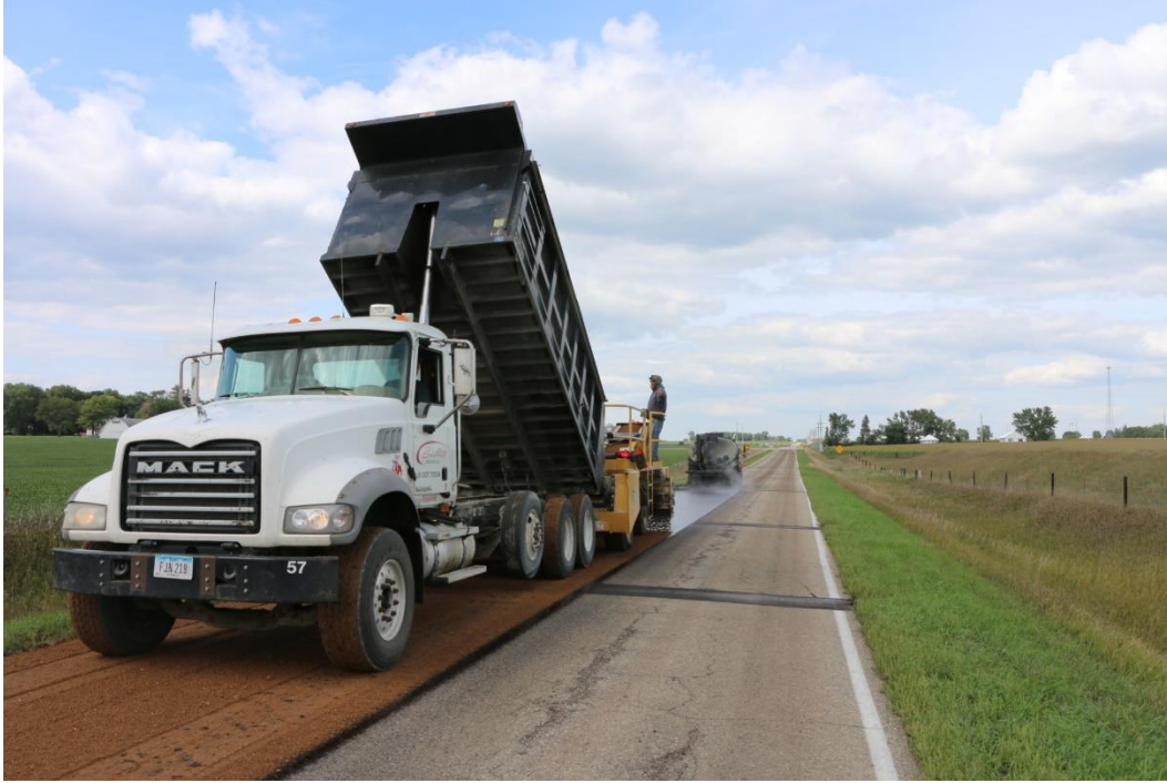
Figure 112. Binder and aggregate applications
