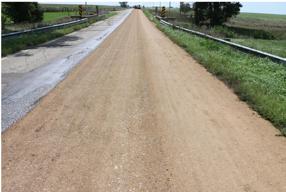
Figure 107. Otta seal first layer construction on CR L-40 near 530th Street
