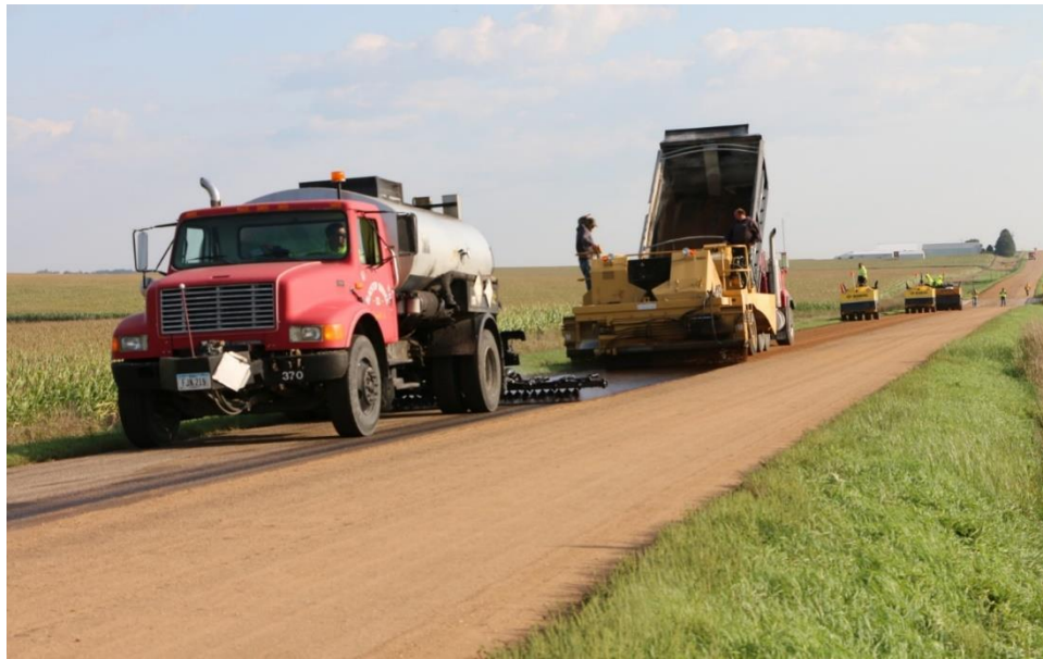
Figure 105. The complete processes of Otta seal construction
