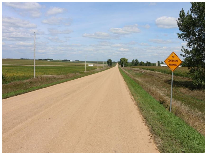
Figure 66. First layer appearance: two days after application
