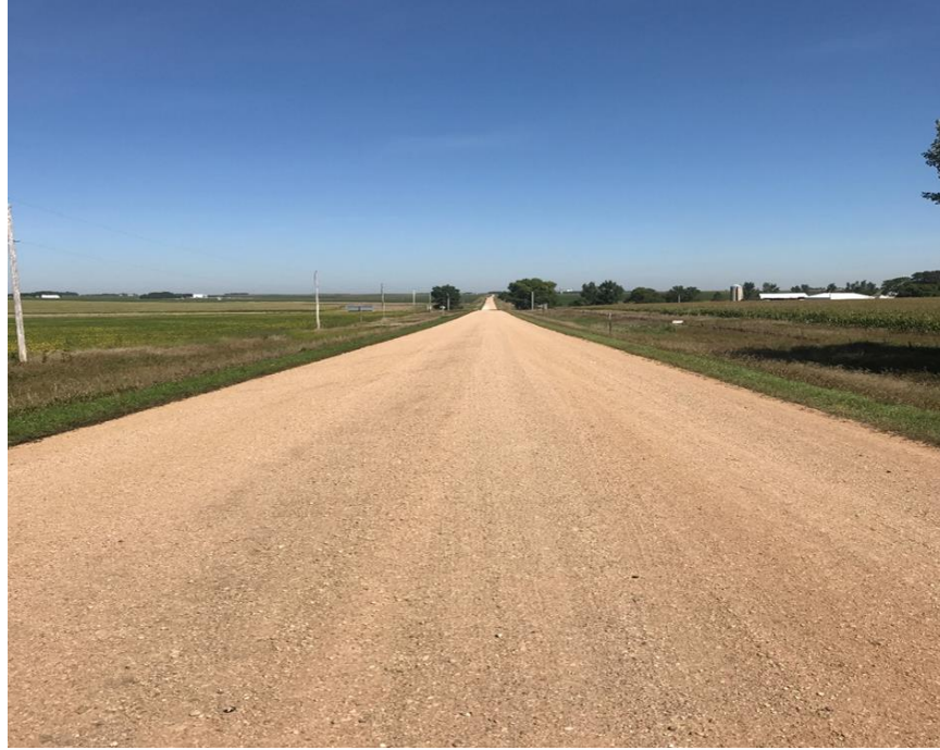
Figure 67. First layer appearance: three days after application
