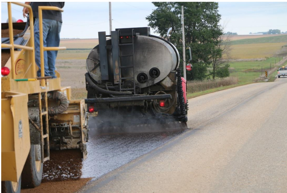
Figure 119. Binder and aggregate application during second layer construction
