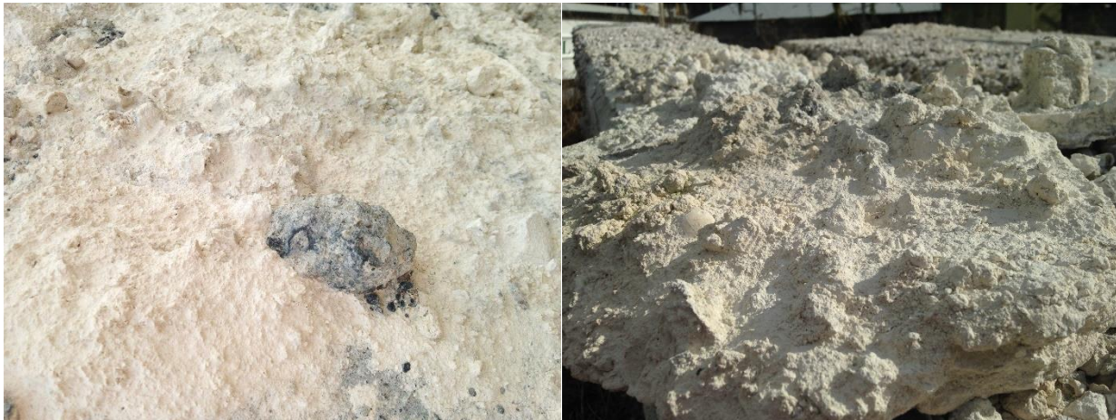
Figure 2.44 Figure 3.5. Limestone adhered to piles extracted from Gandy Bridge / Friendship Trail over Tampa Bay.
