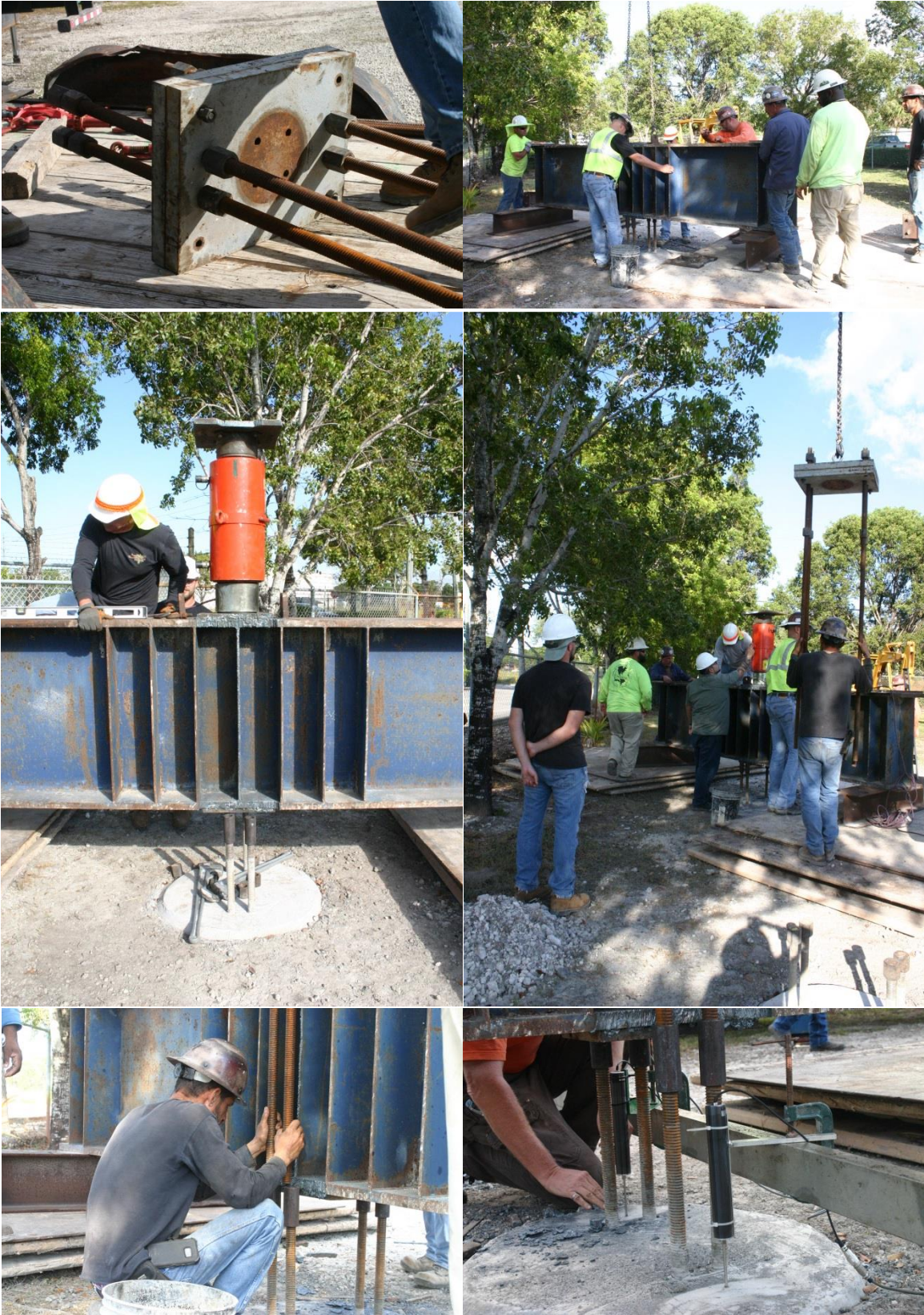
Figure 4.17 Load test setup.
