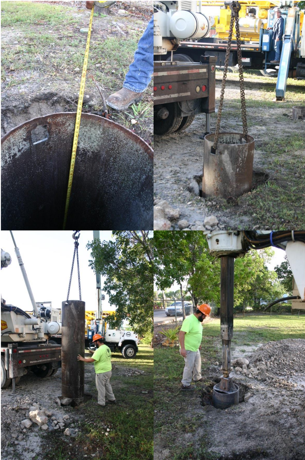
Figure 4.11 Casing extraction and clean out of uncased control shaft.
