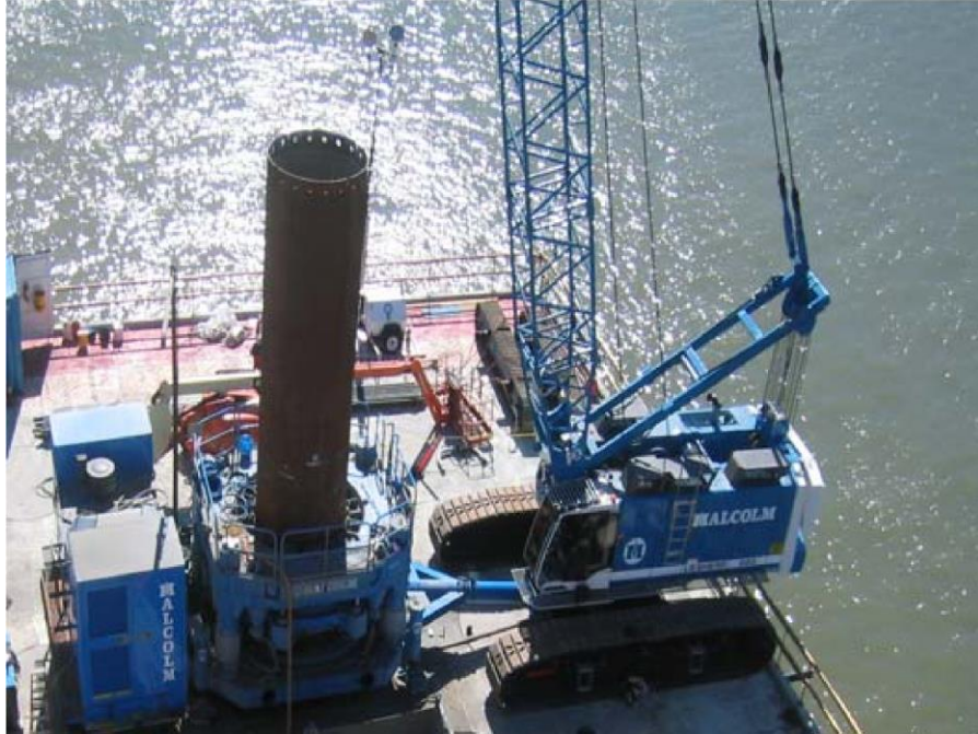
Figure 2.12 Example of rotator machine (Malcolm, 2016).
