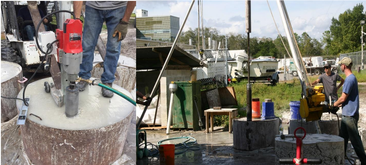
Figure 3.9 Pre-drilling (left) and driving the casing (right).
