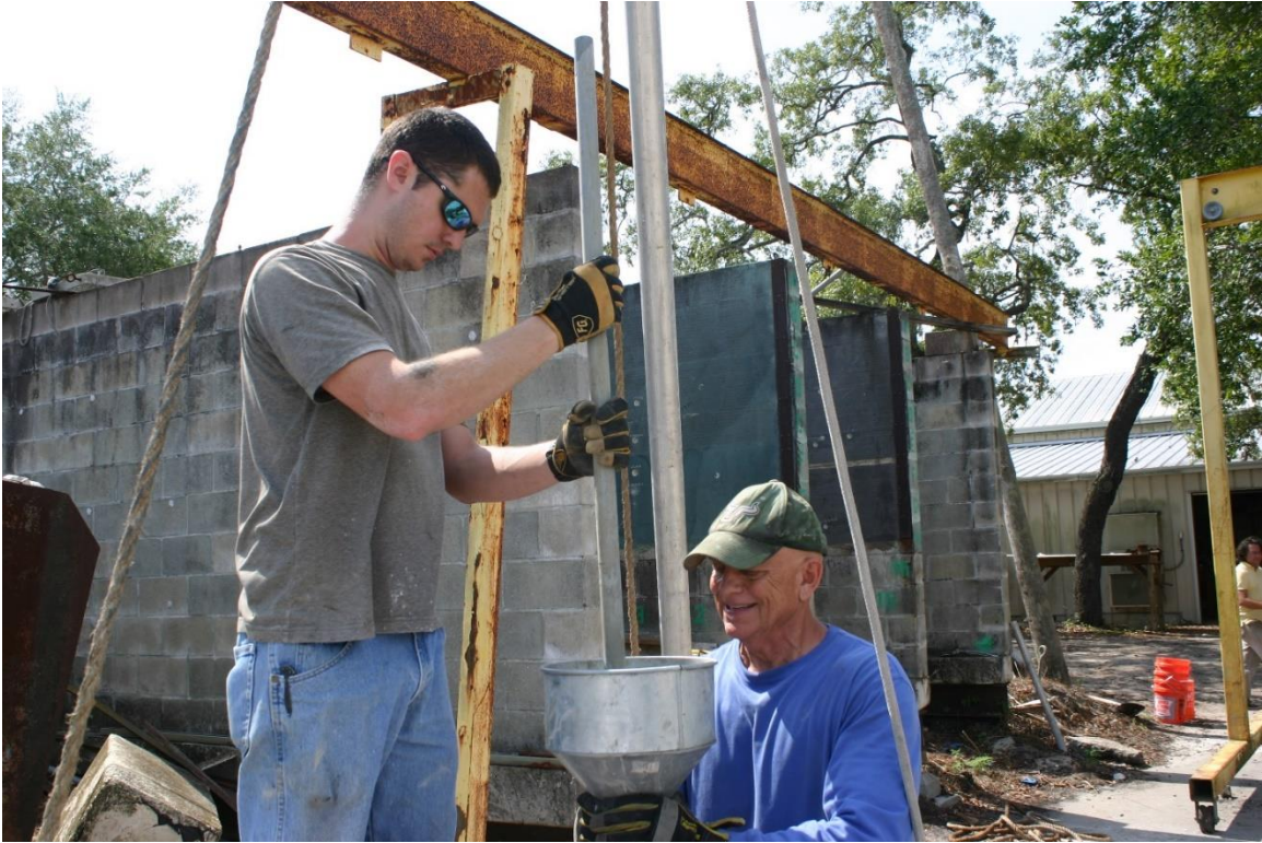
Figure 3.15 Anchor rod placed in tremie before concreting.
