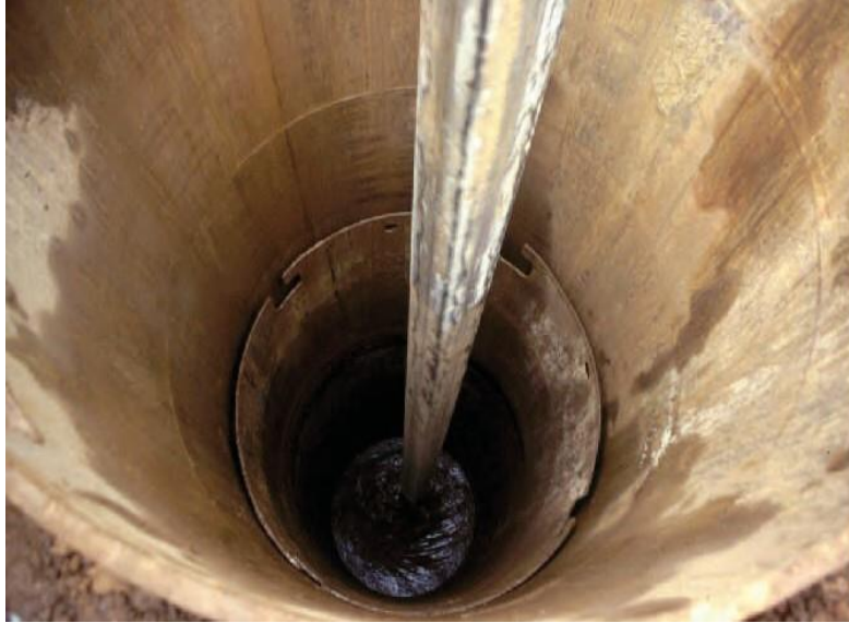
Figure 2.13 Telescoping Casing, most likely permanent (FHWA, 2010).
