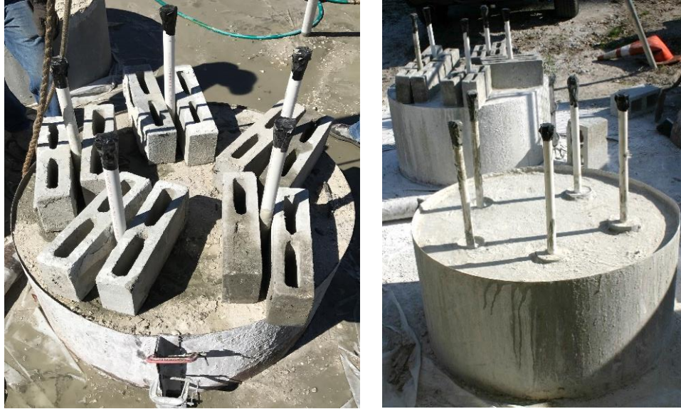
Figure 3.17 Rock socket specimens after concreting (left), ready for load testing (right).
