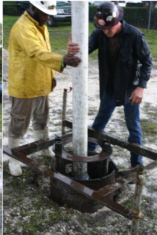
Figure 4.13 Concreting: control shaft (left) and temporary cased shaft (right).
