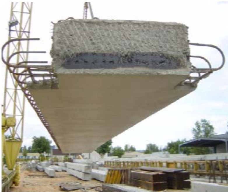
Figure 1. Poutre-Dalle System (Ralls et al., 2005)
