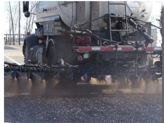
Figure 1 Tack coat truck spraying emulsion
