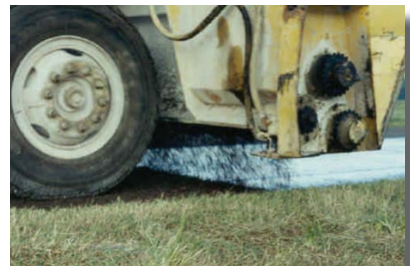
Figure 2 Truck spreading aggregate on top of emulsion
