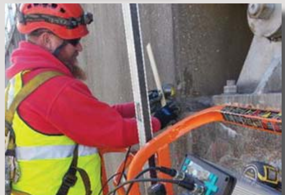
Figure 2 (bottom): FDH operator performing UT measurements
