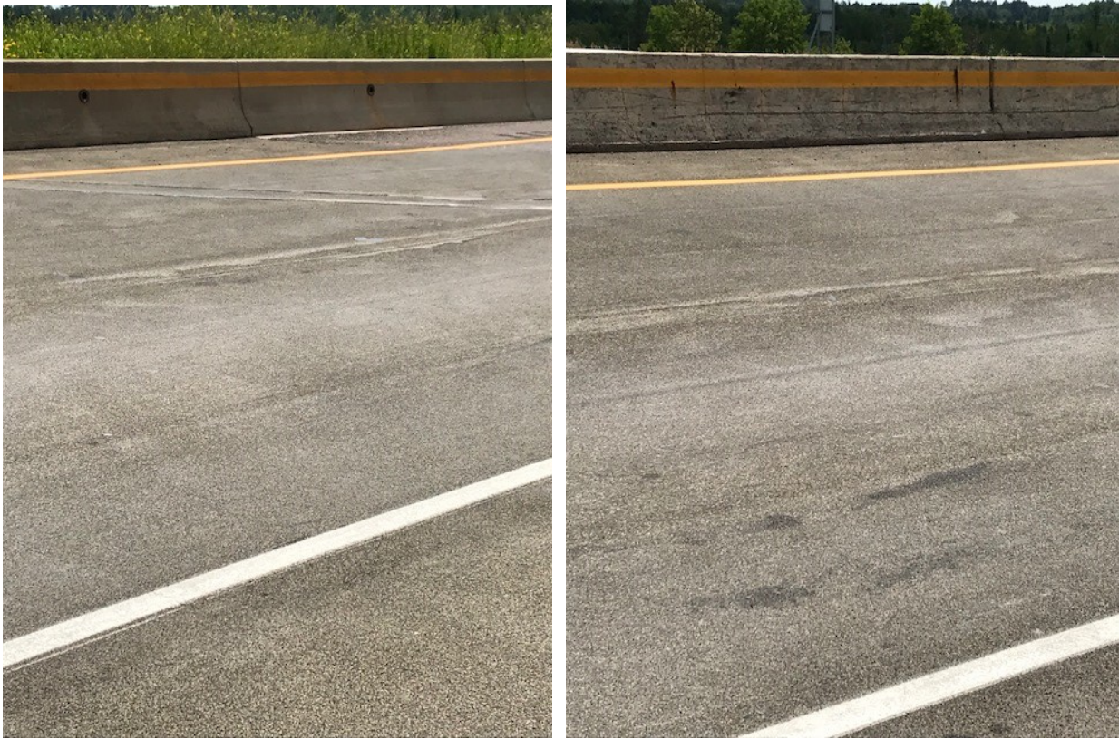
Figure D.3.24: Photos of TPO surface taken July 2018.
