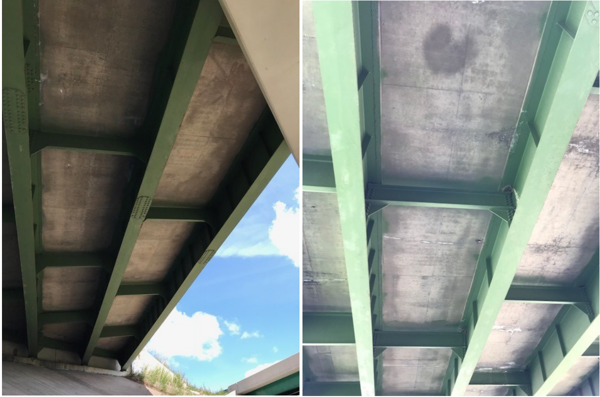
Figure D.3.25: Photos of deck underside (1965 deck) taken in July 2018.
