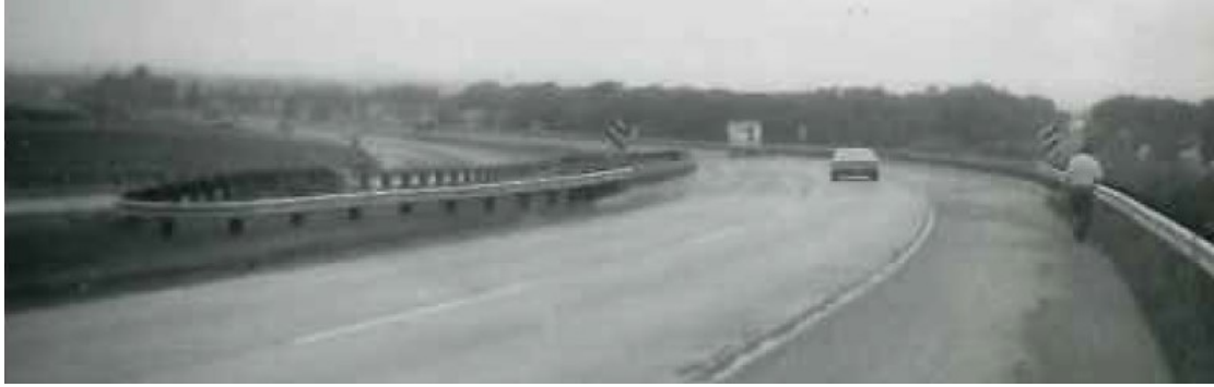
Figure 6.4 Bridge 69006 near Virginia, MN, in 1972 looking northwest.
