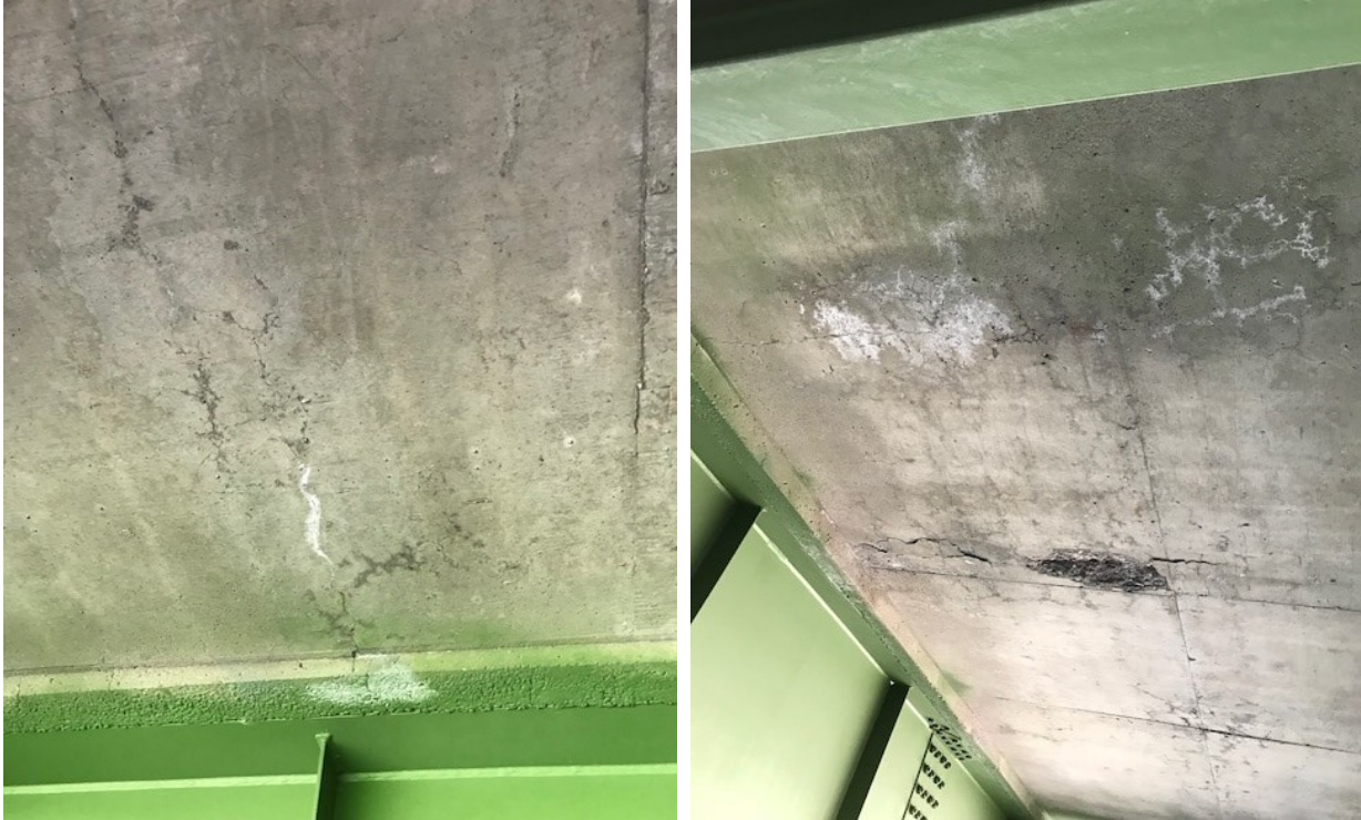
Figure D.3.26: Photos of deck underside (1965 deck) taken in July 2018.
