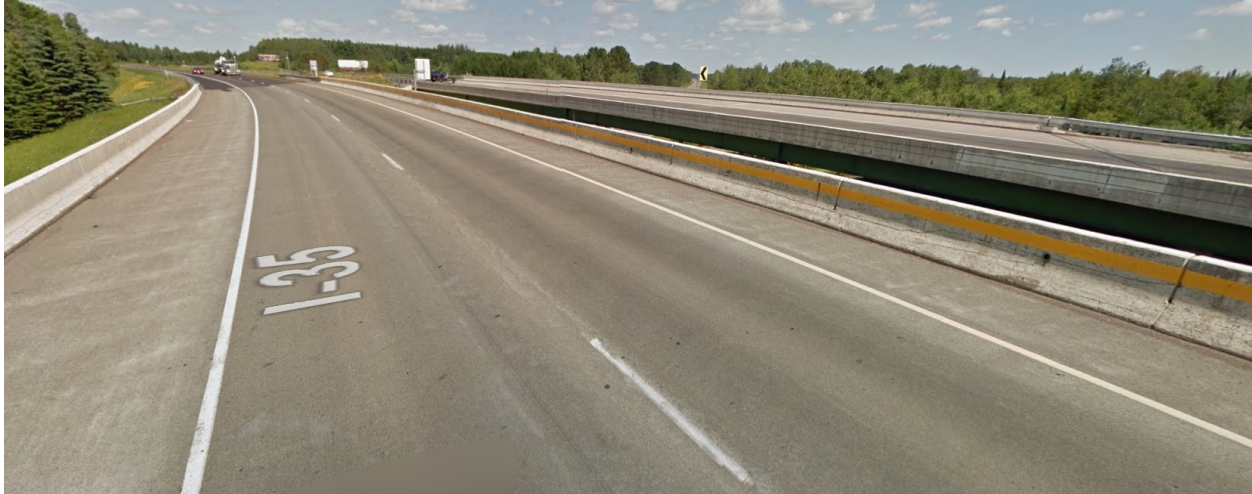
Figure D.3.3: Bridge deck photo from August 2014 (Obtained from Google Streetview)
