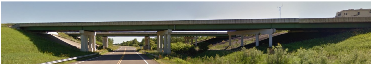
Figure D.3.2: Bridge Elevation from west
