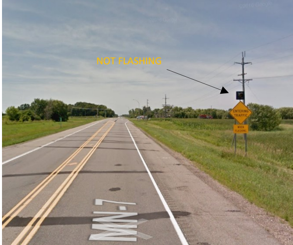
Not active (© 2017 Google from Google Street View)
