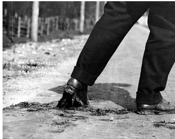
**Figure 1.2. Example of Early Unstable Asphalt Mixture (circa 1912) (Mahoney 2002).**
