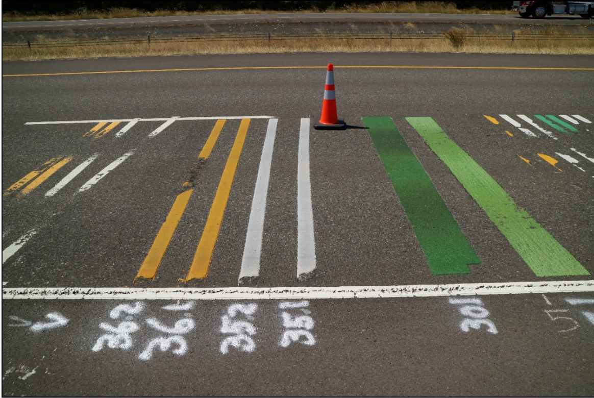
Figure 10.1: Example section of the longitudinal stripe with cracks measured in repeatability test.
