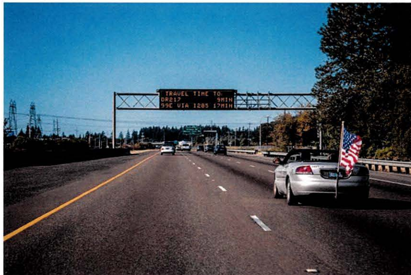
Figure 2.10. Interstate 5 (Image Source: Randy McCourt)
