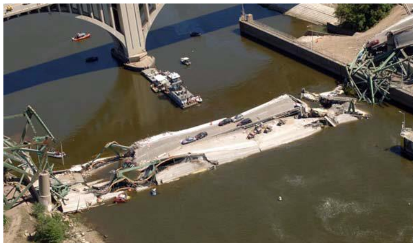
Figure 2.1 Collapsed I-35W bridge section [1]
