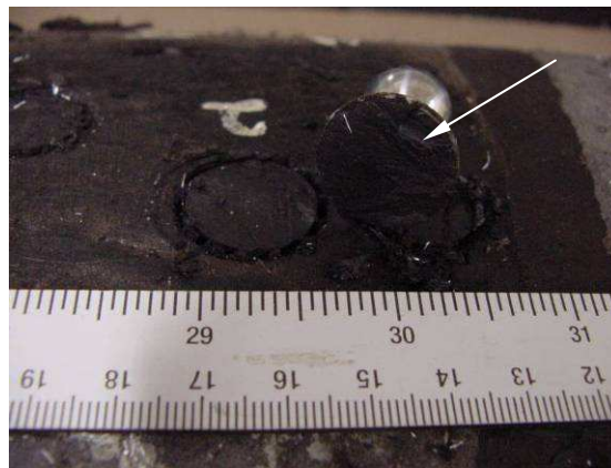
Figure 10. Typical appearance of coal tar coating showing cohesive failure.
