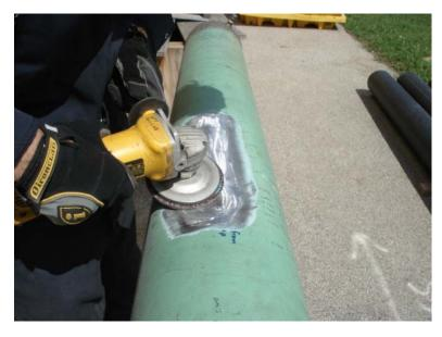
Figure 19 - Grinding the pipe surface for the inspection of cracks
