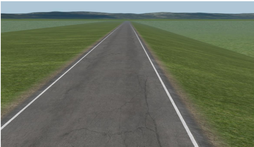
Figure 12. Straight road with a 3:1 side-slope.
