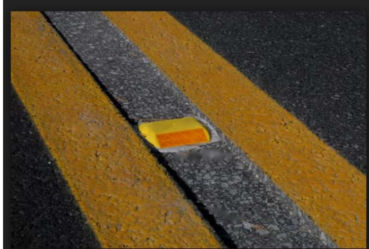
Figure 3: Recessed Snowplowable Pavement Marker
