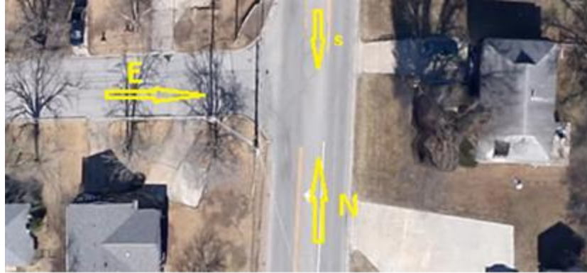
(a) Aerial view (Google 2016)
