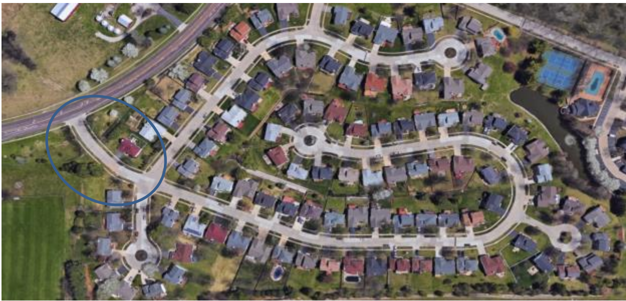
Figure 6.4 Residential driveway at an urban arterial (Google Earth 2016)
