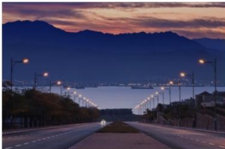
Figure 6.11. Illumination on both sides of the road
