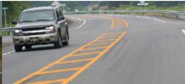
(f) Flush paved median
