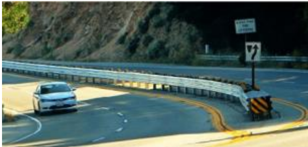
(c) Median W-beam barrier
