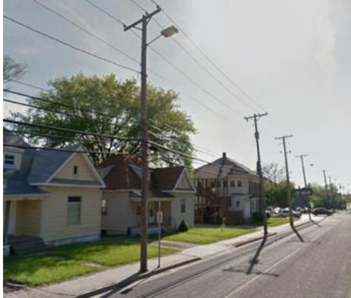
Figure 6.10. Utility posts on side of the road
