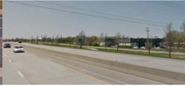
(b) Median concrete barrier
