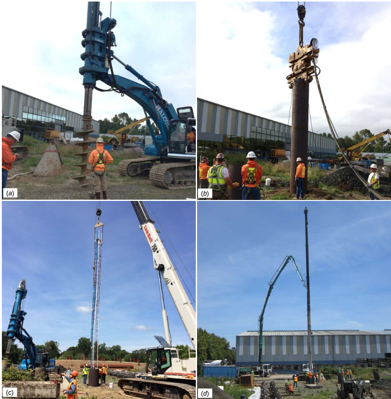
Figure 5.4: Construction of the cased shafts: (a) drilling a hole, (b) vibrating steel casing into the hole, (c) lowering the steel cage for CNIR, and (d) placing the concrete.
