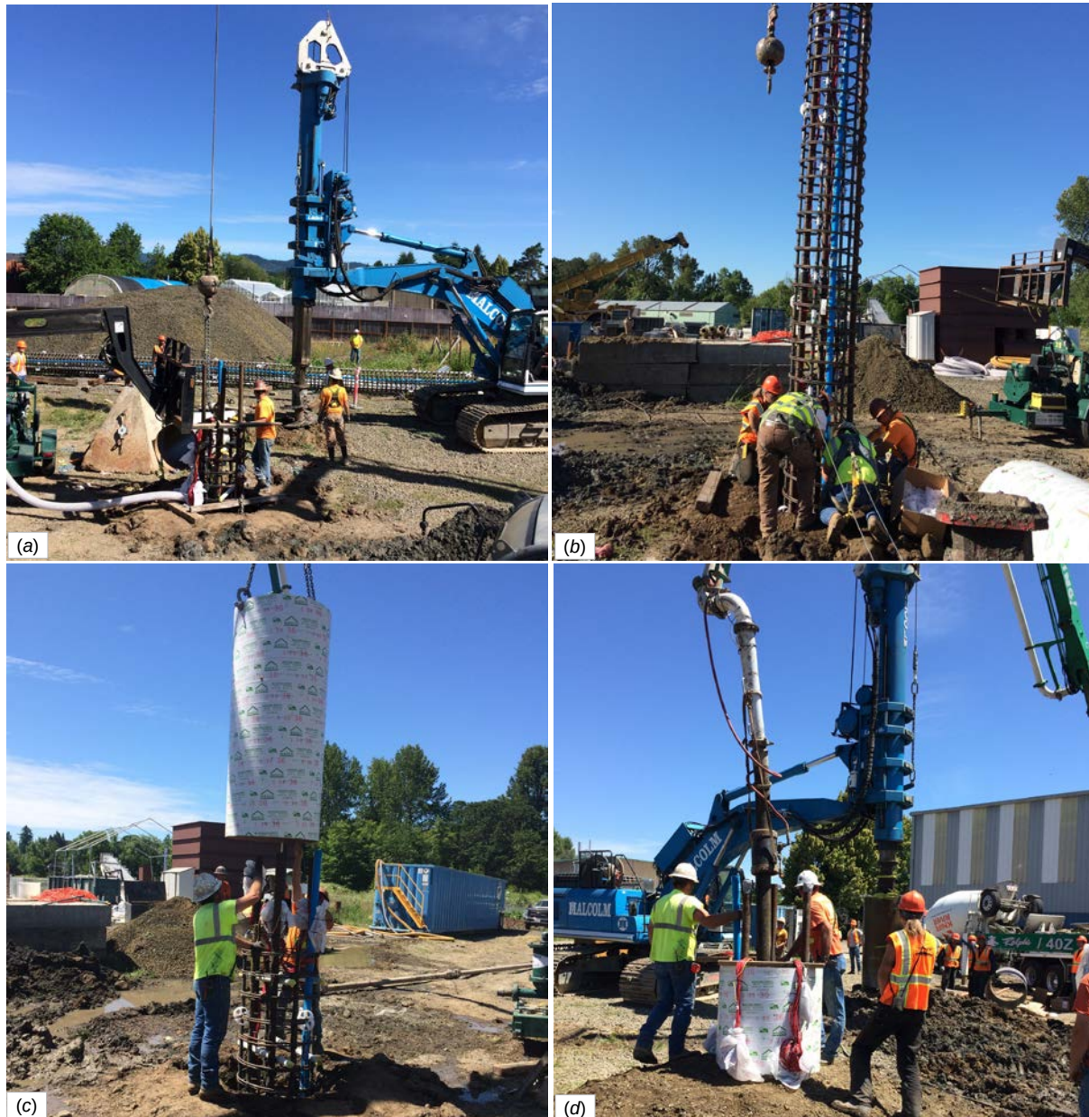
Figure 5.3: Construction of the uncased shafts: (a) drilling a hole, (b) lowering the steel cage into the hole, (c) installing sonotube concrete form, and (d) placing the concrete.
