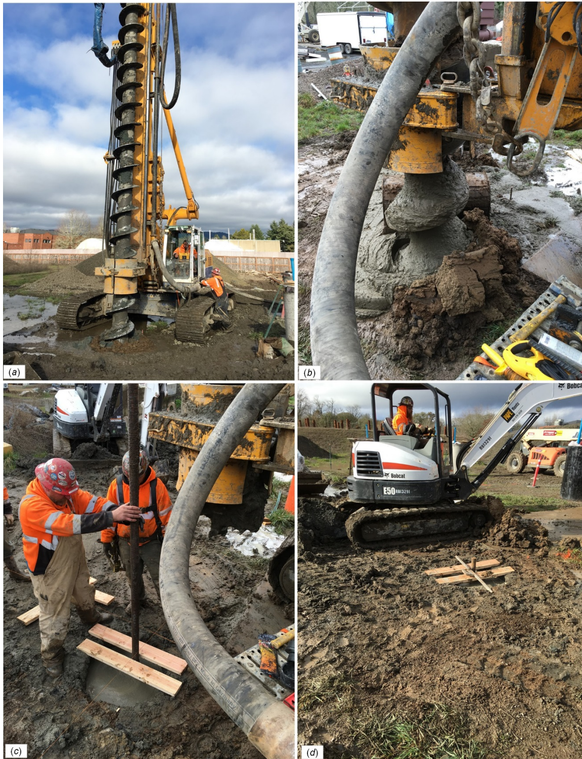
Figure 5.5: Construction of the continuous flight auger piles: (a) drilling a hole, (b) simultaneously pumping of the concrete and withdrawing of the auger, (c) lowering the steel bar, and (d) supporting the steel bar.
