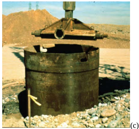
Figure 2.7 Use of (a) oscillator rig, (b) vibro-hammer, and (c) twister bar to advance casing (after Brown et al. 2010)
