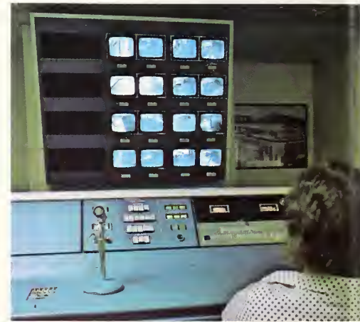
TV cameras located in each station provide the control room with a view of the passengers as they enter and leave the cars.
