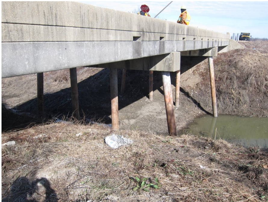
Figure 13: Route WW Bridge with CIP piles.
