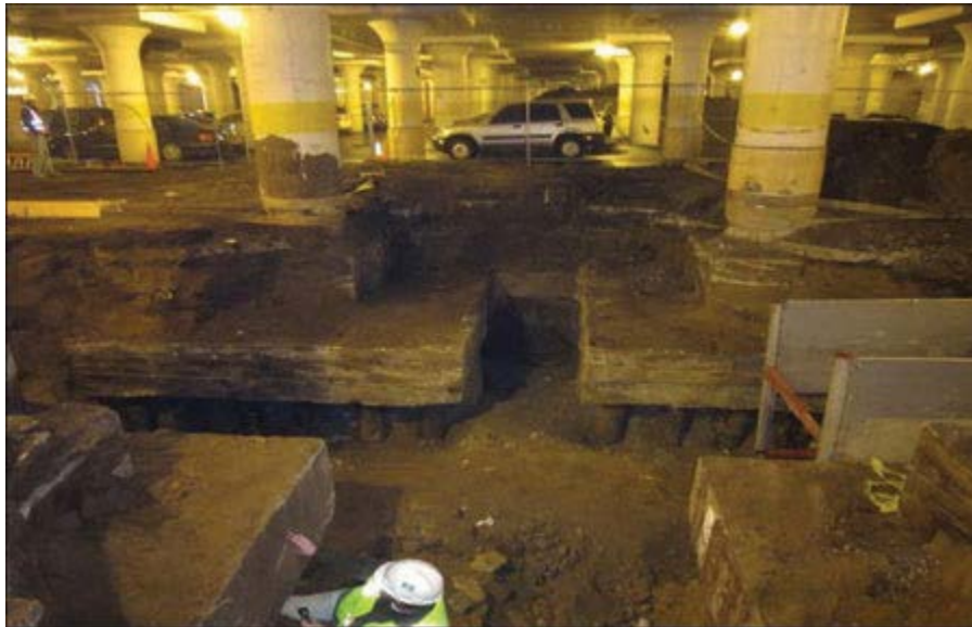
Figure 4: Test pit exposing timber piling. From Johnson and Chauvin (2013).
