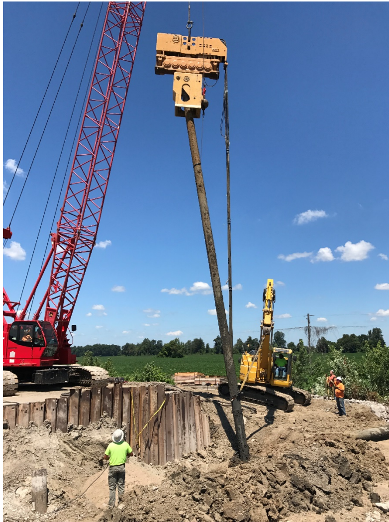
Figure 32: Pile exhumation at the Route WW site.
