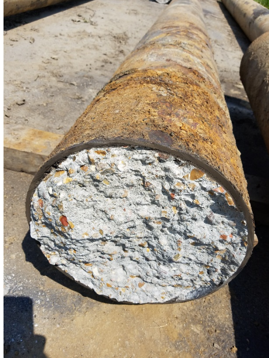
Figure 14: Concrete filled CIP pipe pile from the Route WW bridge site.
