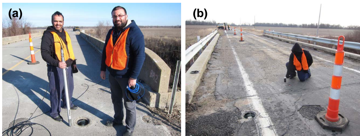
Figure 18: Parallel Seismic equipment used: (a) three-component downhole sensor (shown next to Borehole 2) and (2) instrumented sledge hammer (impacting over Pile 2 location).
