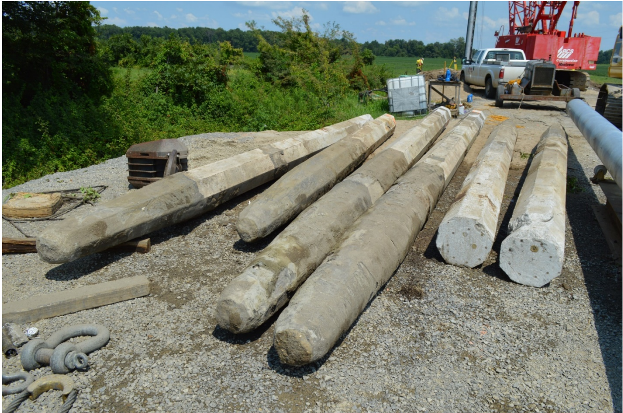
Figure 36: Exhumed precast piles.
