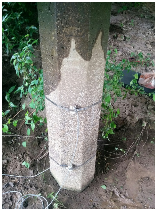
Figure 19: SE test setup on precast Pile 7 at the Route U site.
