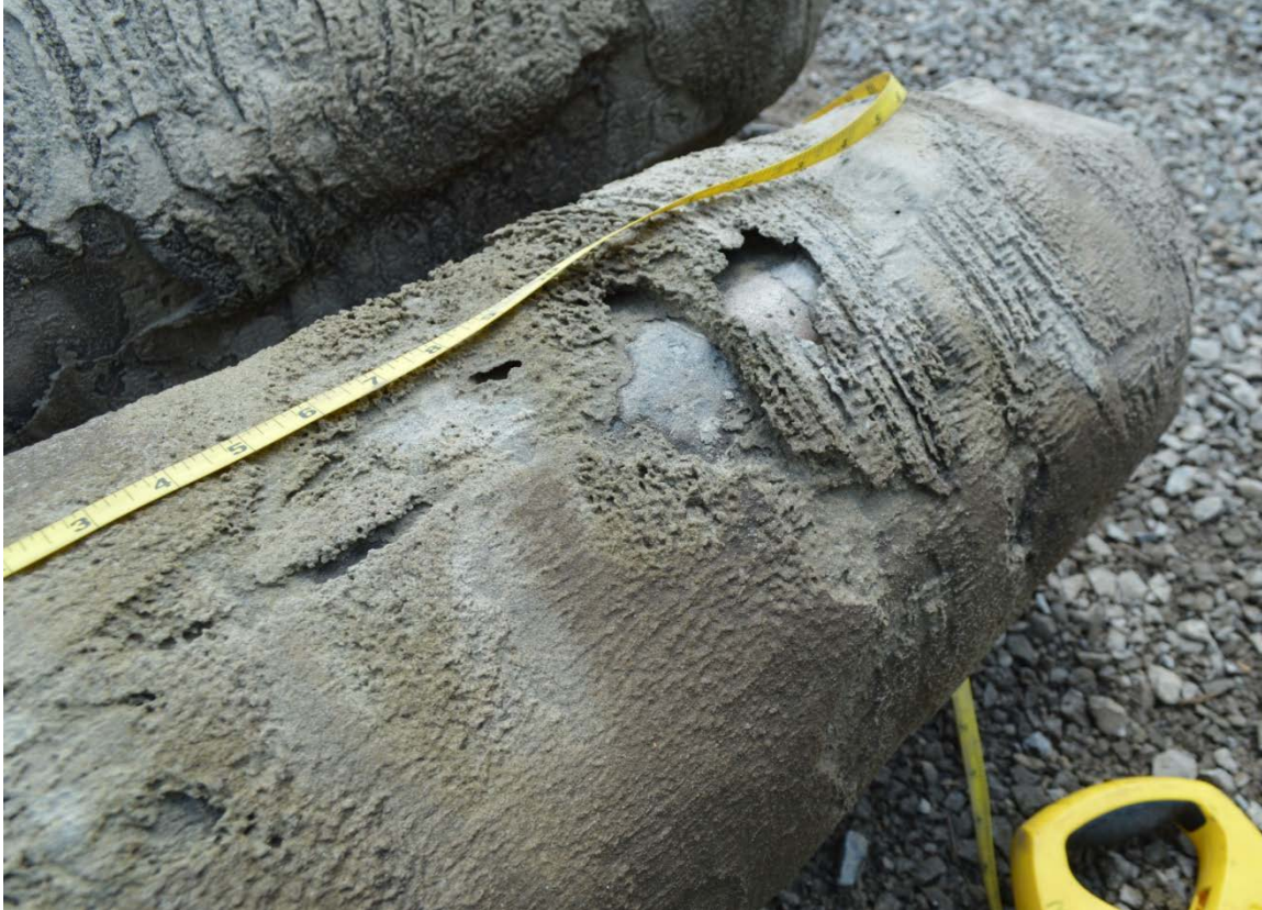
Figure 38: Close-up view of tip of exhumed precast pile showing sand adhered to pile surface.
