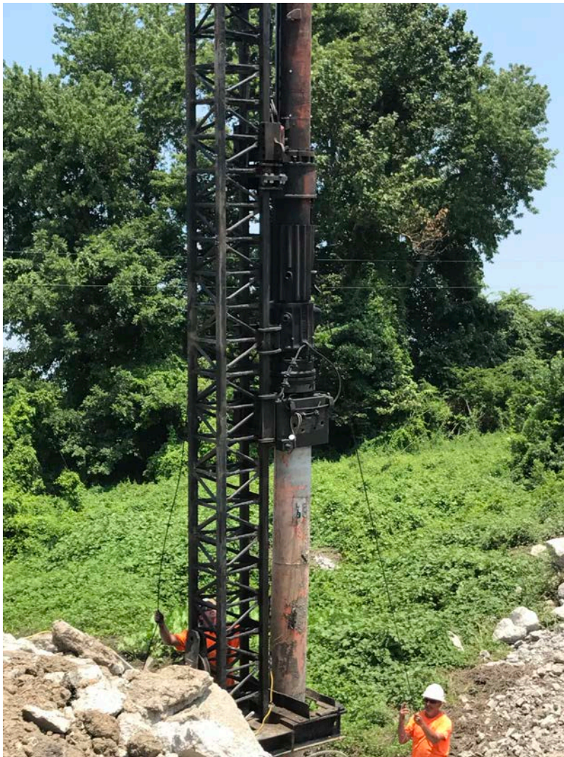
Figure 31: Restrike test of a CIP pile.
