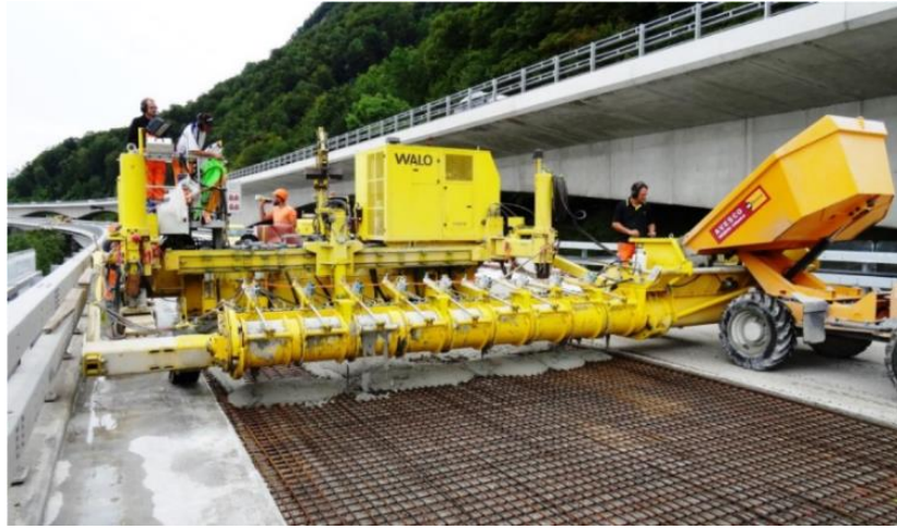
Figure 2-16 Implementation details of UHPC overlay application
