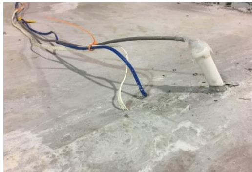
Figure 6-6 Embedded sensors of strain, temperature, and RH at each measurement location
