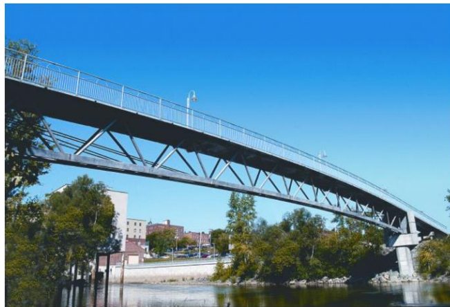
Figure 2-12 Sherbrooke pedestrian bridge (Russell and Graybeal, 2013)
