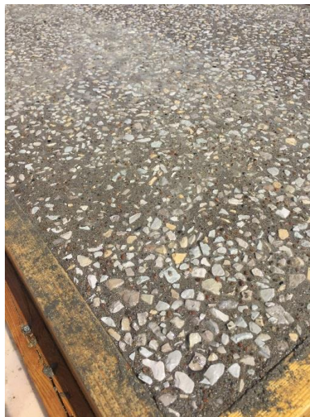
Figure 6-2 Substrate surface preparation
