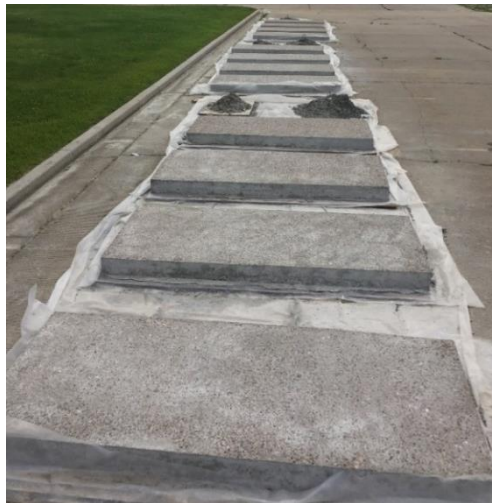
Figure 6-1 Concrete pavement sections as substrate
