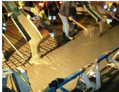
Figure 2-6 Cross-section (dimensions in cm) with UHPC layer (in grey) and view of UHPC casting performed (Bruhwiler and Denarie, 2008)
