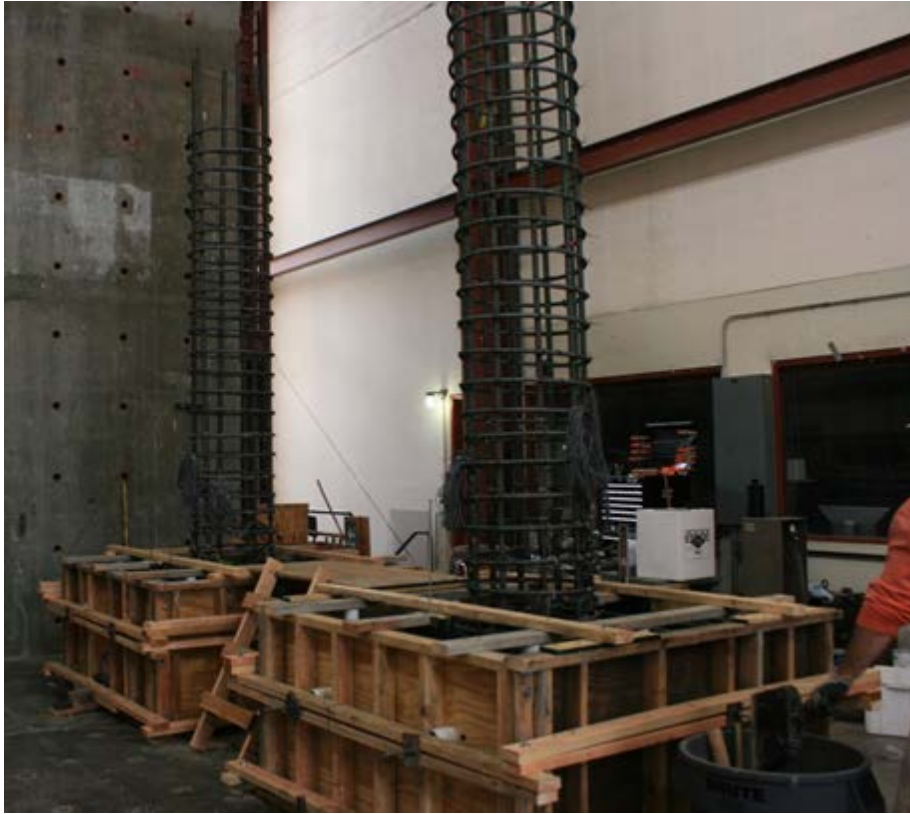
Figure 2.19 - Assembled forms for casting of footings
