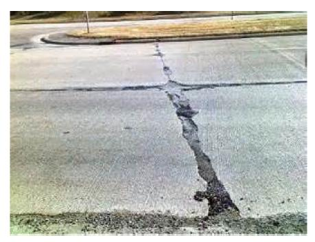
Figure 6.7. Spalling Along a Longitudinal Joint (Photo from [93]) *Spalling* - cracking, breaking, chipping, or fraying of the concrete slab surface within 2 ft. of a joint or crack.
