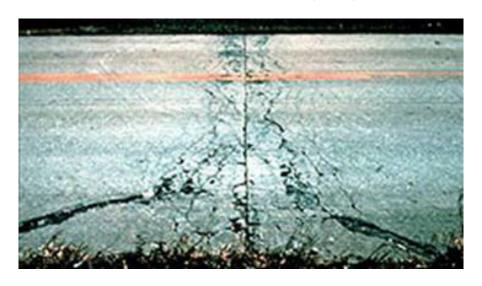
Figure 6.6. Moderate Severity Durability "D" Cracking (Photo from [92])
