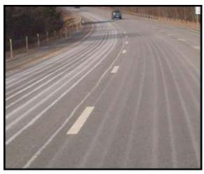
Figure 5: Pavement Pre-Treated with Sodium Chloride Brine Solution
