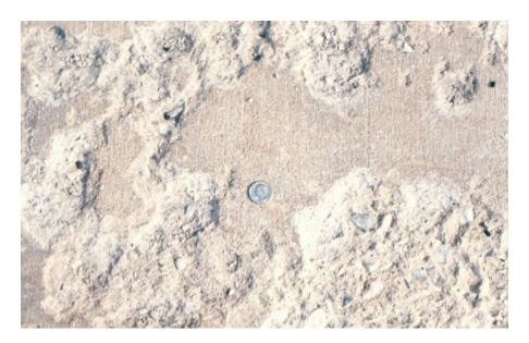
FIGURE 6.4. PORTLAND CEMENT CONCRETE SURFACE SCALING (PHOTO FROM [92]) Surface Scaling – is local flaking or peeling away of the near surface portion (the upper 1/8 to ½ in.) of hardened concrete resulting in the loss of surface mortar.
