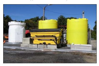
Figure 6: Brine Mixing (Sodium Chloride) and Storage (Sodium Chloride and Magnesium Chloride) Tanks, Putnam Garage
