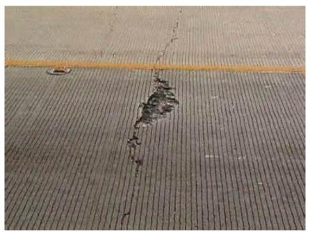
Figure 6.8. Delamination and Transverse Crack (Photo from [93])
