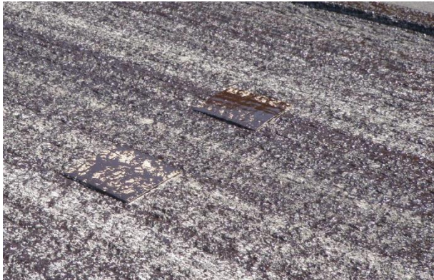
Figure 4.4 Inadequate Tack
