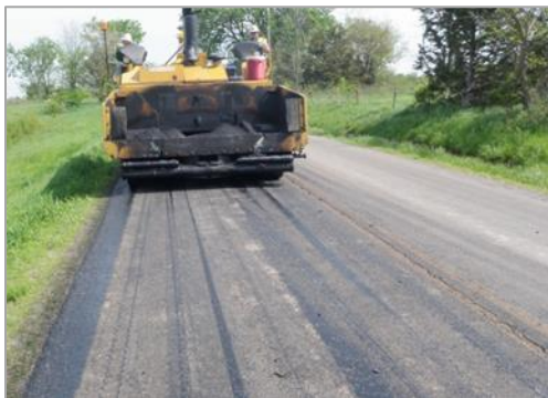
Figure 4.2 Tack Tracking Off Roadway
