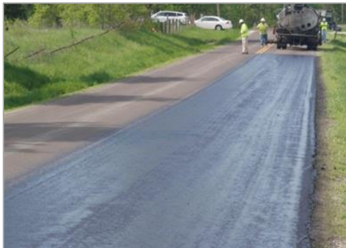
Figure 4.1 0.06 gal/yd 2 Tack Coverage
