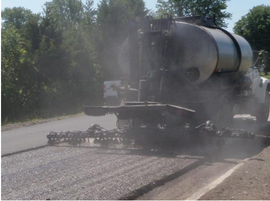
Figure 4.5 Inconsistent Spray
