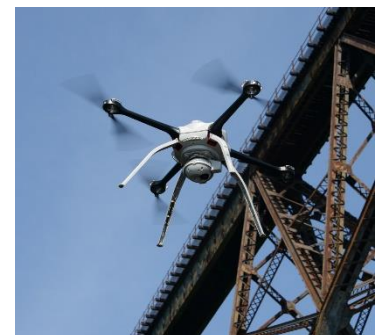
Figure 7. UAS Bridge Inspection
