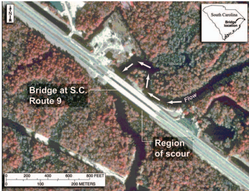
Figure 80. Severe meander on the Waccamaw River at Structure 264000920500 on S.C. Route 9 in Horry County, South Carolina. (Photograph from South Carolina DOQQ Archive, 1994.)
