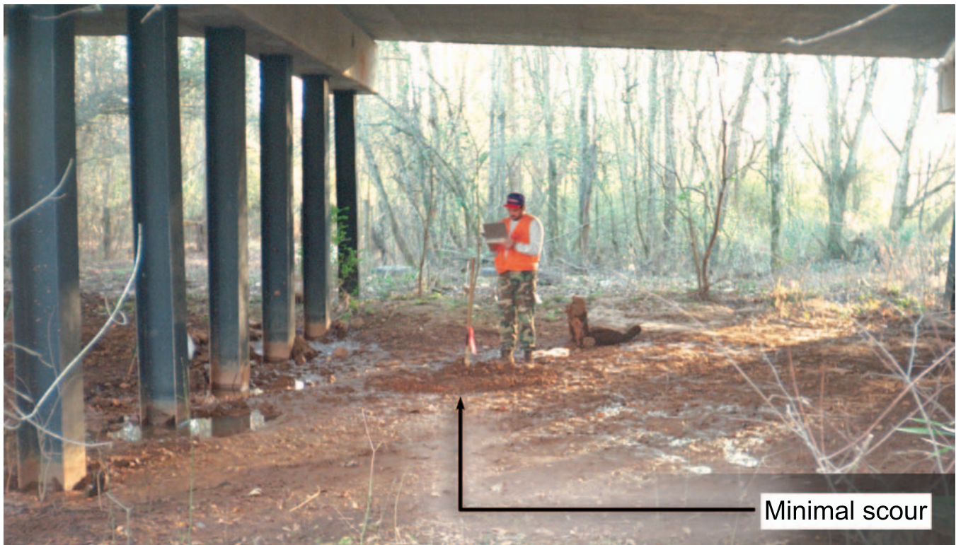
Figure 13. Example of minimal scour in the clayey soils of the Piedmont at Structure 047026300100 on Road S-263, crossing the Rocky River in Anderson County, South Carolina. (Photograph by the South Carolina District, U.S. Geological Survey, 1997.)
