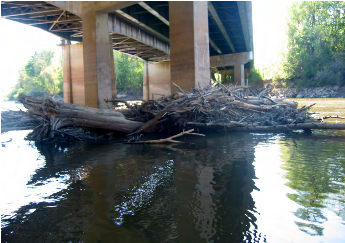
Figure 79. Examples of debris accumulation that can increase scour potential at (A) structure 367004500100 on Road S-45 crossing the Enoree River in Newberry County, South Carolina (March 8, 2005), and (B) structure 342007620100 on U.S. Route 76 crossing the Great Pee Dee River in Marion County, South Carolina (April 11, 2006). (Photography by the U.S. Geological Survey, South Carolina Water Science Center.)
