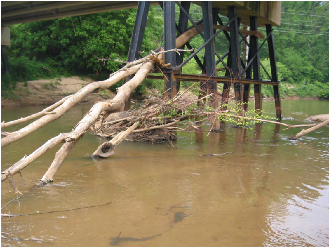
Figure 78. Examples of debris accumulation that can increase scour potential at (A) structure 307011200100 on Road S-112 crossing the Enoree River in Laurens County, South Carolina (October 9, 2002), and (B) structure 307026300100 on Road S-263 crossing the Enoree River in Laurens County, South Carolina (May 10, 2005). (Photography by the U.S. Geological Survey, South Carolina Water Science Center.)
