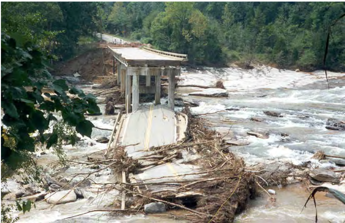
Figure 81. Failure of structure 304041800300 on S.C. Route 418 crossing the Enoree River in Laurens County, South Carolina (A) during the August 1995 flood (August 27, 1995), and (B) after the flood (September 1995). (Photography by the U.S. Geological Survey, South Carolina Water Science Center.)
