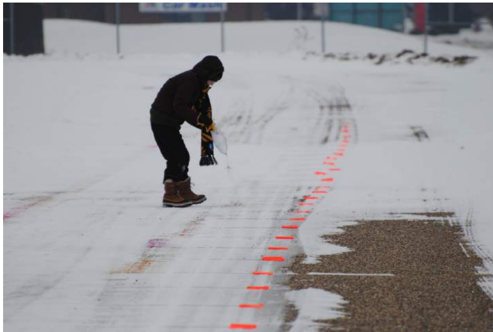
Figure 6 Distribution of deicer on marked areas: full lane width treatment (top); and compacted wheel track treatment (bottom).
