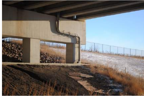
b) Down chute piping, outside lane.
