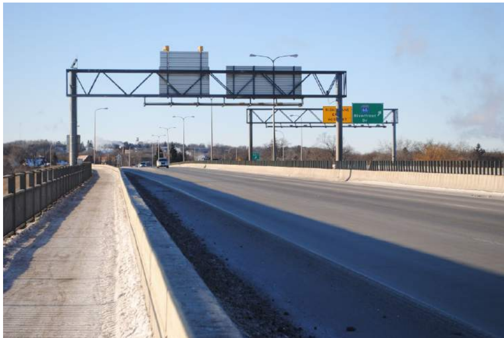
b) Northbound lanes, view south.
