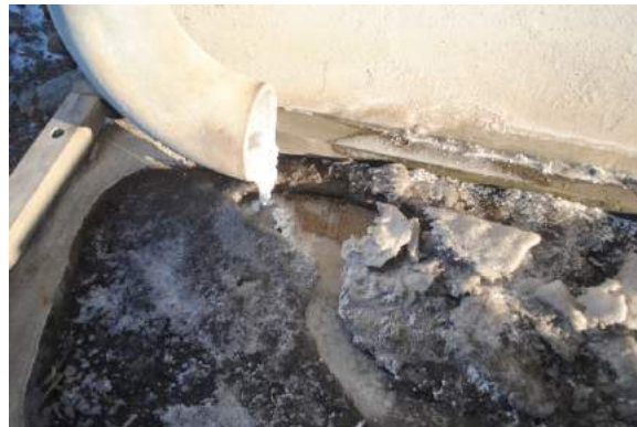
d) Outlet to concrete drainage gutter.
