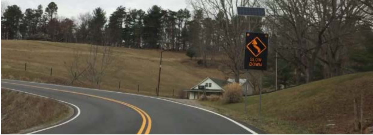
Figure 39. Curve 8.1 treatment – dynamic curve warning sign
