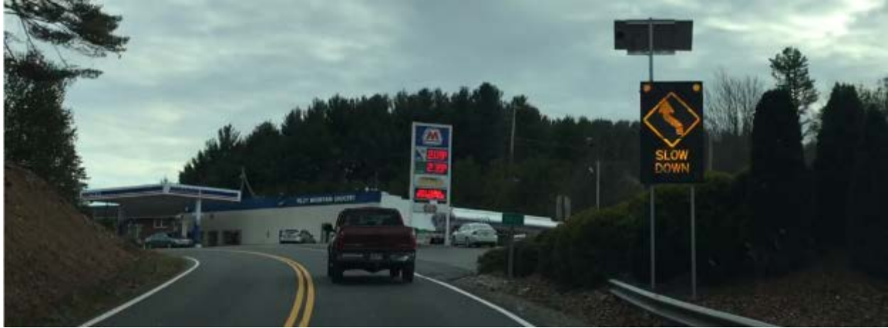
Figure 42. Curve 8.2 treatment – dynamic curve warning sign
