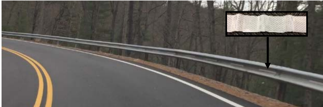
Figure 44. Curve 6 treatment – continuous reflectors
