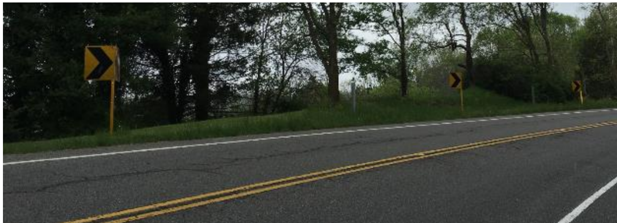
Figure 13. Curve 9 treatment – retroreflective chevron posts
