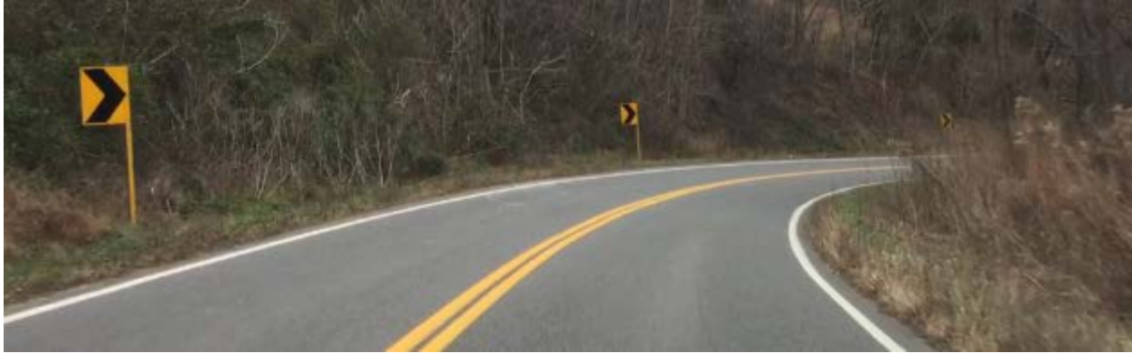
Figure 8. Curve 1 treatment – retroreflective material on chevron posts
