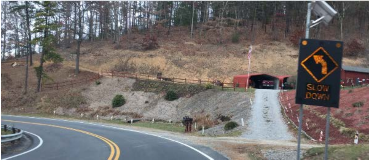
Figure 35. Curve 5 treatment – dynamic curve warning sign
