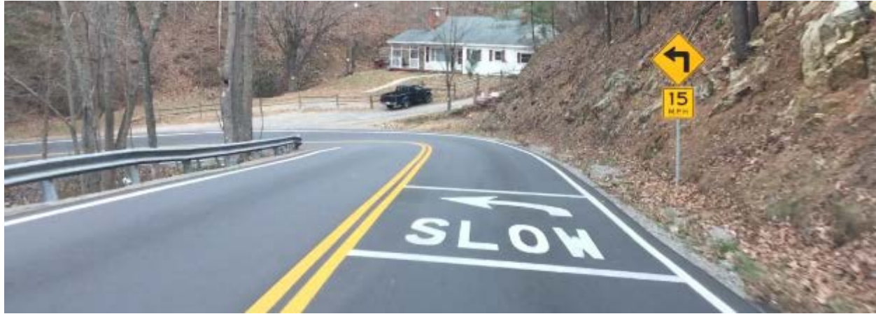
Figure 31. Curve 7 treatment – on-pavement signage
