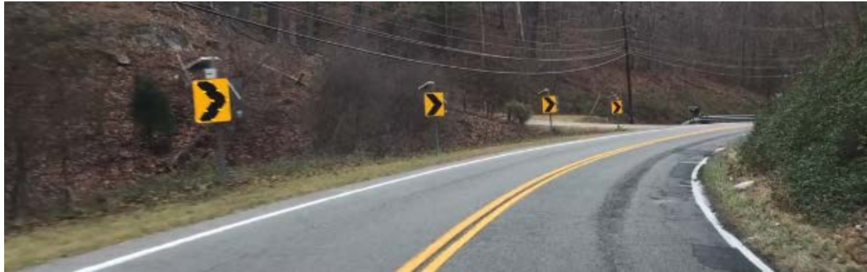
Figure 16. Curve 2 treatment – sequentially flashing chevrons
