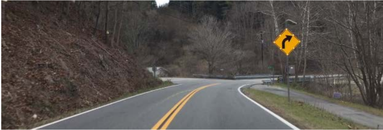
Figure 21. Curve 3 treatment – blinking curve warning sign
