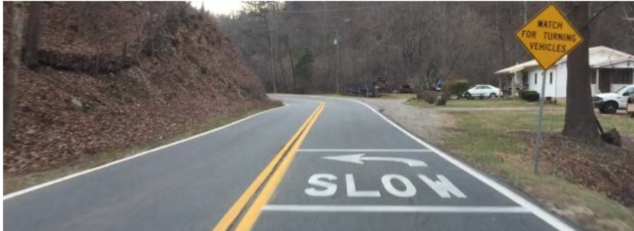
Figure 26. Curve 4 treatment – on-pavement signage
