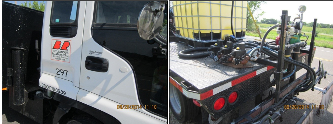
Figure 3.8 Installation of Biorestor® on Wright CSAH 75 shoulder.
