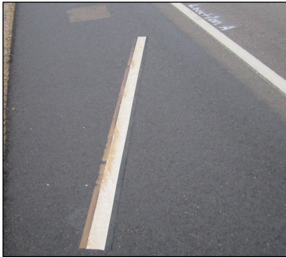
Figure 3.12 Test setup for monitoring retroreflectivity and application rate; Jointbond®.
