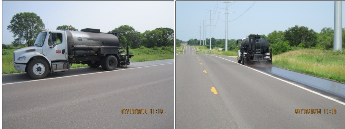
Figure 3.3 Installation of CSS-1h on Wright CSAH 75 shoulder.
