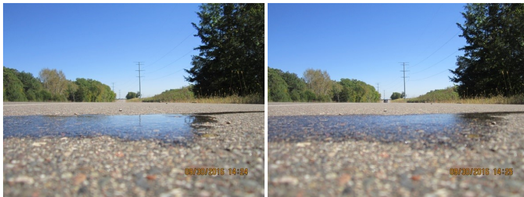
Figure 5.16 Ponded water soaking into surface texture (left, right).
