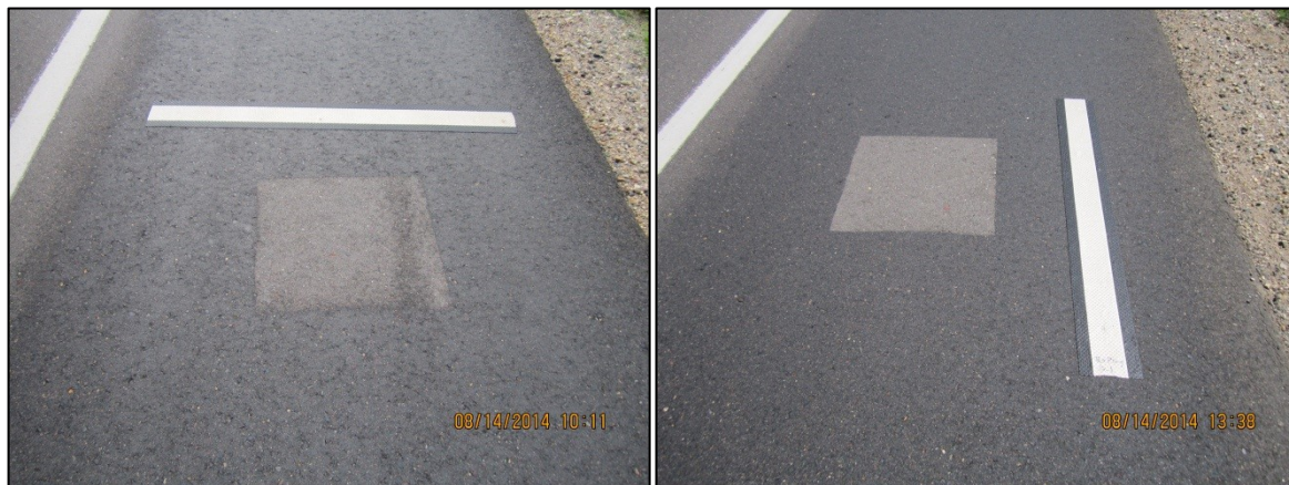
Figure 3.5 Test setup for monitoring retroreflectivity and application rate; RePlay™.
