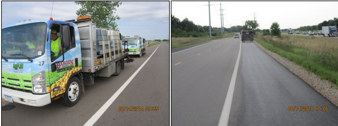
Figure 3.4 Installation of RePlay™ on Wright CSAH 75 shoulder.
