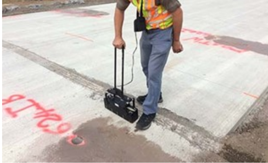
Figure 5.7 MIRA sweep being conducted adjacent to wheel rut in Cell 624.
