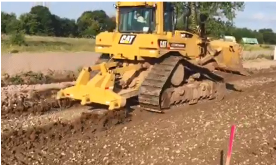
Figure 7.6 Subgrade conditioning with dozer and ripping teeth, MnROAD Cell 228.
