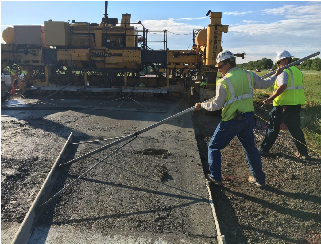
Figure 4.14 Contractor working on Cell 806 with 0.75 percent by volume fiber mix.
