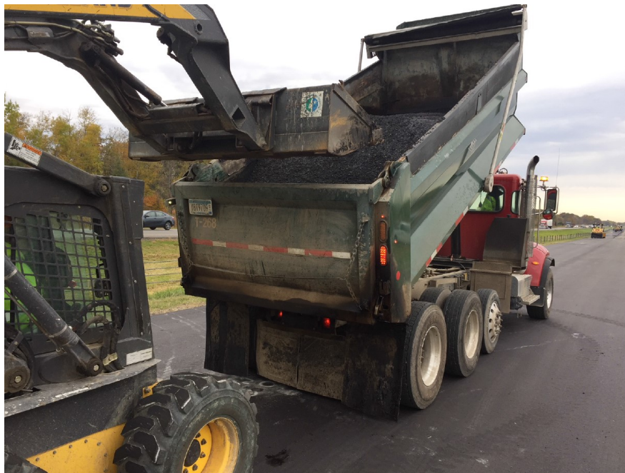
Figure 3.4 Bulk sampling approach for NRRA asphalt mixtures.
