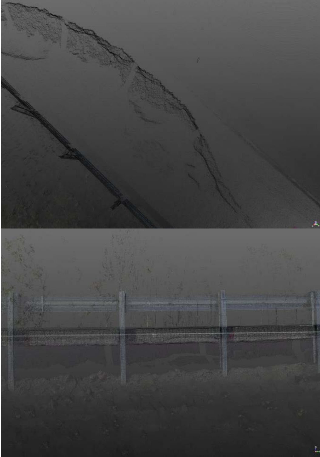
Figure 12. Route 251 Slope Failure – Shoulder Erosion, laser scanner generated point clouds with images superimposed.
