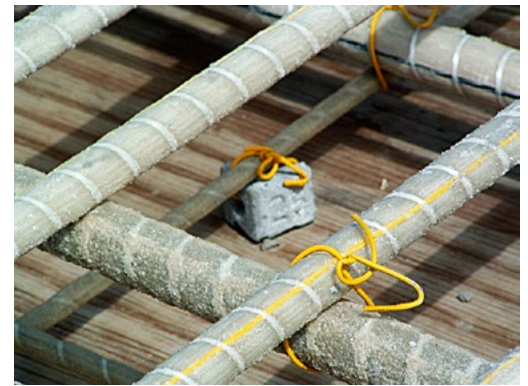
The fiber-based reinforcing bars shown here were developed through years of research and testing, and because they do not corrode, promise important benefits for the durability and reduced maintenance expense of the structure they will be part of.
