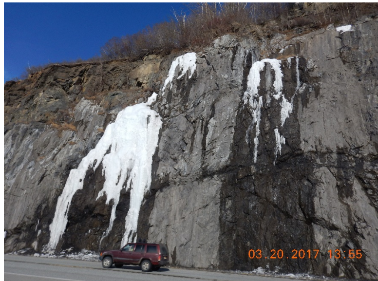
Figure 12 – Ice slab melting on dark colored rock near MP 113.2 NB on the Seward Highway (Photo by Scarptec, Inc.)
