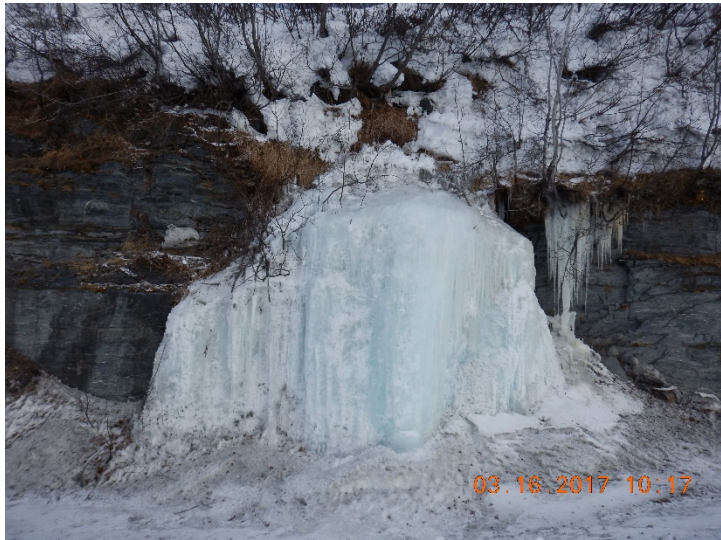
Figure 32 – Ice development near MP 23 SB along Richardson Highway (Photo by Scarptec, Inc.)
