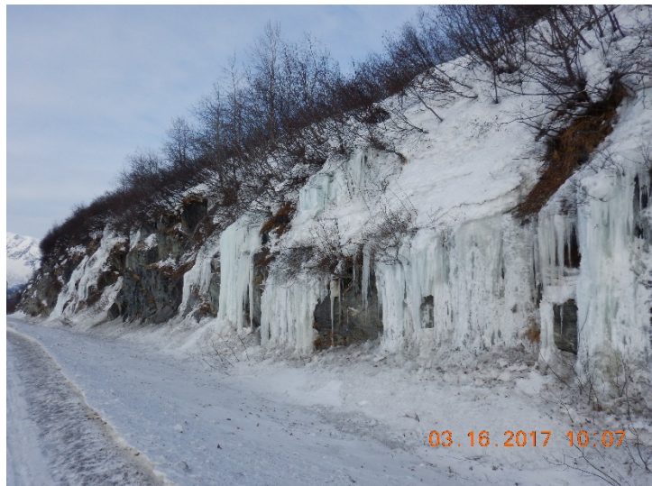
Figure 31 – Ice development near MP 22.9 SB along Richardson Highway (Photo by Scarptec, Inc.)
