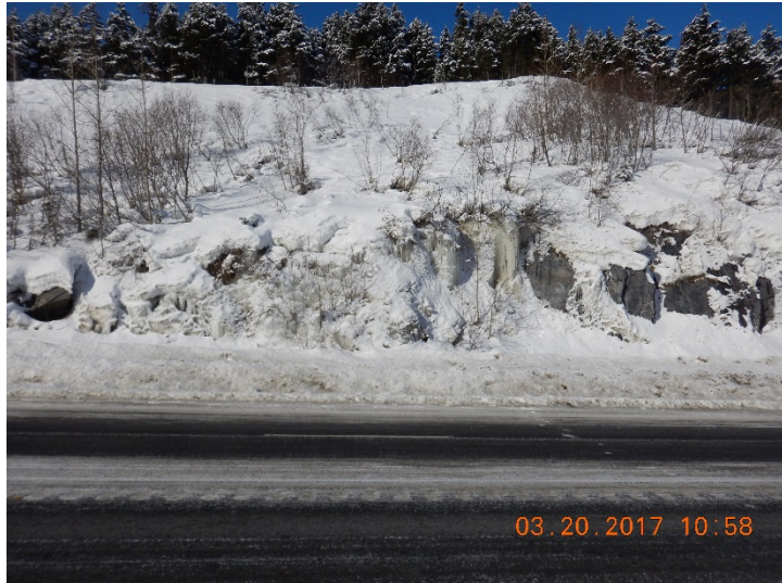
Figure 29 – Ice development near MP 52.3 SB along Seward Highway (Photo by Scarptec, Inc.)
