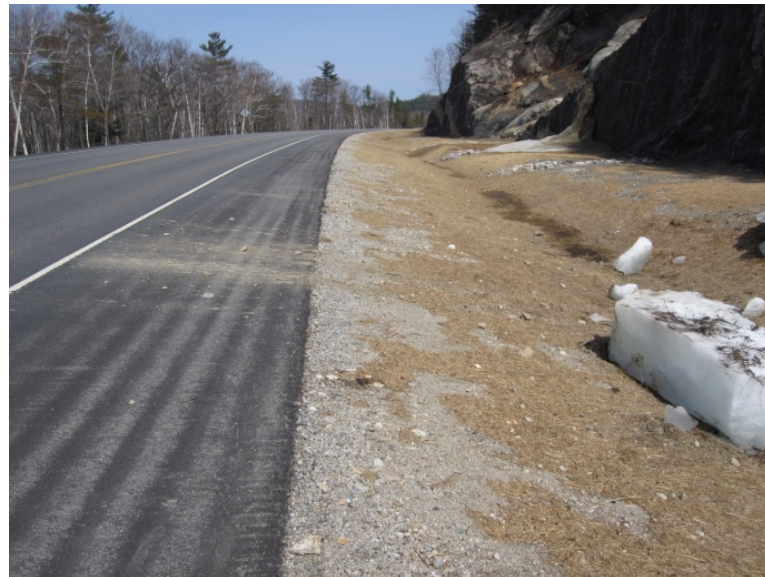
Figure 11 – Impact splatter from icefall impact in Gilead, Maine. Note mud and gravel in road. Photo adapted courtesy of Haley & Aldrich, Inc.
