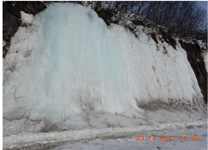
Figure 30 – Well-developed ice slab near MP 38.3 SB along Richardson Highway (Photo by Scarptec, Inc.)
