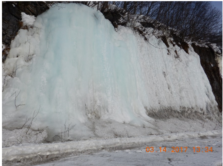
Figure 13 – Strong blue ice slab with adjacent weak white ice near MP 38.3 SB on Richardson Highway (Photo by Scarptec, Inc.)
