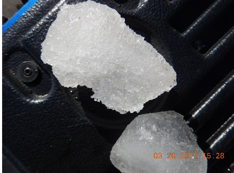
Figure 14 – Sample of fallen coarse-grained weak white ice from ditch at MP 113.2 NB on the Seward Highway (Photo by Scarptec, Inc.)
