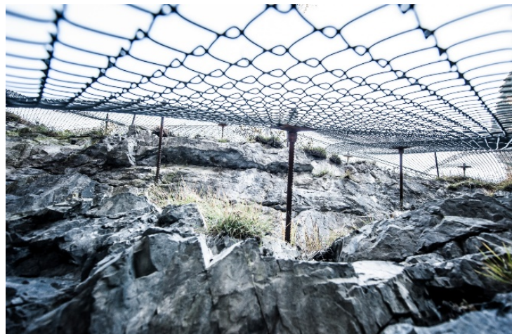
Figure 20 – Slotted icefall netting used in Austria (Photo by Trumer, Ltd.)
