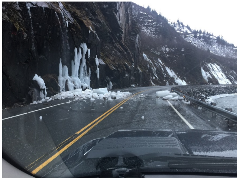
Figure 8 – Direct icefall impact & shatter at MP 13.9 Richardson Highway. Slab partially rotated outward during fall from overhung slope on 13 December 2017. Photo courtesy of AKDOT&PF.
