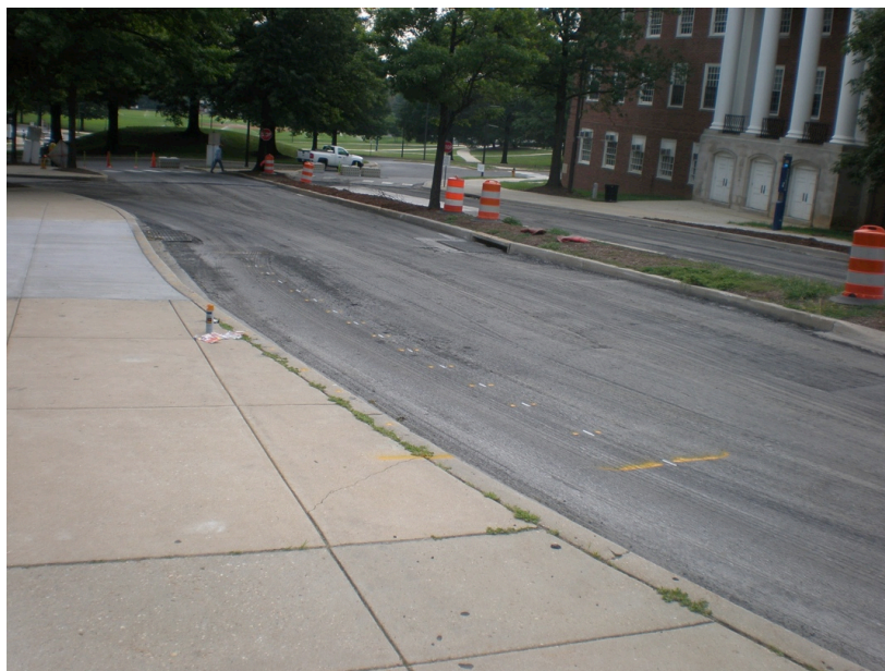
Figure 158. Photo. Encapsulated tags placed in the roadway prior to paving.
