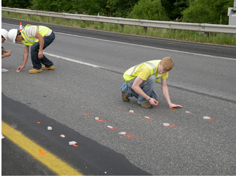
Figure 99. Photo. Placement of SAW RFID tags on surface of existing milled pavement.
