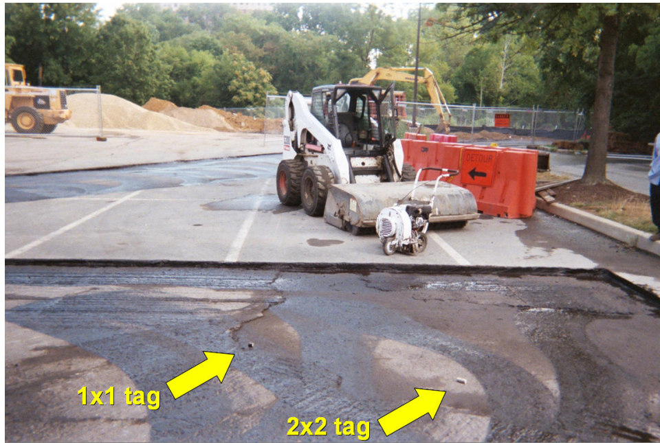
Figure 23. Photo. Pre-placement of tags at UMD Lot XX1 paving project.
