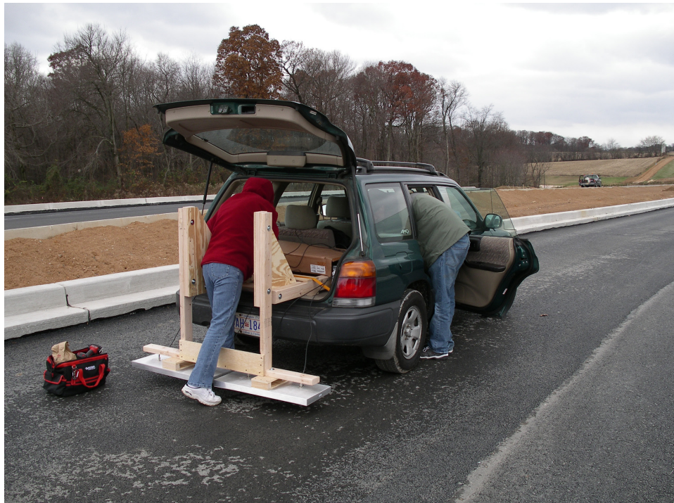
Figure 34. Photo. Vehicle-mounted antennae and RFID reader.
