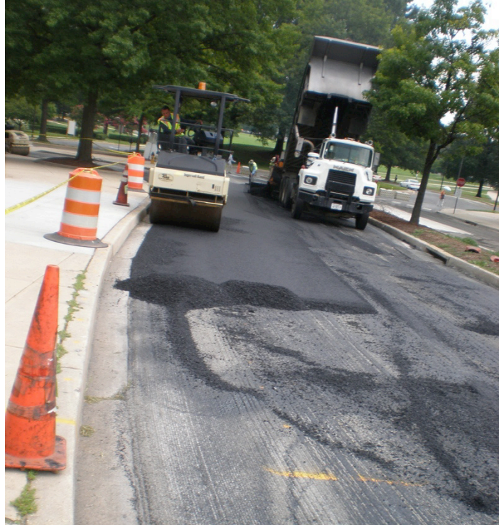
Figure 161. Photo. Paving in progress.
