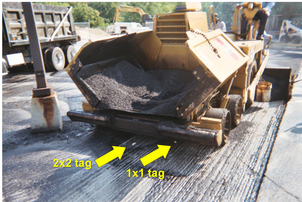
Figure 24. Photo. Paving over pre-placed encapsulated tags.
