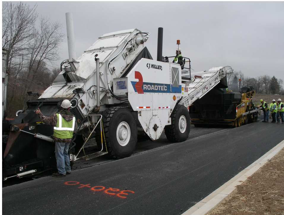
Figure 38. Photo. RoadTec® SB-2500D material transfer vehicle used in April 2008 paving at the Hampstead Bypass project.
