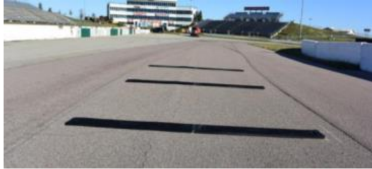
(a) Rumble Strip Layout – Viewed Longitudinally
