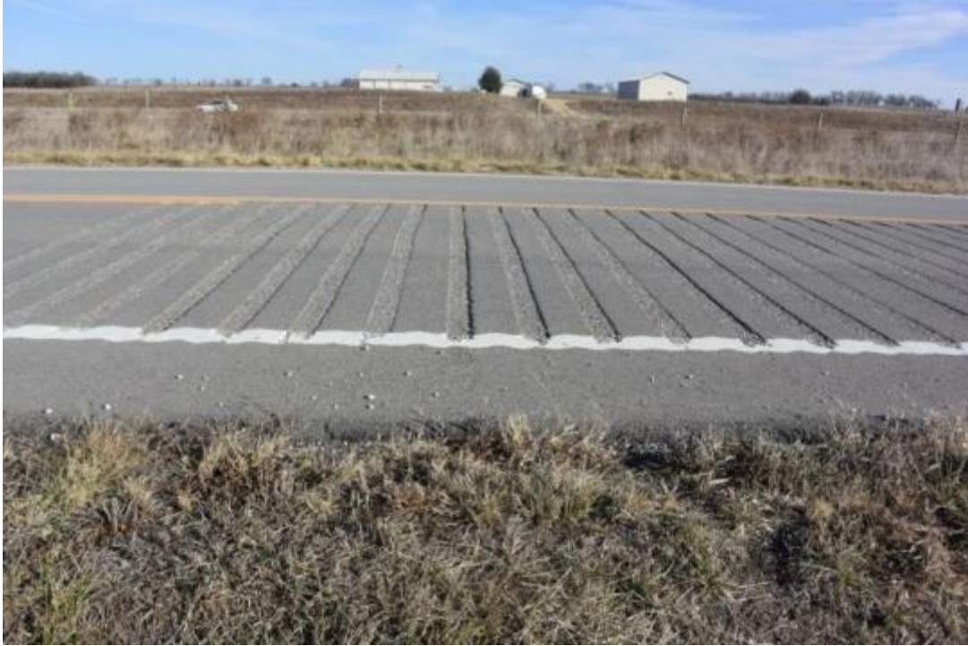
Figure C.7: CIP Strips on Southbound E 1250 Rd Near US-56
