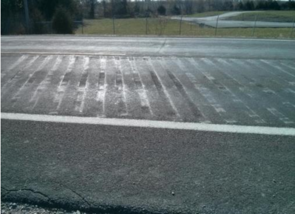
Figure C.3: CIP Strips on K-32 Near Intersection at K-32 and US-24/US-40
