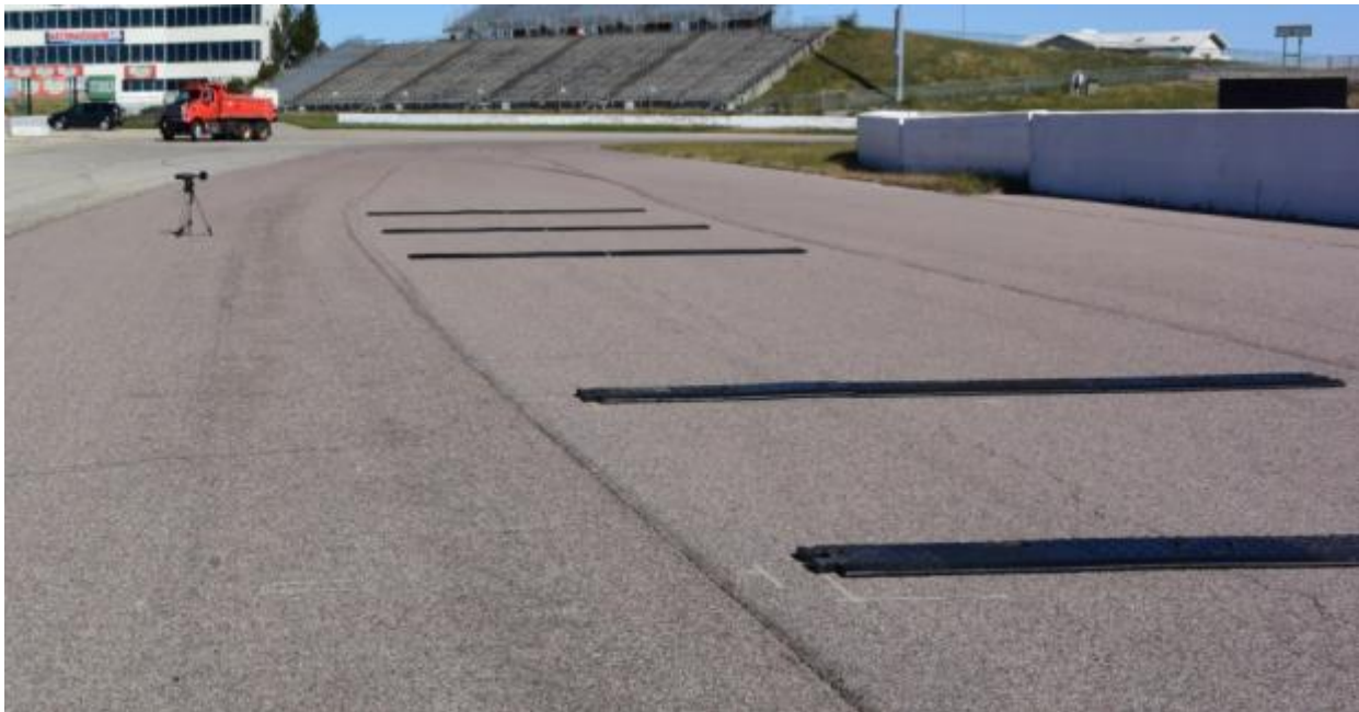
Figure 4.10: Arrangement of Sound Meter at Closed-Course Facility
