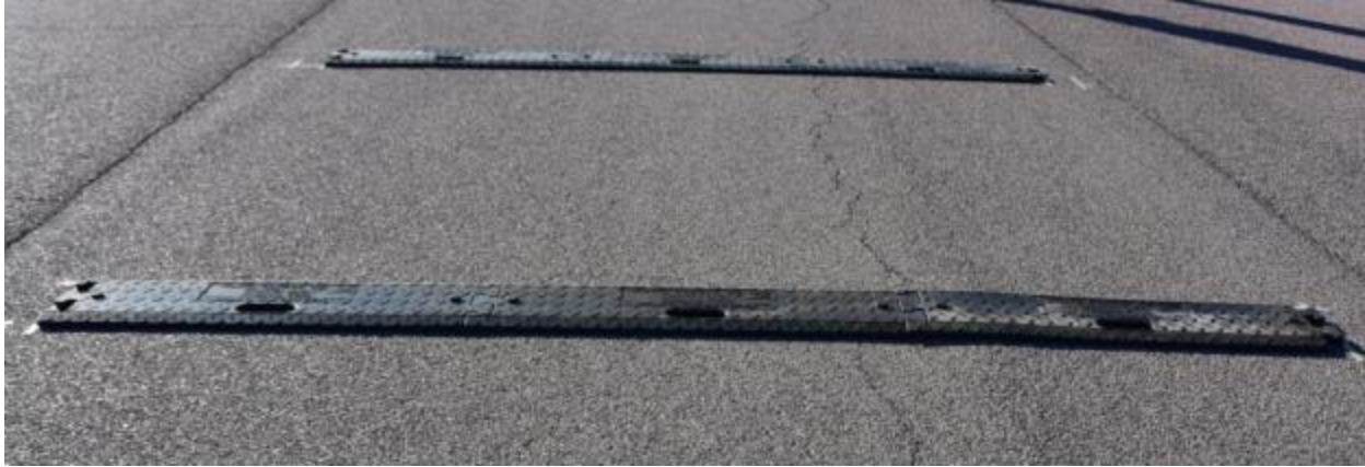
(a) Installed TrafFix Alert Rumble Strips
