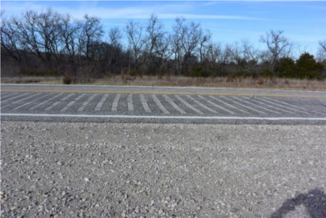
Figure C.6: CIP Strips on N 1150 Rd Near Intersection at N 1150 Rd and E 1000 Rd
