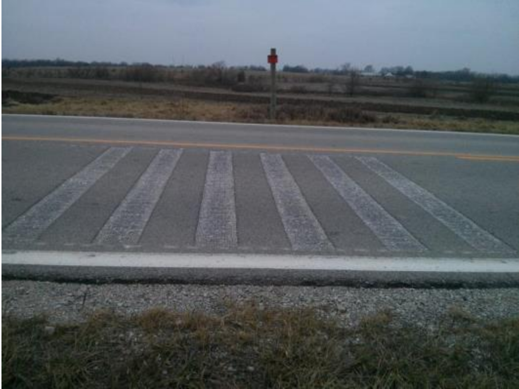
Figure C.5: CIP Strips on Southbound 1061 Near US-56
