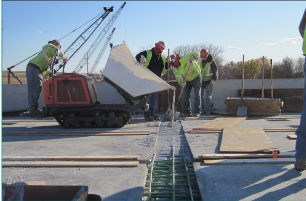
Figure 1. Field casting of grout in the connections between PBEs.
