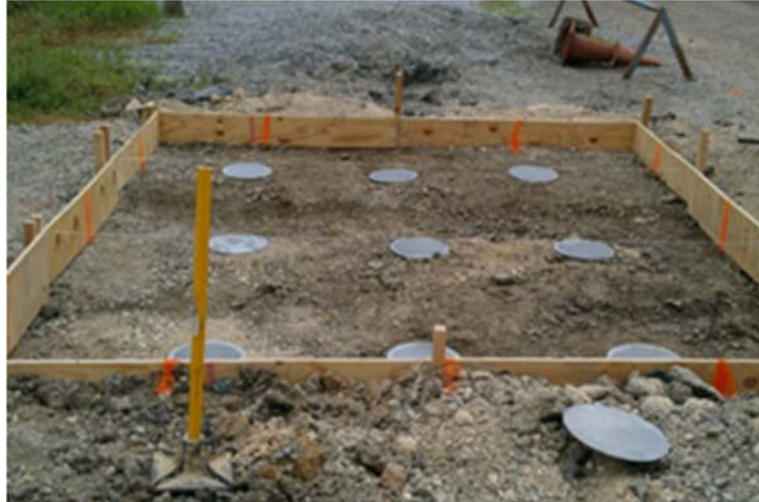
Figure 7 Plate layout for LTRC slab
