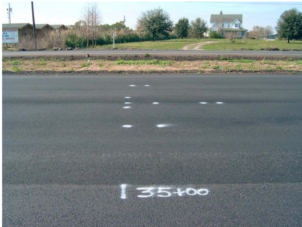
Figure 4 Coring for STA 35+00
