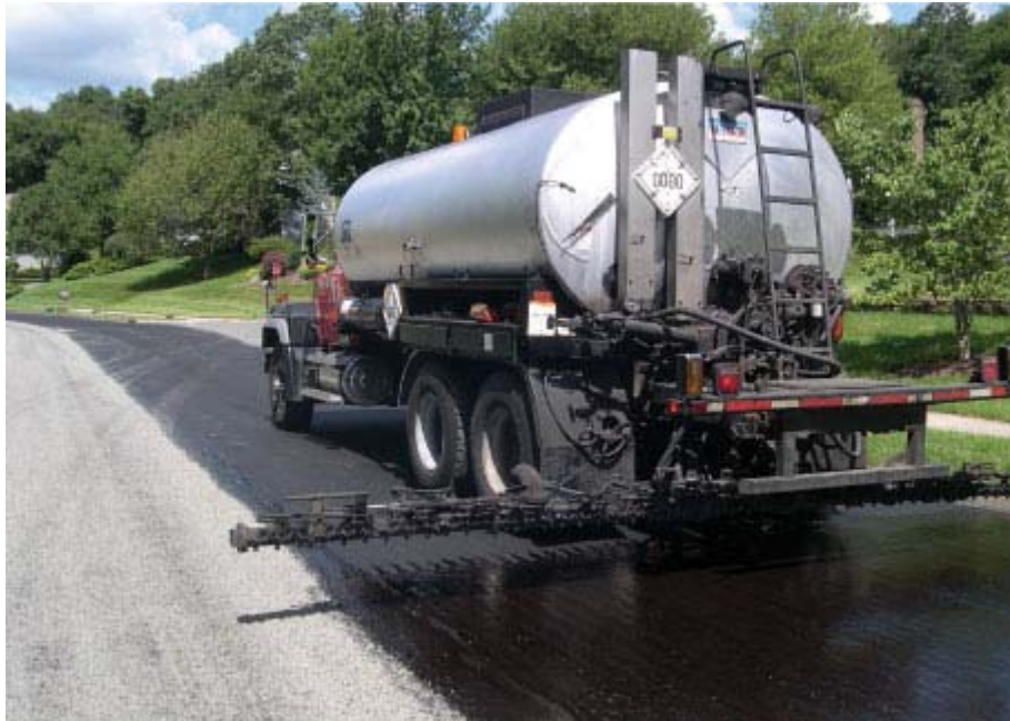
Figure 1 Typical application of tack coat
